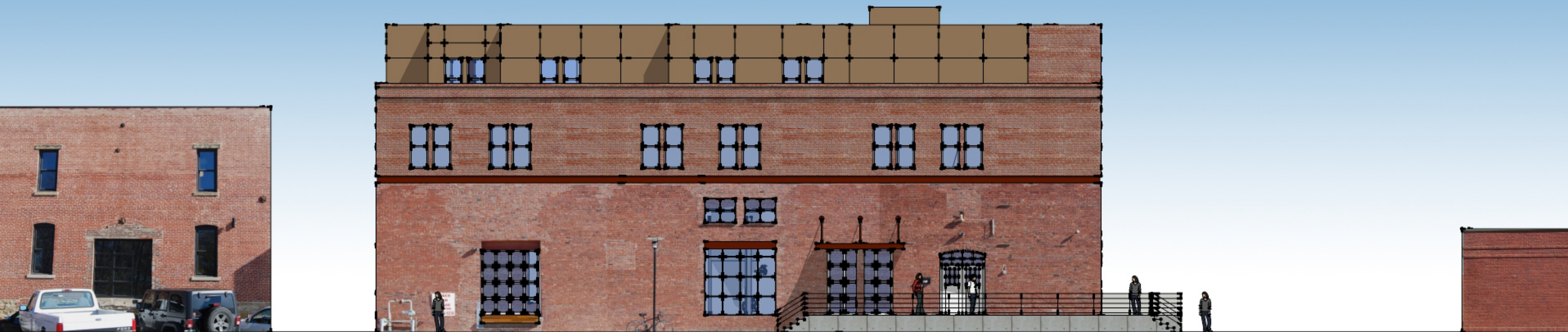
WEST ELEVATION, PENNSYLVANIA
