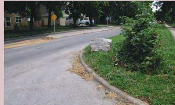
*Indeed, this is just a rock, but it was placed here to solve a critical problem: drivers had been cutting the corner, which damages the curbing and can be dangerous to others, especially people walking and biking. The rock is an inexpensive solution that fits just fine into the context.*
