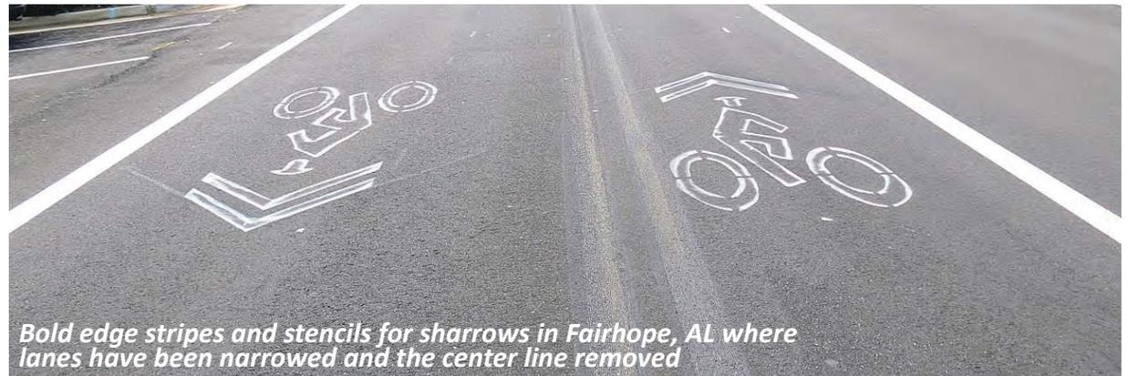
*Bold edge stripes and stencils for sharrow in Fairhope, AL where lanes have been narrowed and the center line removed*
