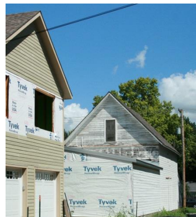
Barn During Rehabilitation
