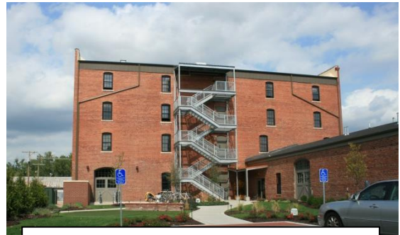
South View of Poehler Building Today
