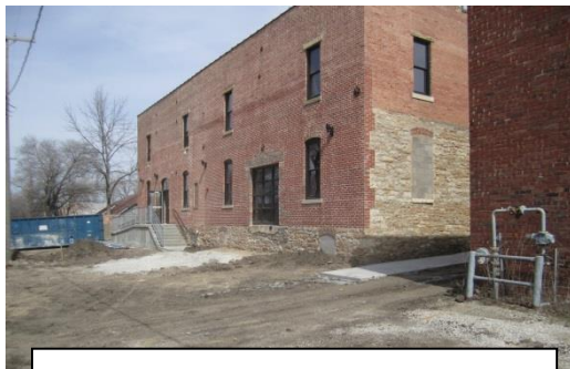
Cider Building During Rehabilitation
