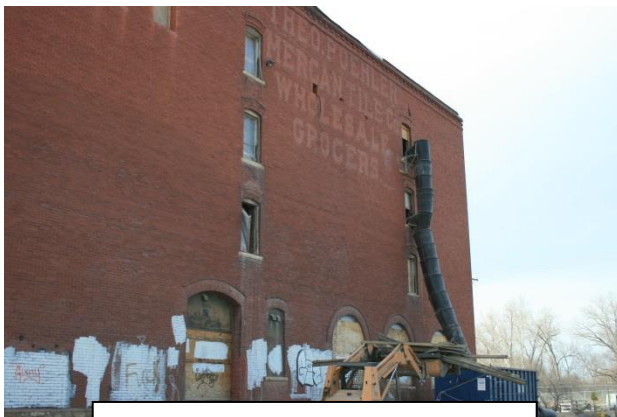
Property Prior to Rehabilitation
