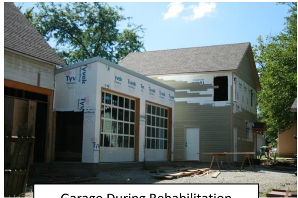
Garage During Rehabilitation
