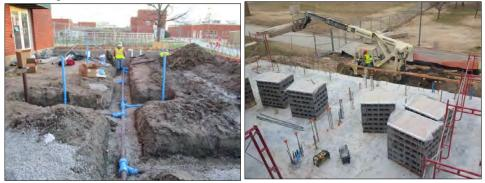
*Fall 2015 – Ongoing –* Dewatering and excavation at Pump Station 10 site located at the northwest corner of 31<sup>st</sup> and Louisiana Streets, with station construction and pipe installation ongoing throughout 2016 and 2017.
