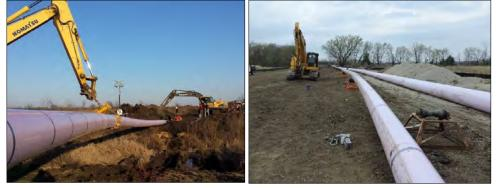
*June 2015 – Ongoing* - Wakarusa WWTP site construction. The first significant task was excavation for the biological nutrient removal (BNR) basin, final clarifiers and UV disinfection building. Formwork, rebar installation and concrete placement are underway on the below-grade slabs and walls in these areas. Installation of sanitary sewer, process piping and electrical ductbank began Fall 2015 and is in progress sitewide.
