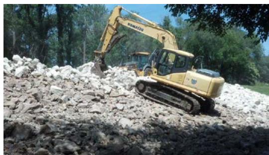
Work on Kansas River Levee
