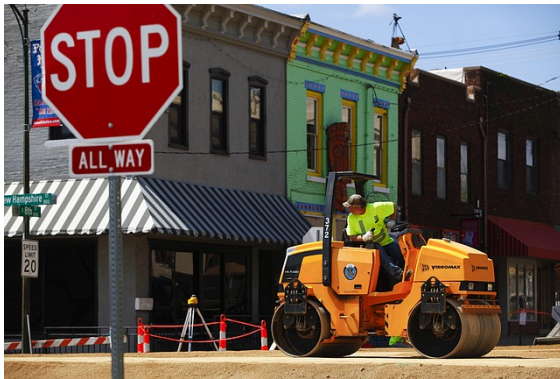
Shot put construction downtown
