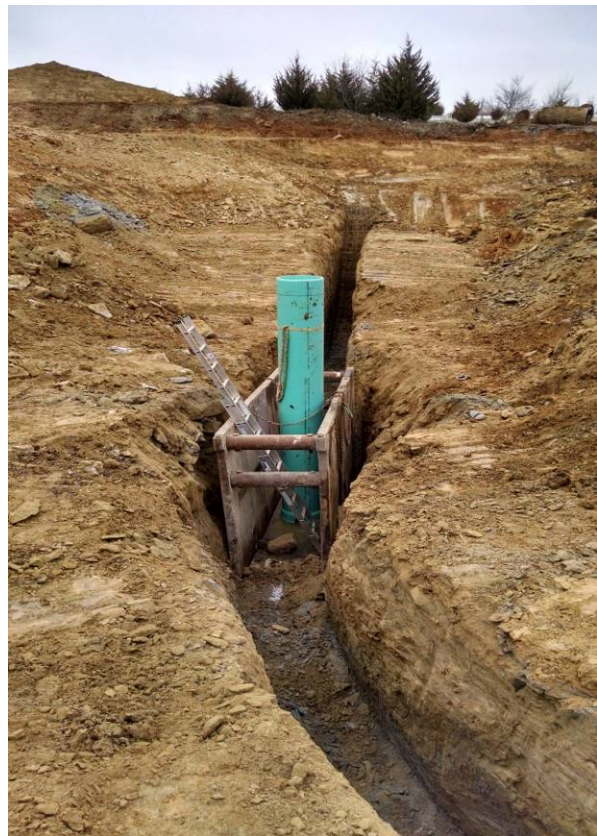
Interceptor Trench construction
