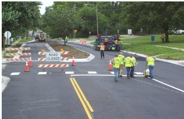
Louisiana Street Mill & Overlay
