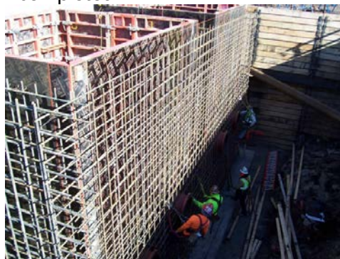
South wall of Maple Street Pump Station
