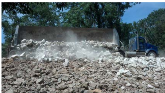
Work on Kansas River Levee
