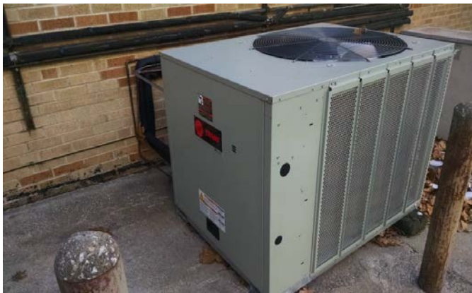
Condenser replacement Douglas County Senior Center
