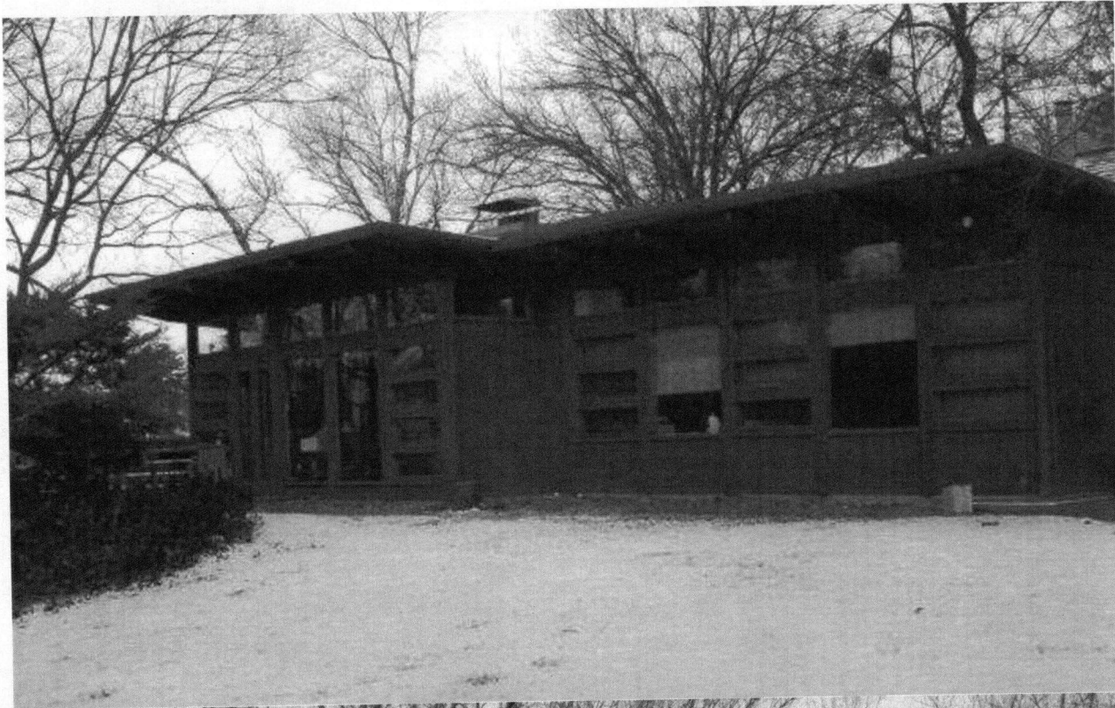
Figure 9. South elevation in 2014 (top) and 1951 (bottom). Top image by John Charlton; bottom image from Lawrence Modern ( http://lawrencemodern.com/bakers-dozen/university-place/post-construction-photos/ ).
