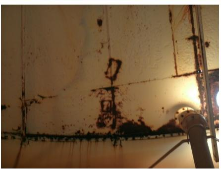
Severe Corrosion and Failed Interior Coating
