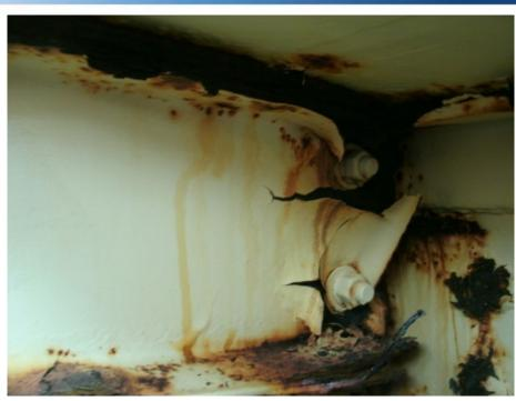
**Roof Beam Corrosion**
