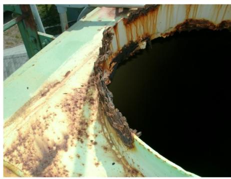
**Roof Hatch Corrosion**
