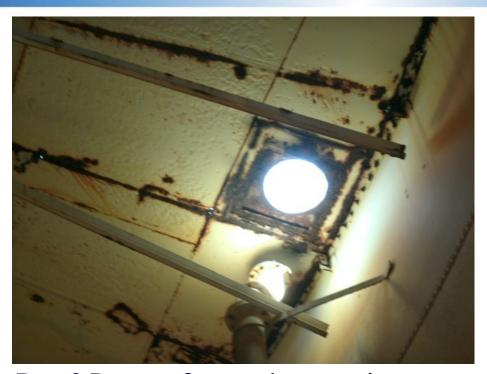
Roof Beam Corrosion and Failed Beams
