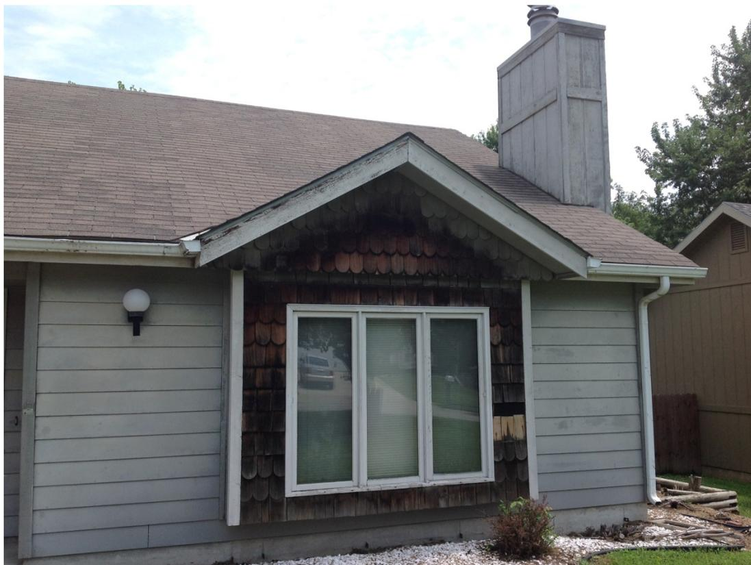
South elevation, rotten chimney chase
