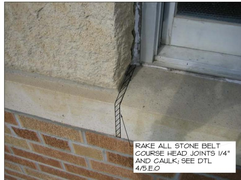
RAKE ALL STONE BELT COURSE HEAD JOINTS 1/4" AND CAULK; SEE DTL 4/5.E.O
