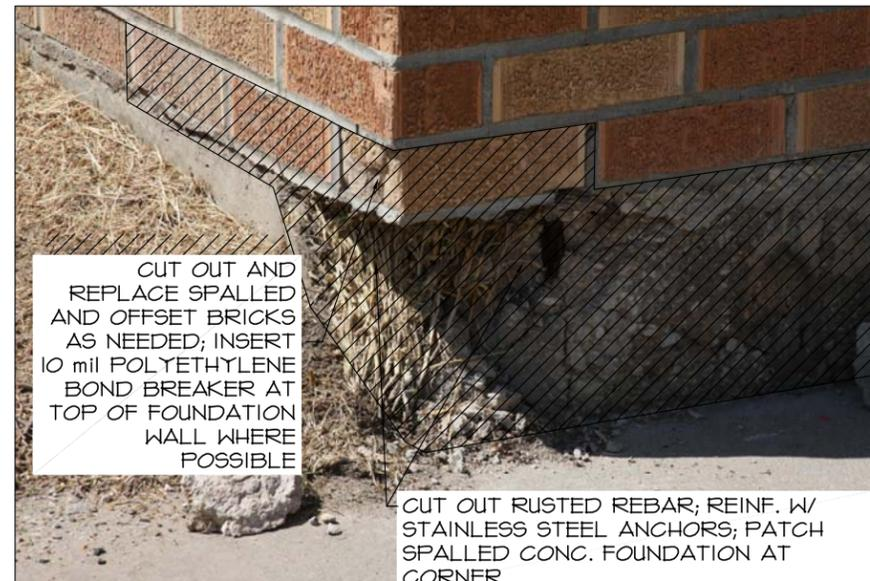
CUT OUT AND REPLACE SPALLED AND OFFSET BRICKS AS NEEDED; INSERT 10 mil POLYETHYLENE BOND BREAKER AT TOP OF FOUNDATION WALL WHERE POSSIBLE
