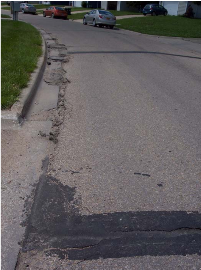
Overland Dr, Monterey Way to Eldridge St (Residential, PCI = 52.3)
