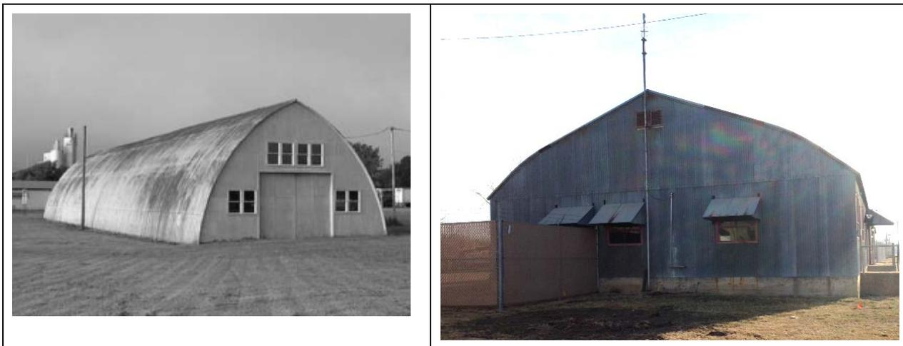
While there are some similarities to the EmKay, the structure at 620 E 8<sup>th</sup> does not have the arch system to the ground but has side walls. The structure at 620 E 8<sup>th</sup> is also 42' X 121'.
