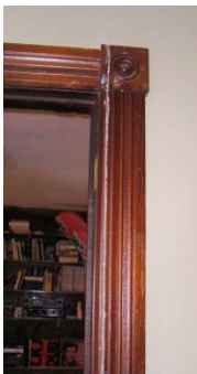
customized wood trim around windows with alteration of chamfered edges with notching and embellished bullet blocks.
