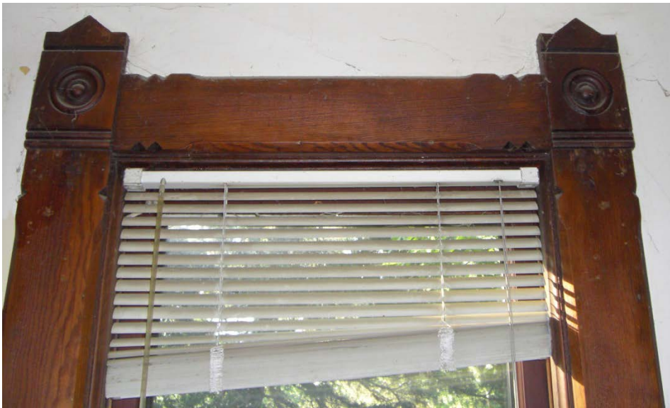
customized wood trim around windows with alteration of chamfered edges with notching and embellished bullet blocks.
