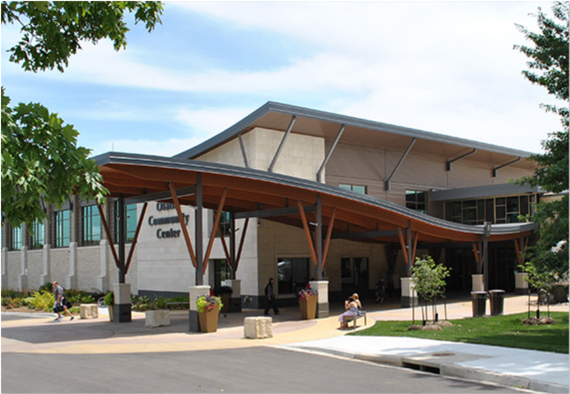
Olathe Community Center
