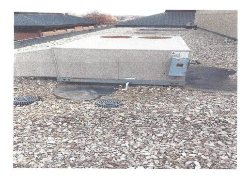
The mechanical unit on the north roof area is not high enough above the roof to flash properly. This unit would need to be raised about six to eight inches above the existing height. NRCA recommends that all mechanical curbs be a minimum of eight inches.
