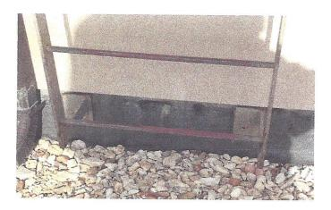
When secondary items were installed, mechanical fasteners were run directly through the base flashings of the membrane. This should never happen. These types of details would be corrected at the time of the new roof.
