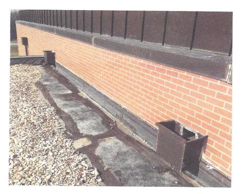
The short masonry wall on the south side of the facility appears to have the weep holes in the brick covered up by the existing roof; or they were never installed. This is another area where the interior could be showing up as a leak. It appears that someone attempted roof repairs on the membrane with an asphalt product that is not supposed to be used on this type of roof.
