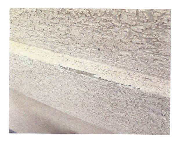
There are many areas around the EFIS wall assembly that are open and allowing water to enter the assembly. This also allows the insulation to get wet causing it to lose its insulating properties as well as freeze up in the winter causing further damage to the EFIS.
