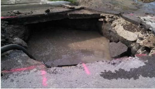
The water main leak caused a large hole, 20 ft x 10 ft on East 19<sup>th</sup> Street and Bullene.
