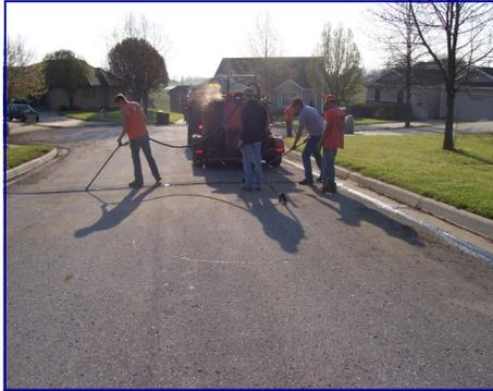
**What Is Crack Sealing?** A key preventative maintenance technique where small cracks are filled with a rubberized asphalt product creating thick "snake like" lines on the street. Sealing the cracks helps prevent water from getting into the street pavement and causing potholes.
