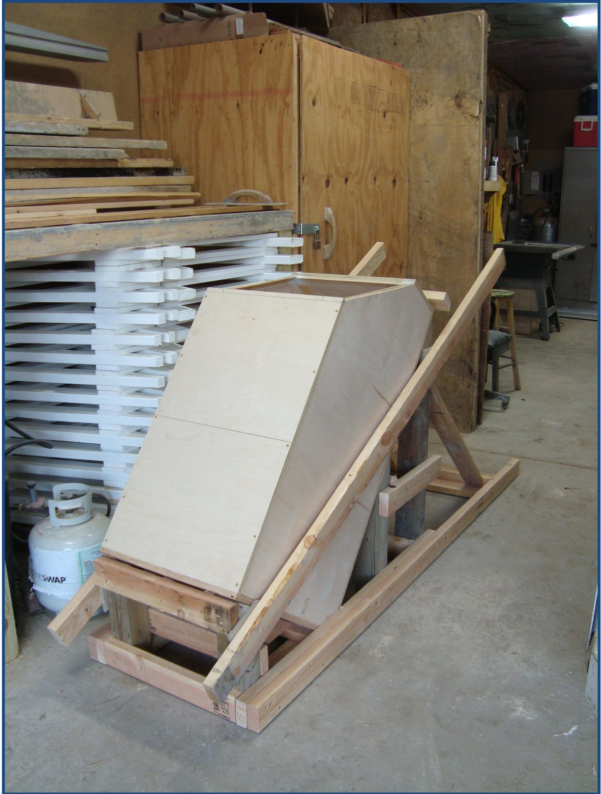
Form for the new pedestal
