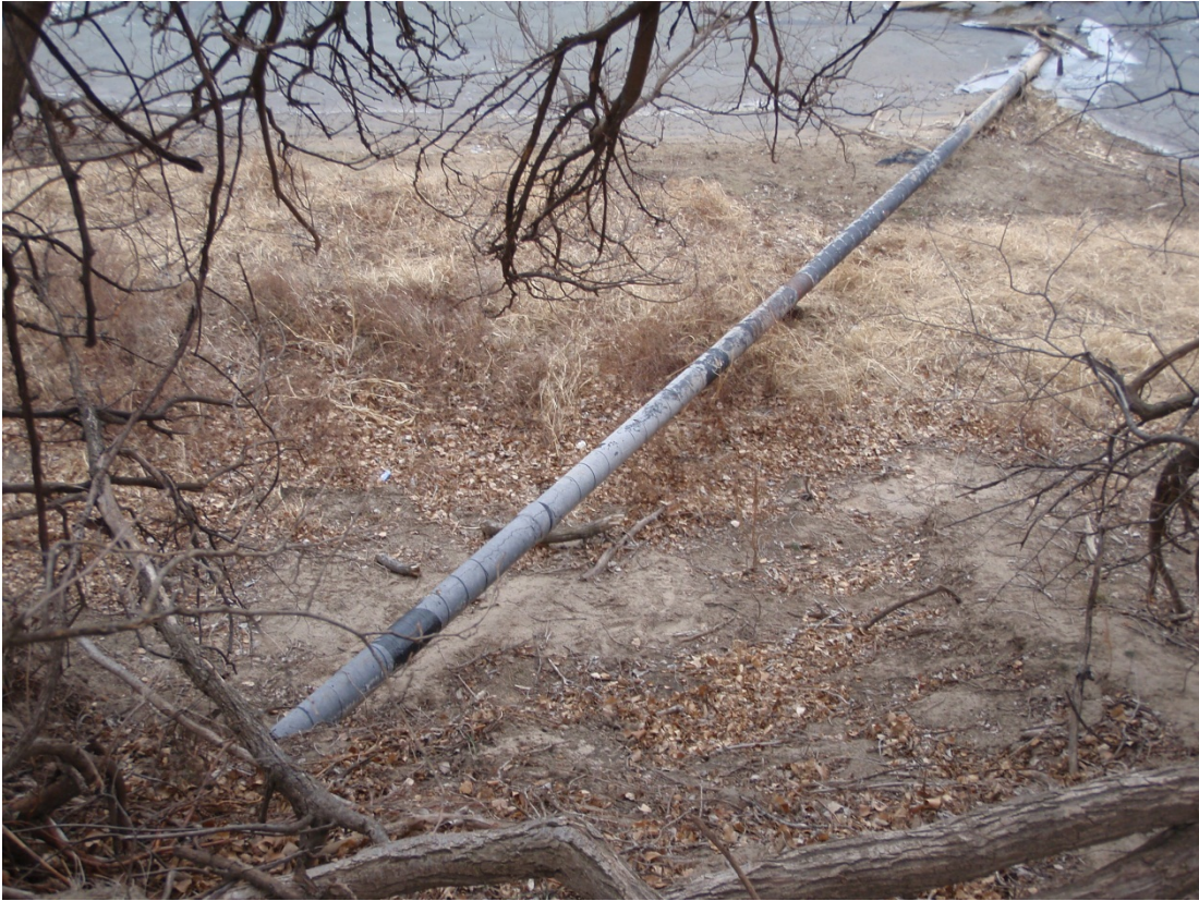
Exposed forcemain looking south from the north riverbank.
