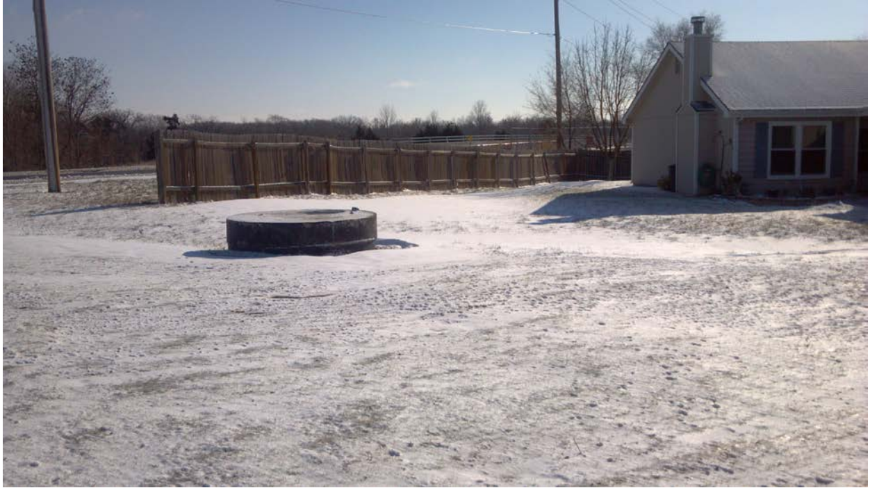
Existing Manhole SW241219-041
