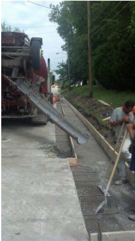
**Description** – During Contracted Concrete Patching & Curb Replacement on N 3<sup>rd</sup> St north of Maiden Ln.
