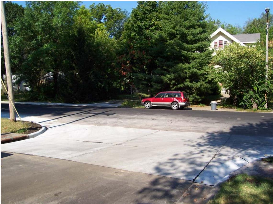
**Description** – Pawnee Ave at Massachusetts St after completion of Contracted Asphalt Overlay (Installed Concrete Intersection Approach seen here also).
