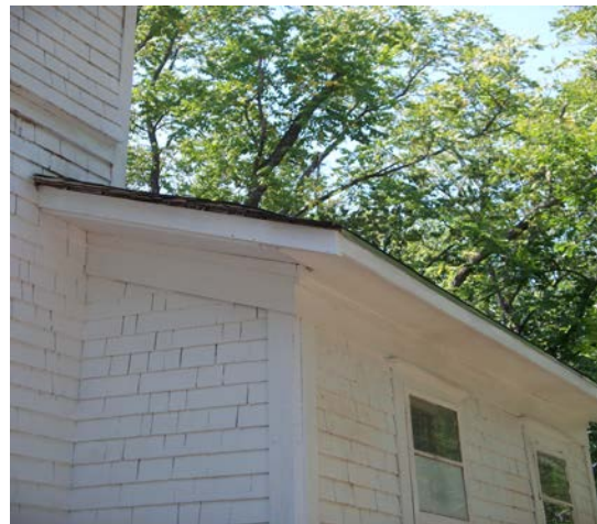
1313 Haskell Ave. N.W. roof & eaves repaired
