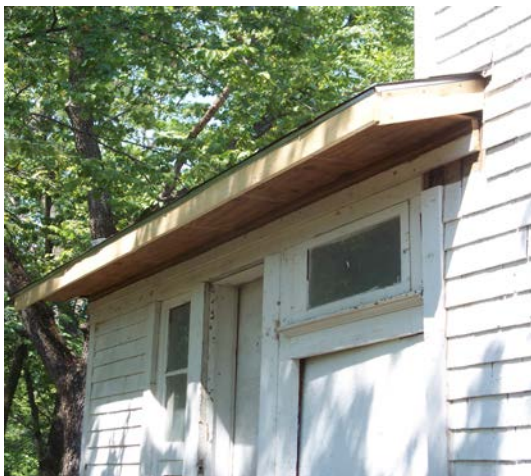
1313 Haskell Ave. S.W. roof & eaves repaired
