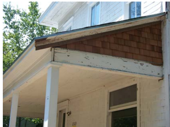
1313 Haskell Ave. Porch roof & eaves repaired
