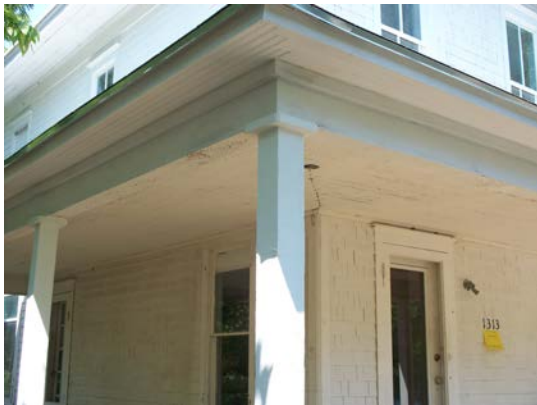
1313 Haskell Ave. Porch bead board soffits & roof repair
