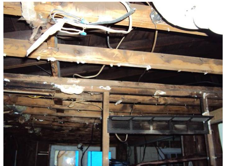
Fire damaged electrical boxes in ceiling (1<sup>st</sup> floor)
