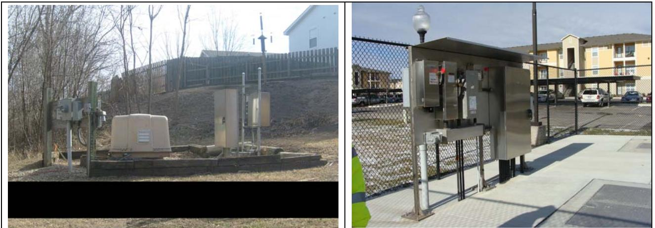
**Figure 3.** Existing pump station on the left. Example of new station (without the fencing) Underground facilities will be level-or slightly elevated and the panel will contain the above ground equipment.
