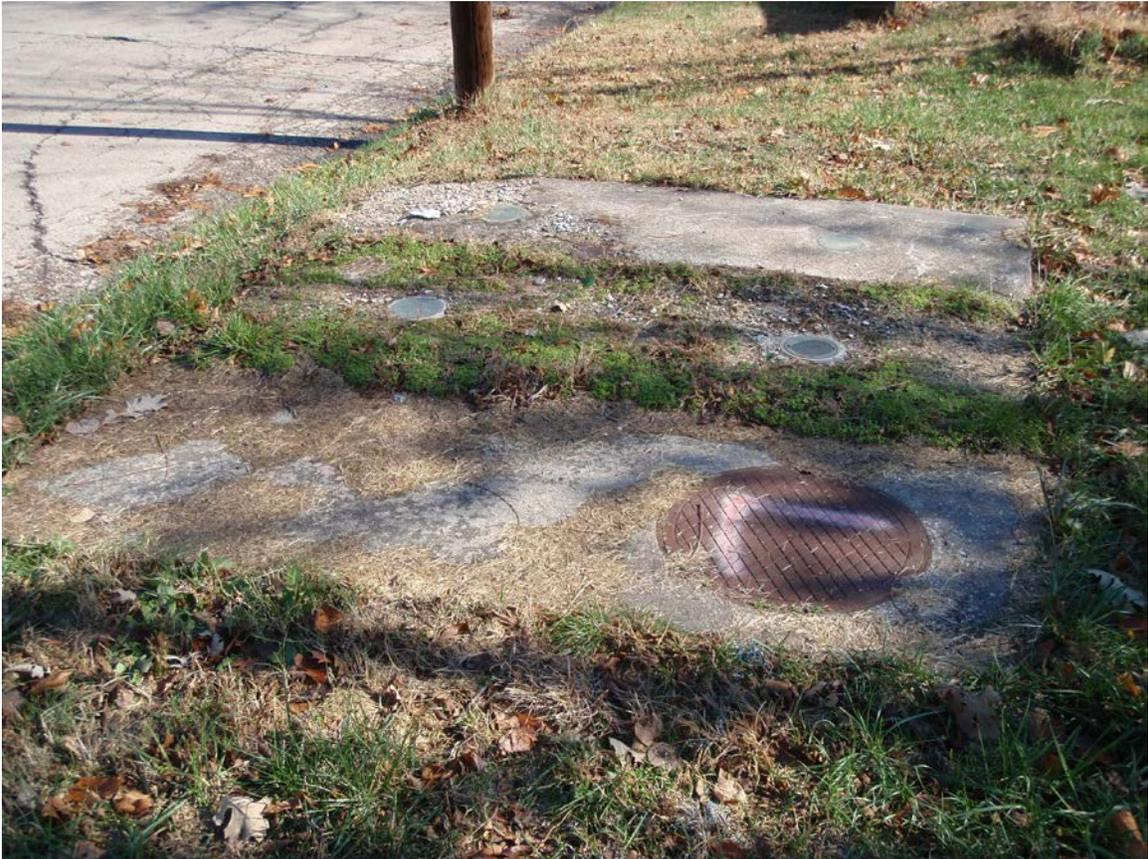
Kaw WTP East Vault in 3<sup>rd</sup> Street ROW – 1955 24" Gate and Check Valve and Vault
