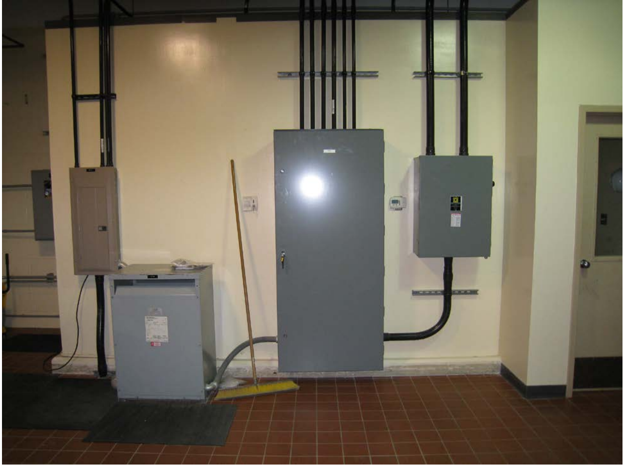
Completed 480 Volt Power Panel
