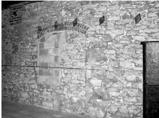
Existing brick and stone masonry – Zone 1
