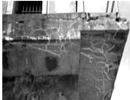
Common conditions of historic concrete – spalling (left) and cracking (right)
