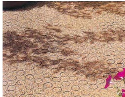
Example of compacted gravel system
