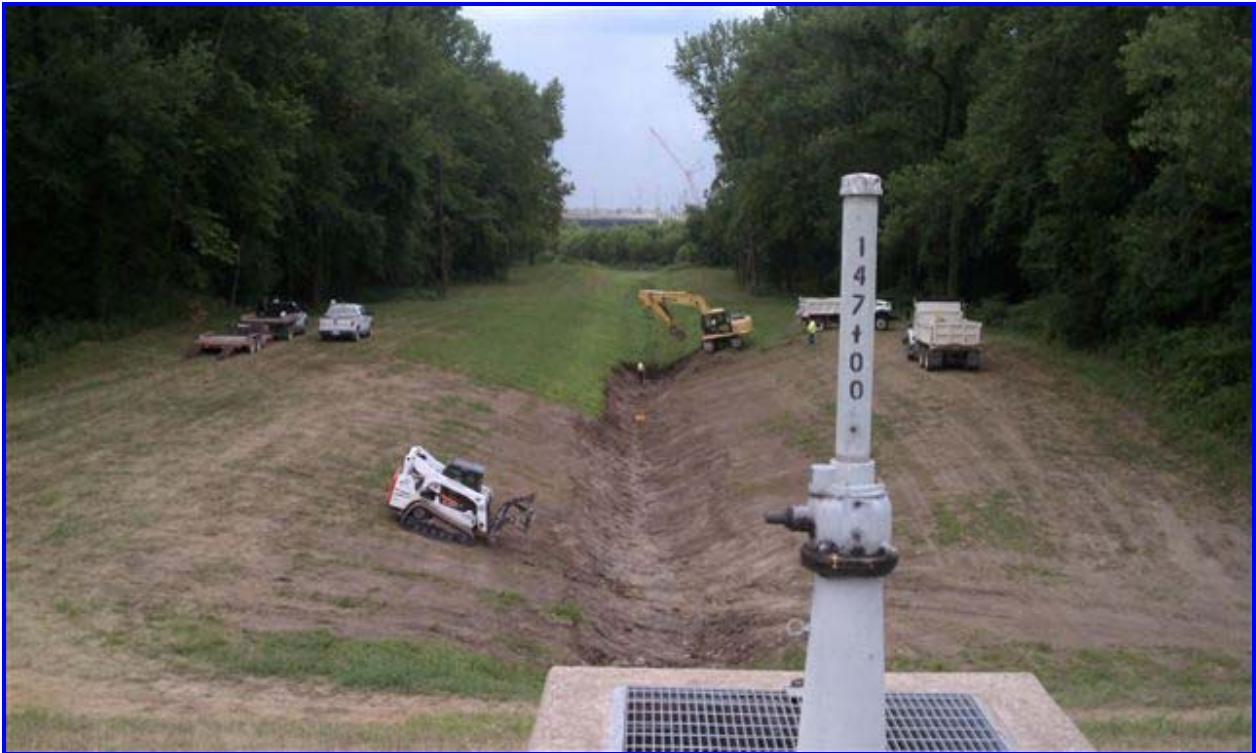
Levee Crew reshaping and clearing a drainage structure to the KAW
