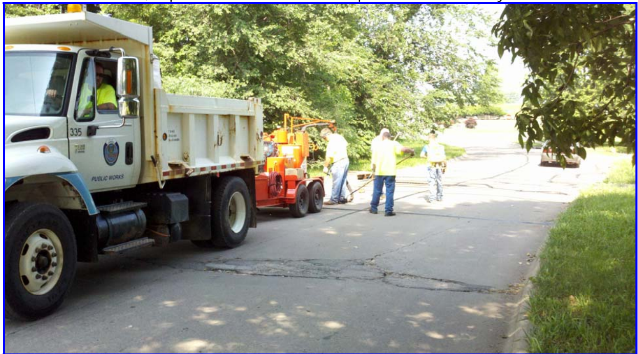
Asphalt Crew crack sealing
