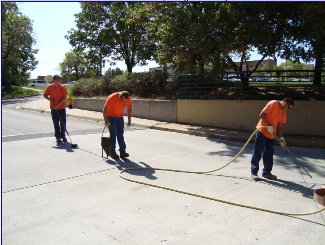
Asphalt crew joint sealing new speed cushion at the River Front parking garage
