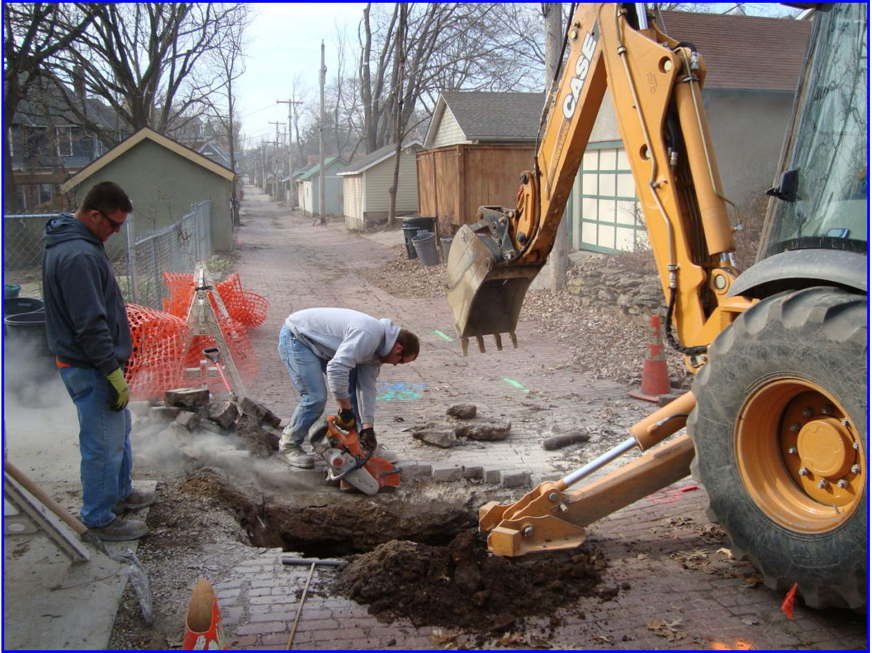
Concrete Crew repairing brick alley
