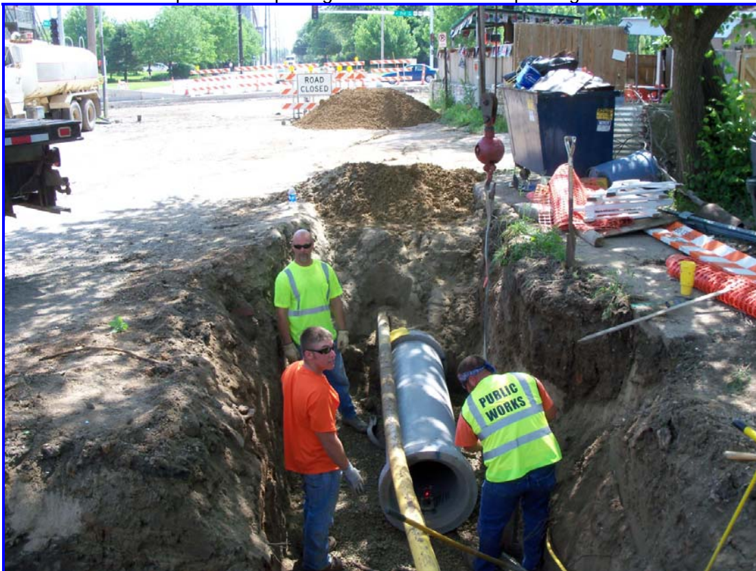
Storm Water Crew installing new storm sewer pipe
