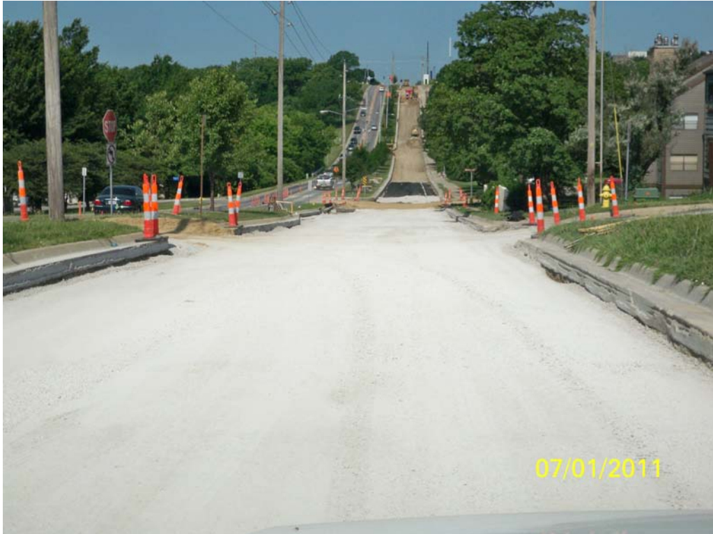
Description – Contracted Reconstruction of westbound driving lanes of Bob Billings Parkway east of Kasold Dr during Pavement Removal and Subgrade Preparation & Treatment
