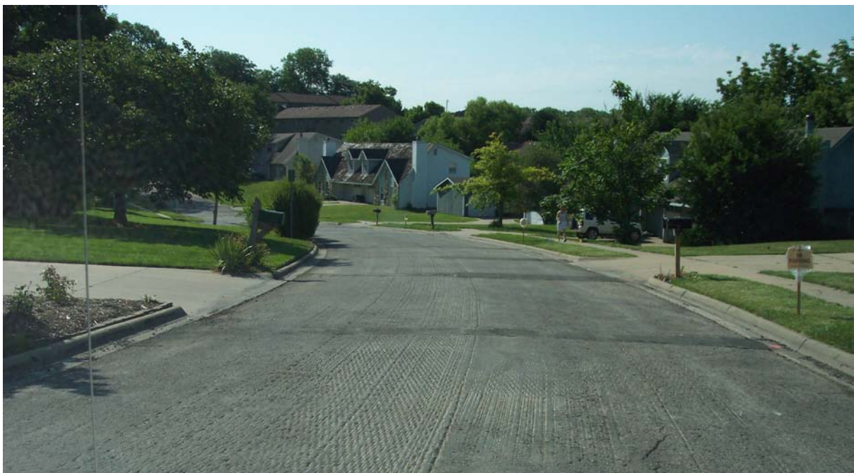
Description - Contracted Milling and Patching on Oxford Rd to University Dr prior to Overlay
