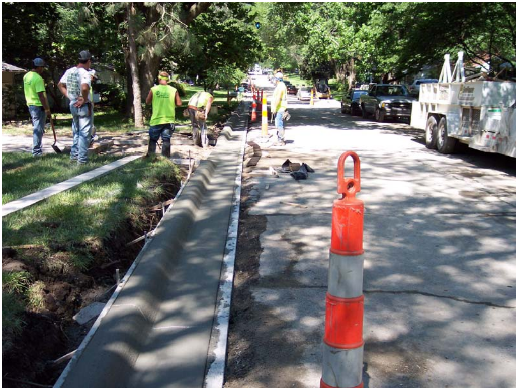
Description – Contracted Concrete Curb & Gutter work prior to Milling & Overlay on W 22 nd St between Ousdahl Rd & Naismith Dr
