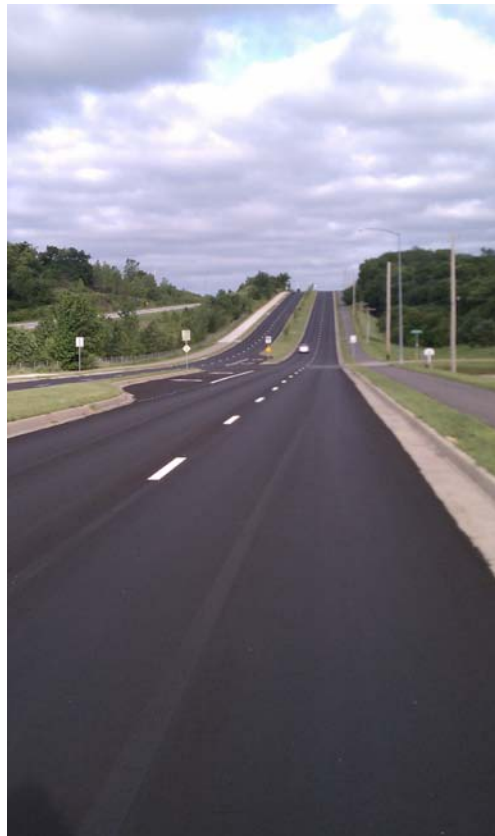
Description – Contracted Microsurfacing/Patching w/ Pavement Markings on Clinton Parkway west of Wakarusa Dr
