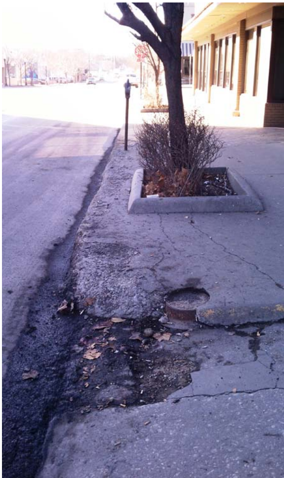
Description – Contracted Concrete Curb & Gutter Repair with Concrete Pavement Patching in Downtown Lawrence (left picture - prior to work, right picture - during removal/replacement)
