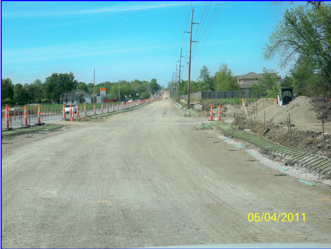
Kasold looking north – subgrade ready for concrete
