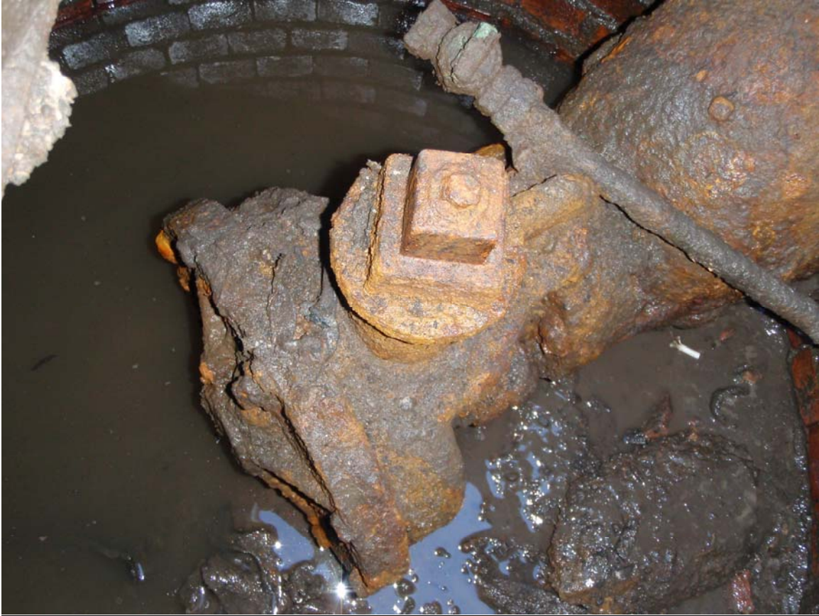
20" Gate Valve 8 th & Kentucky - Valve operator and manhole
