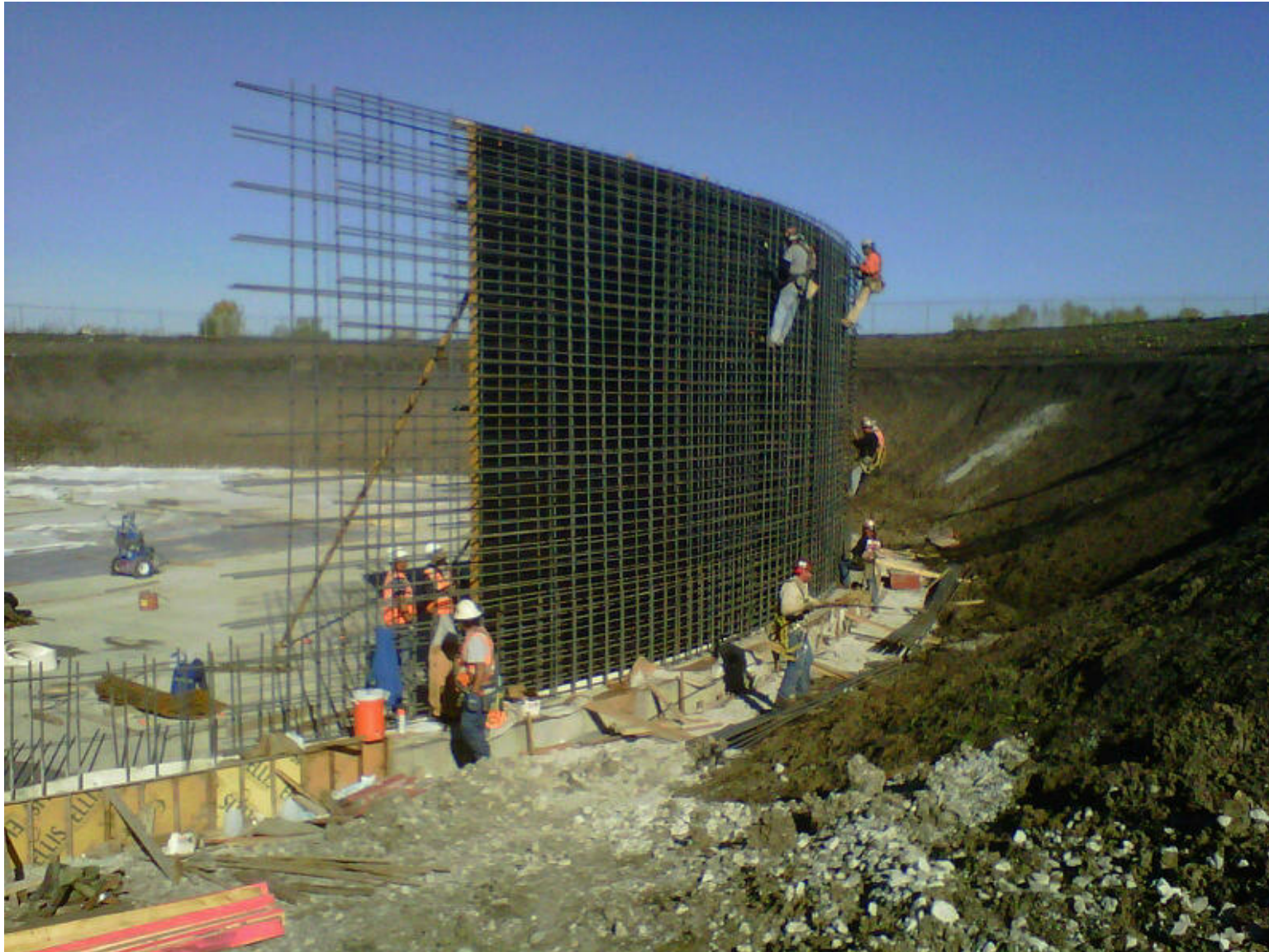
Iron workers placing rebar for a basin wall concrete pour.
