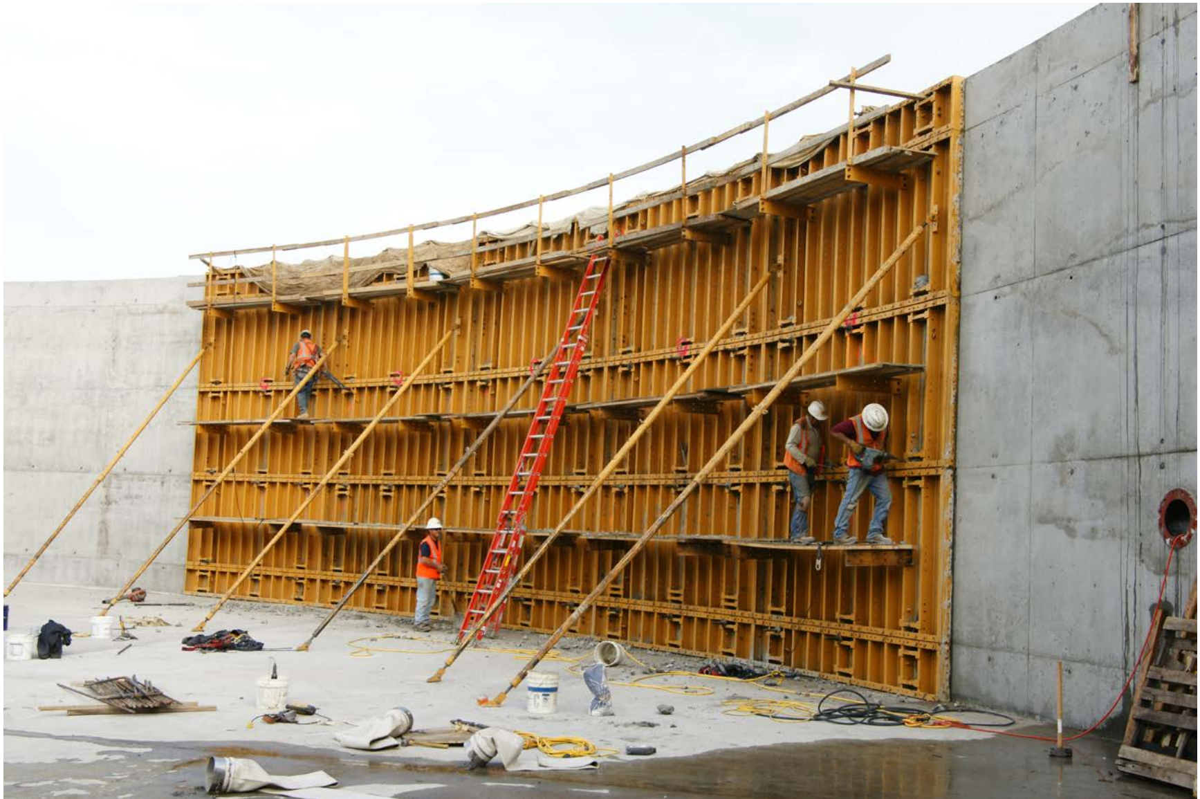
Inside view of basin wall and concrete form work.
