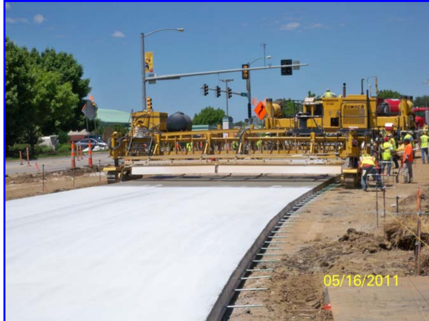
Kasold (north bound lanes 31 st to 23 rd ) Approximately 4,500 Cubic Yards of concrete poured
