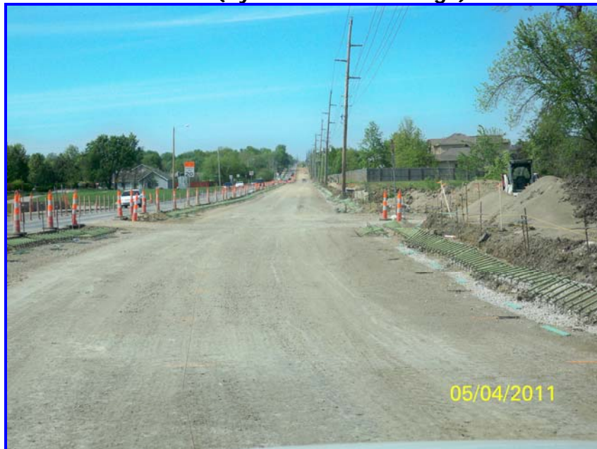
Kasold (flyash treated subgrade ready for concrete)
