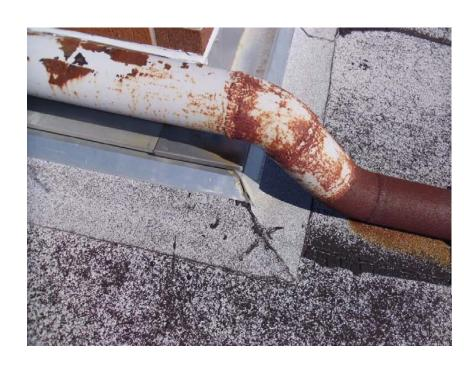
Gas lines will be coated with rust prohibitive coating to prevent further damage.
