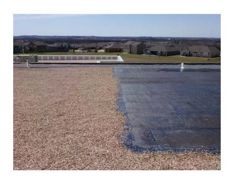
Crews apply cold asphalt then coat with gravel. The cold asphalt imbeds the 3/8-5/8 inch pea gravel and holds it tight against the asphalt membrane.
