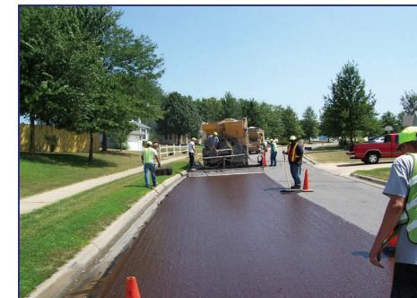
**What Is Microsurfacing?** Microsurfacing is a preventative street sealing technique that uses a pre-mixed slurry of rock, polymer asphalt binders, cement, and filler materials to seal the entire roadway at a depth of about 3/8th of an inch. It is applied over the top of the pavement.
