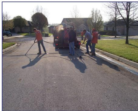
**What Is Crack Sealing?** A key preventative maintenance technique where small cracks are filled with a rubberized asphalt product creating thick "snake like" lines on the street. Sealing the cracks prevents water from getting into the street and causing potholes.
