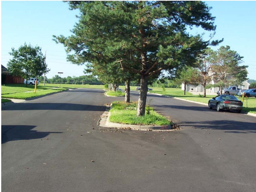
Description – Contracted Milling & Overlay (Phase 1) on Atchison Ave near 31 st St
