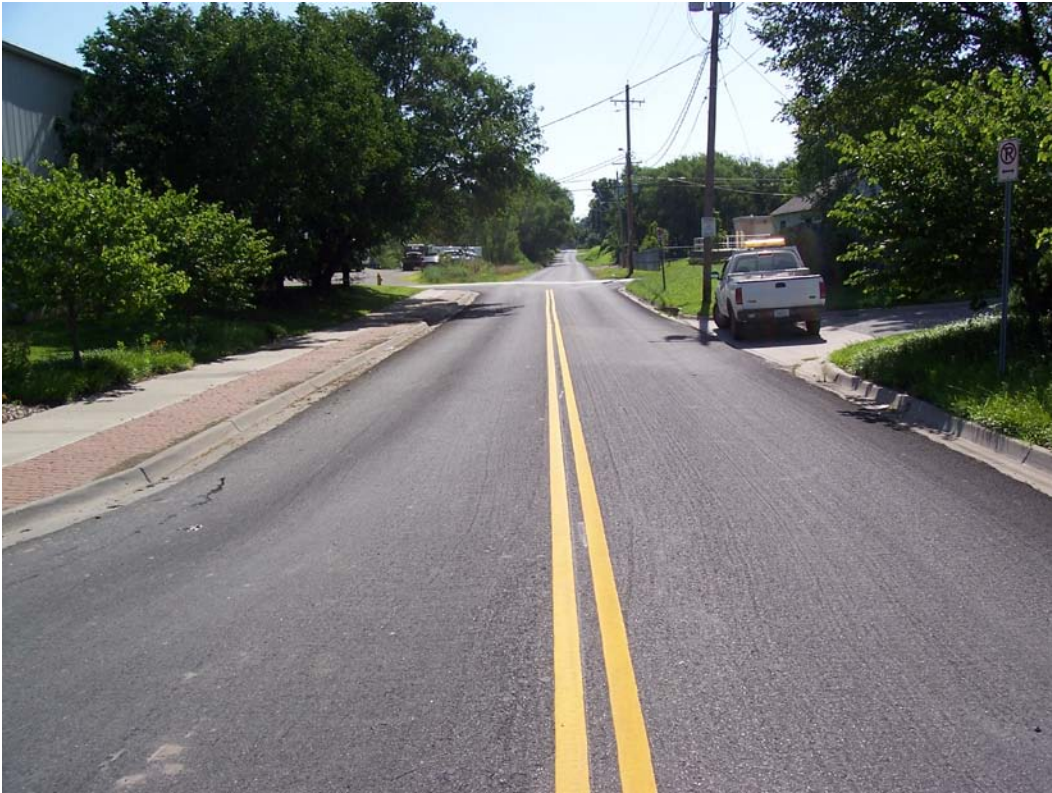
Description – Contracted Microsurfacing/Patching w/ Pavement Markings in north Lawrence
