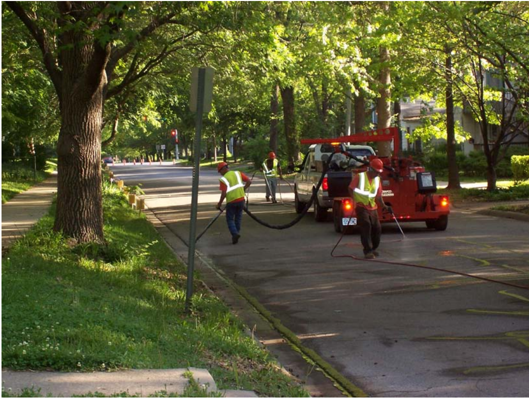
Description – Contracted Crack Sealing
