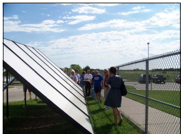
The Sustainable Homes Tour also visited the Douglas County Jail which has installed 200 square feet of solar collection to heat domestic water.
