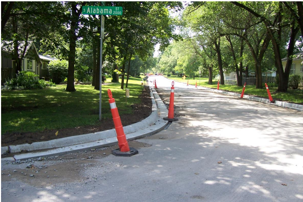
Description – Curb & Gutter Removal & Replacement on 20 th St west of Alabama St as part of Contracted Milling & Overlay (Phase 2)
