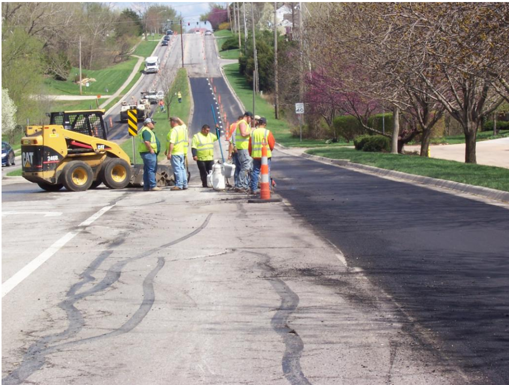
Description – Bob Billings Parkway near Wagon Wheel Rd after Contracted Milling and Overlay Patching as part of Emergency Repair and Rehabilitation
