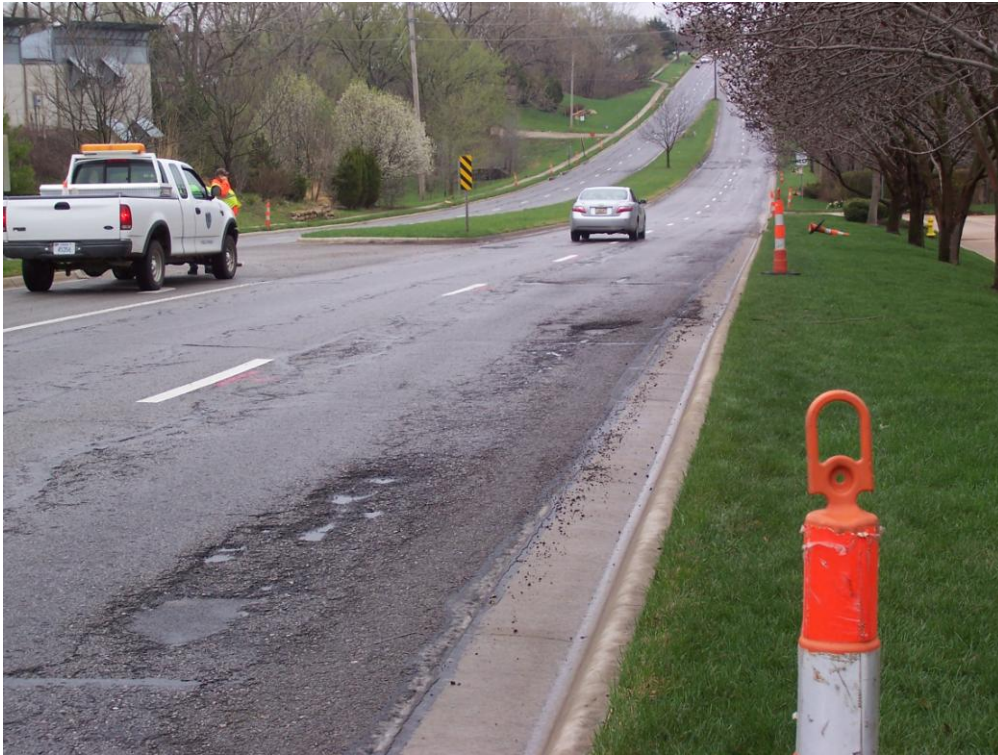
Description – Condition of Bob Billings Parkway near Wagon Wheel Rd prior to Contracted Milling and Overlay Patching as part of Emergency Repair and Rehabilitation
