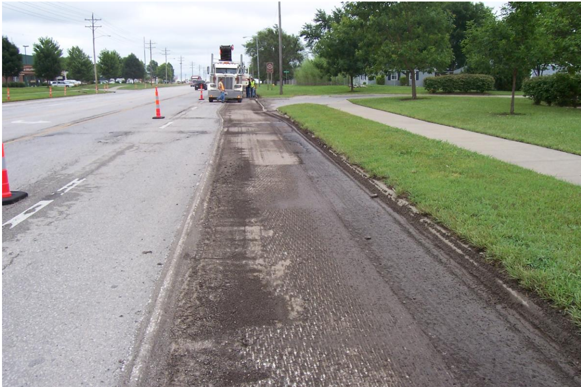
Description – Condition of E 23 rd St east of Harper Ave during Milling as part of E23rd St KLINK Milling and Overlay Project
