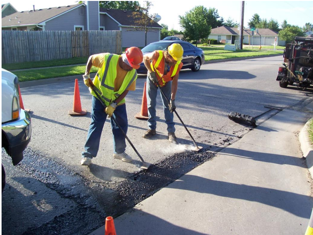
Description – Contracted Crack & Joint Filling w/ "PolyPatch" on Monterey Way N of W 6 th
