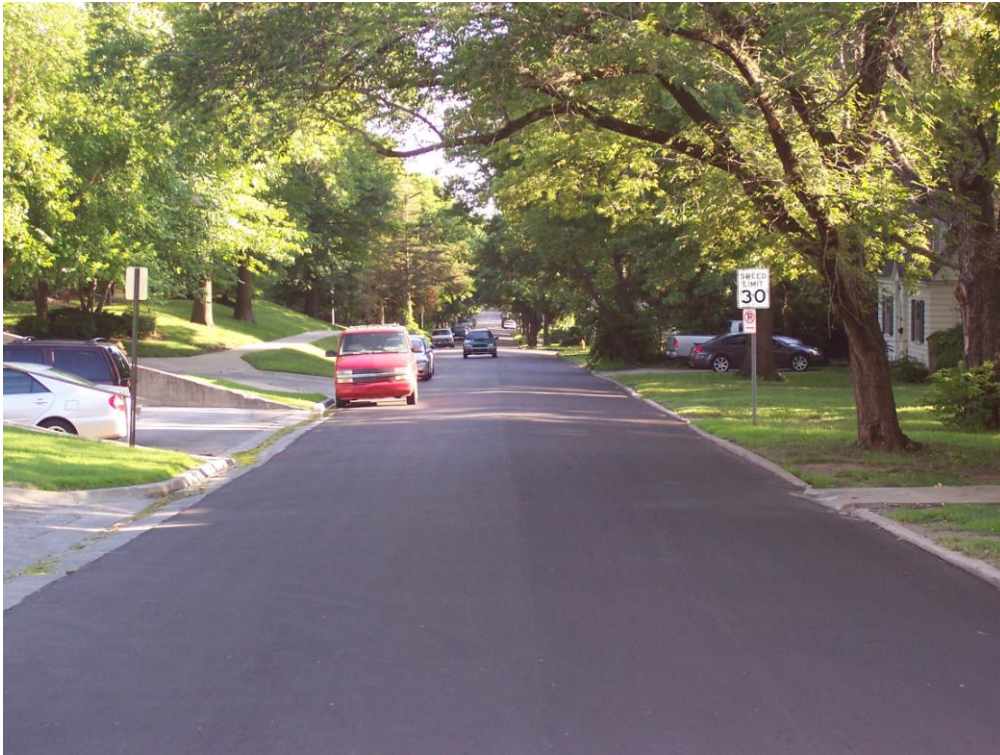
Description – Contracted Milling & Overlay (Phase 1 "Add") on Missouri St near 11 th St
