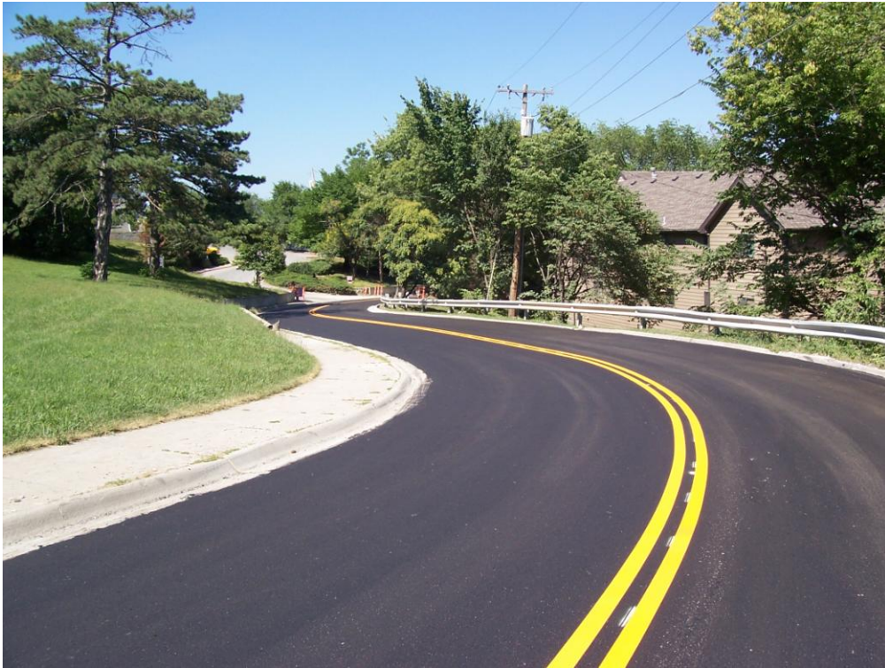
Description – Completed Overlay & Pavement Markings on Emery Rd from 9 th St to High Dr as part of Contracted Milling & Overlay (Phase 1 “Add”)
