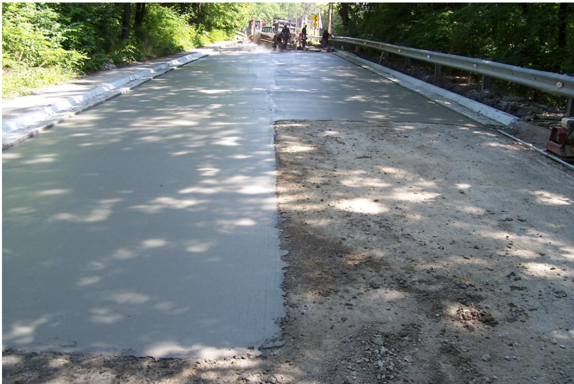
Description – Concrete base repair patching on Emery Rd from 9 th St to High Dr as part of Contracted Milling & Overlay (Phase 1 "Add")
