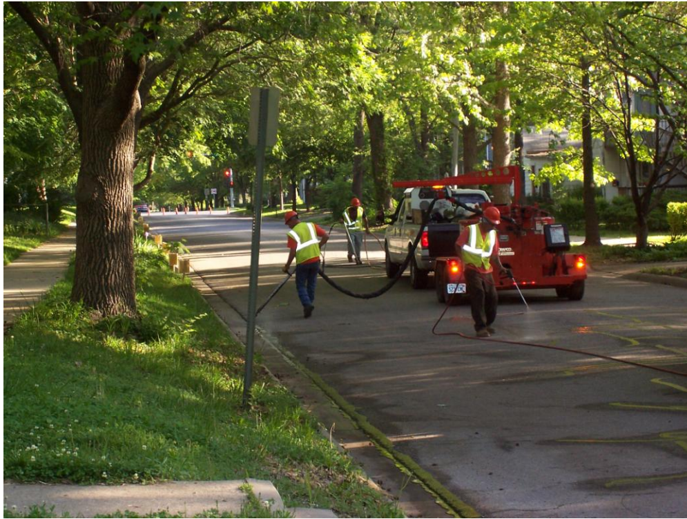
Description – Contracted Crack Sealing
