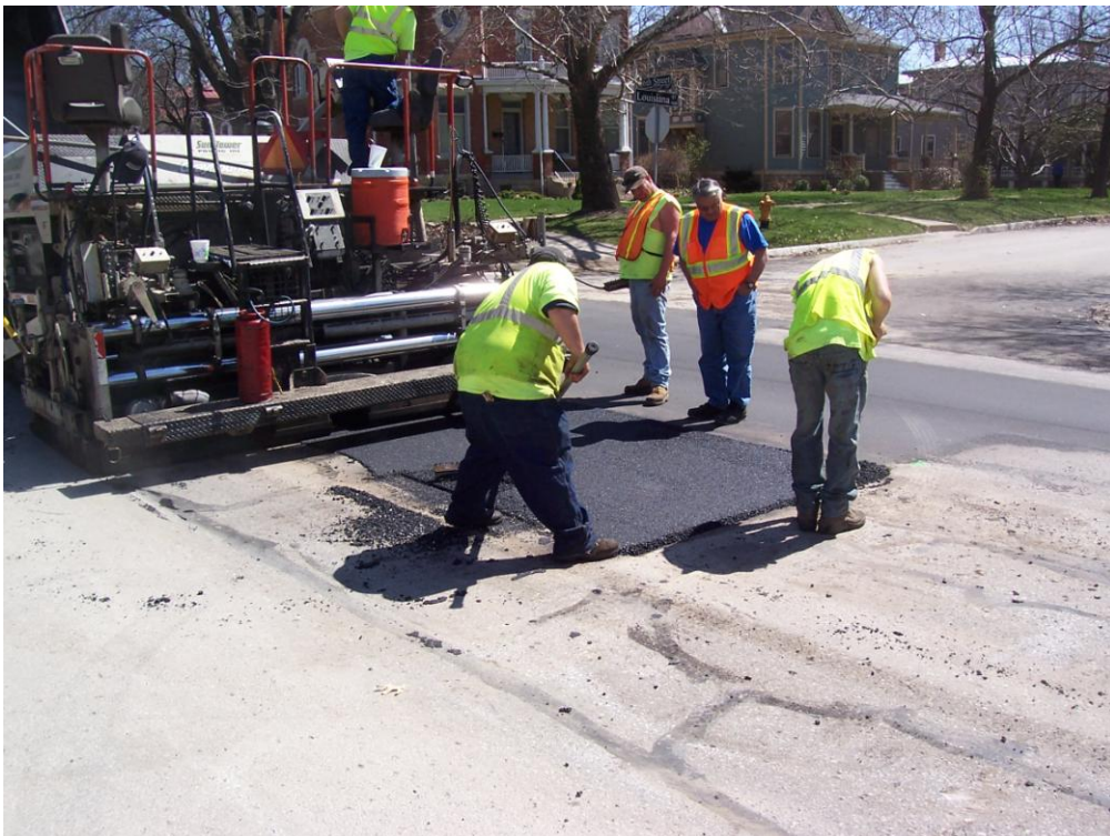
Description - Contracted Milling and Overlay Patching on W 6 th St as part of emergency repair and rehabilitation
