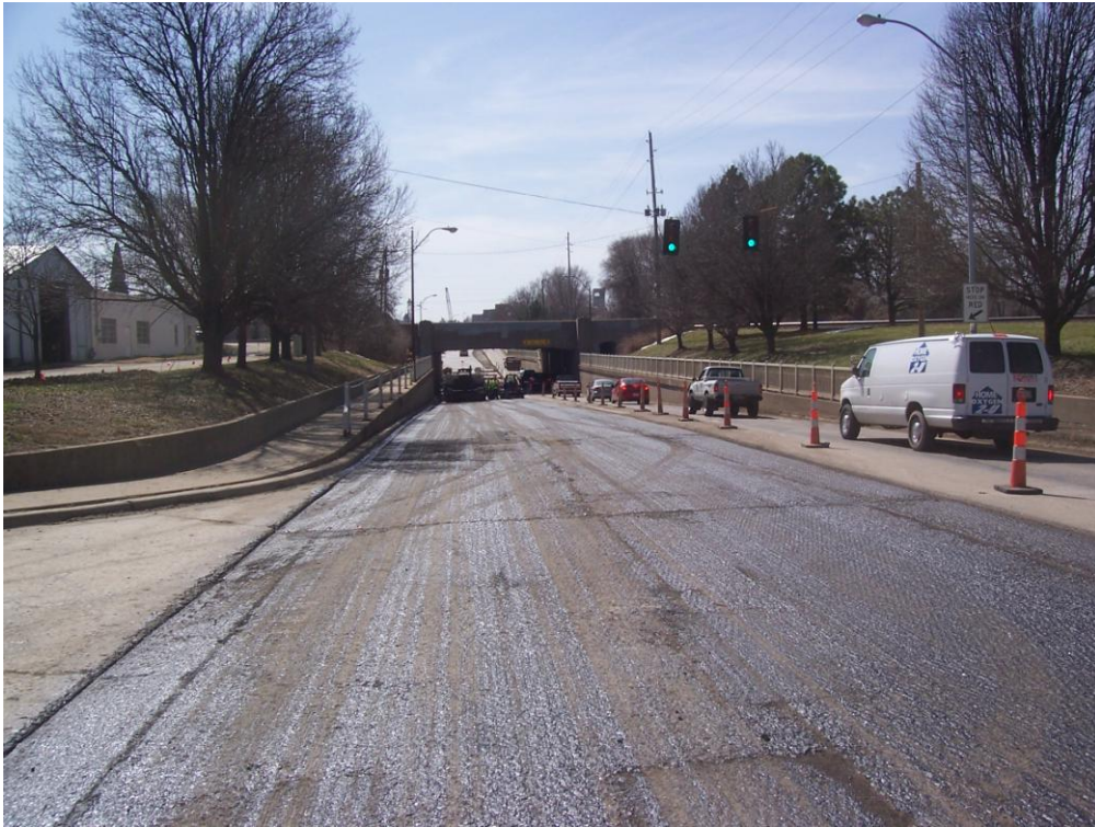
Description – N 2 nd St @ Lincoln St after Milling and just prior to Contracted Overlay as part of Emergency Repair and Rehabilitation in coordination w/ 2 nd & Locust Project
