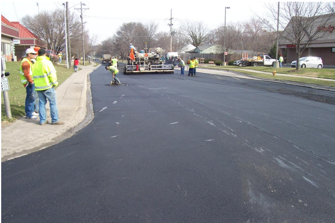
Description – Louisiana St near 23 rd St during Contracted Milling and Overlay Patching as part of Emergency Repair and Rehabilitation
