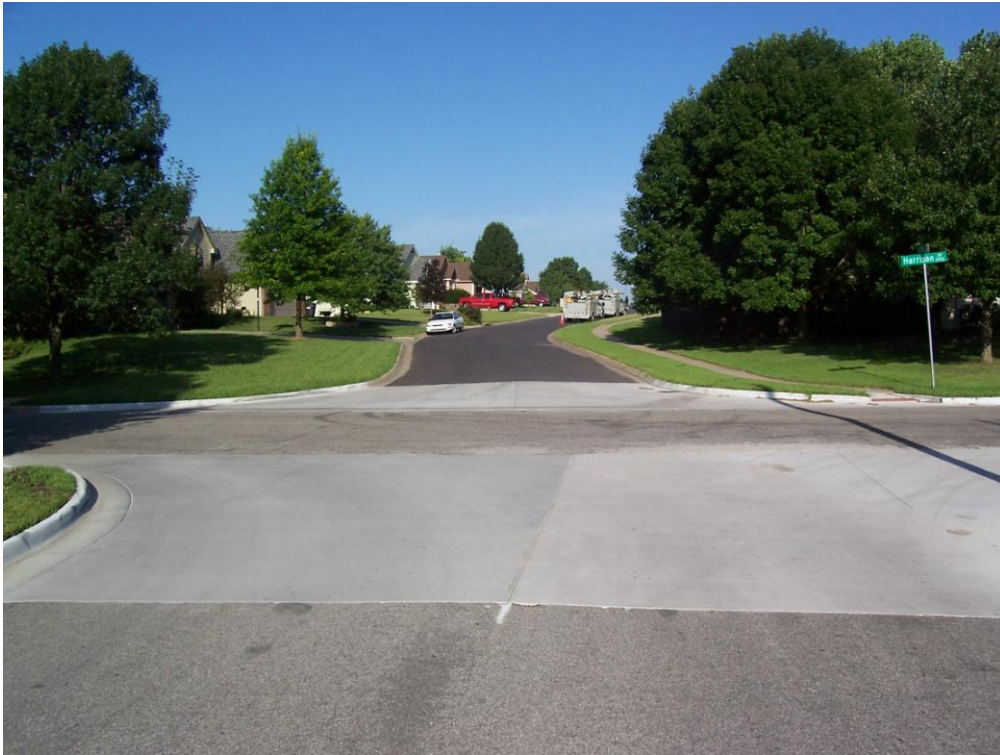
Description – Contracted Milling & Overlay (Phase 1) on 30 th St at Harrison Ave with coordinated concrete intersection work performed by Internal Street Division
