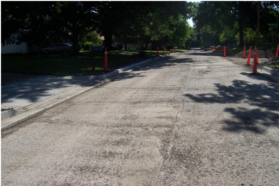
Description – W 20 th St near Mitchell St has been Milled after Curb & Gutter Removal & Replacement as part of Contracted Milling & Overlay (Phase 2)
