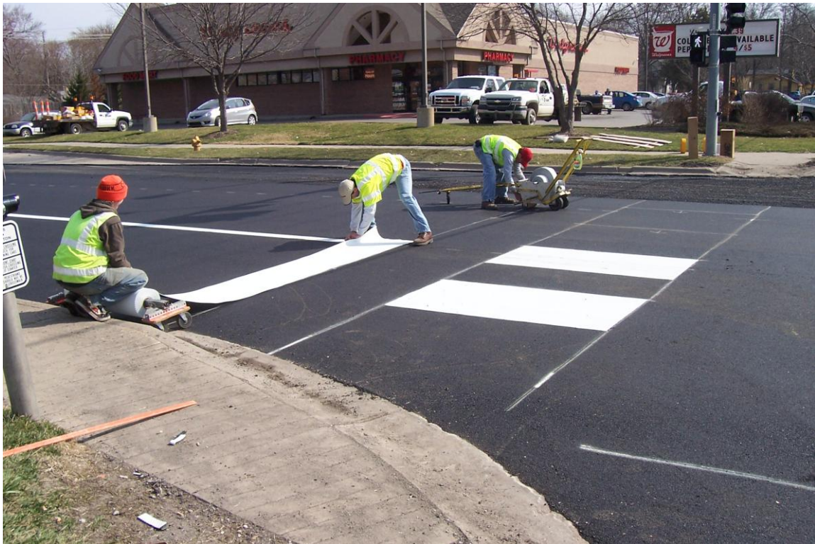
Description – Louisiana St near 23 rd St during Contracted Milling and Overlay Patching w/ Pavement Markings as part of Emergency Repair and Rehabilitation
