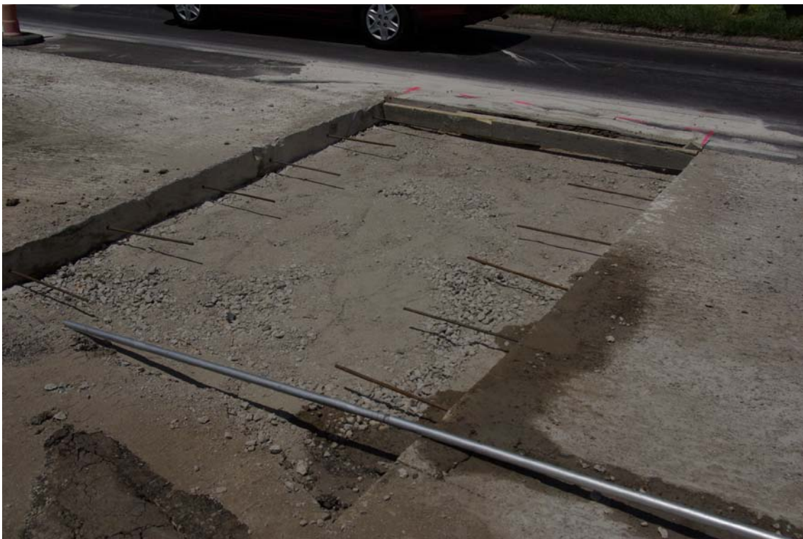
Average size of patching needed per driving lane every 100'.
