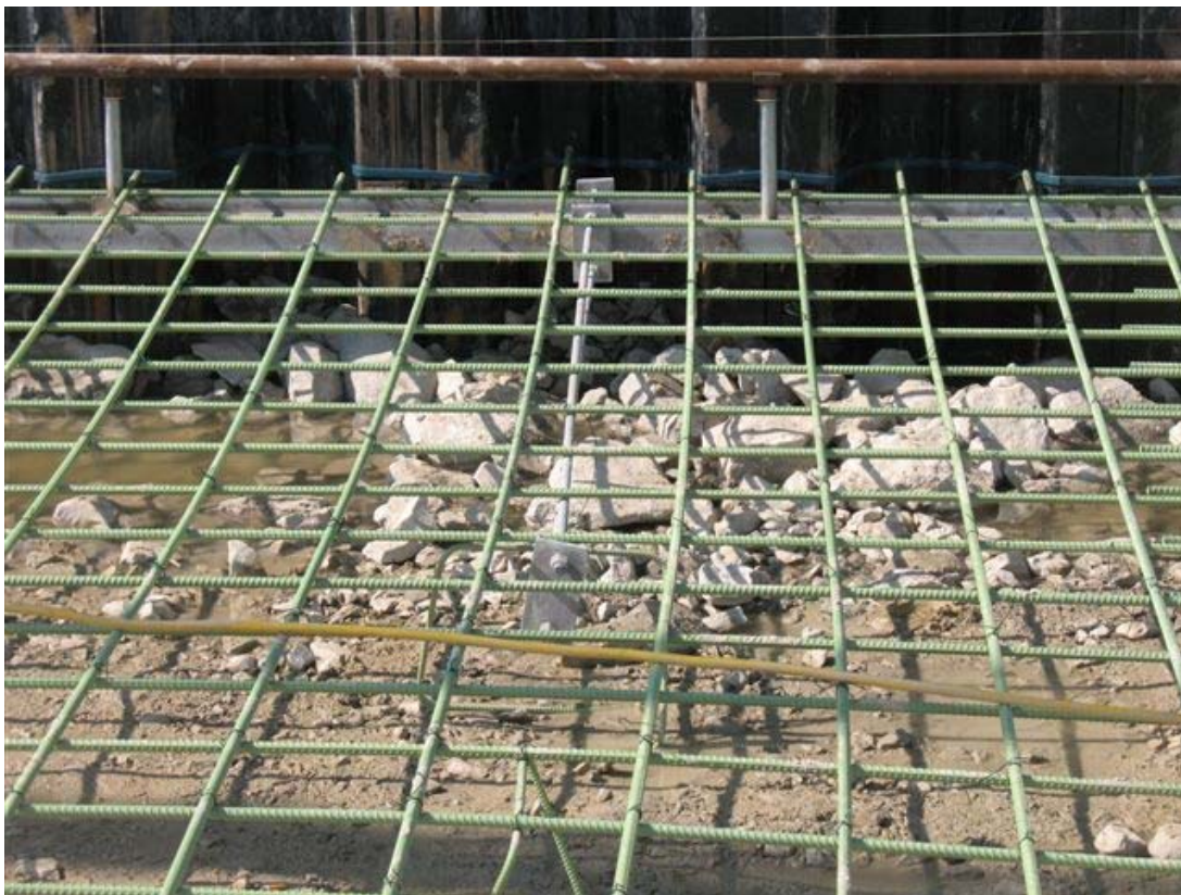
The sheet pile anchor system is visible below the layer of epoxy coated reinforcing steel.
