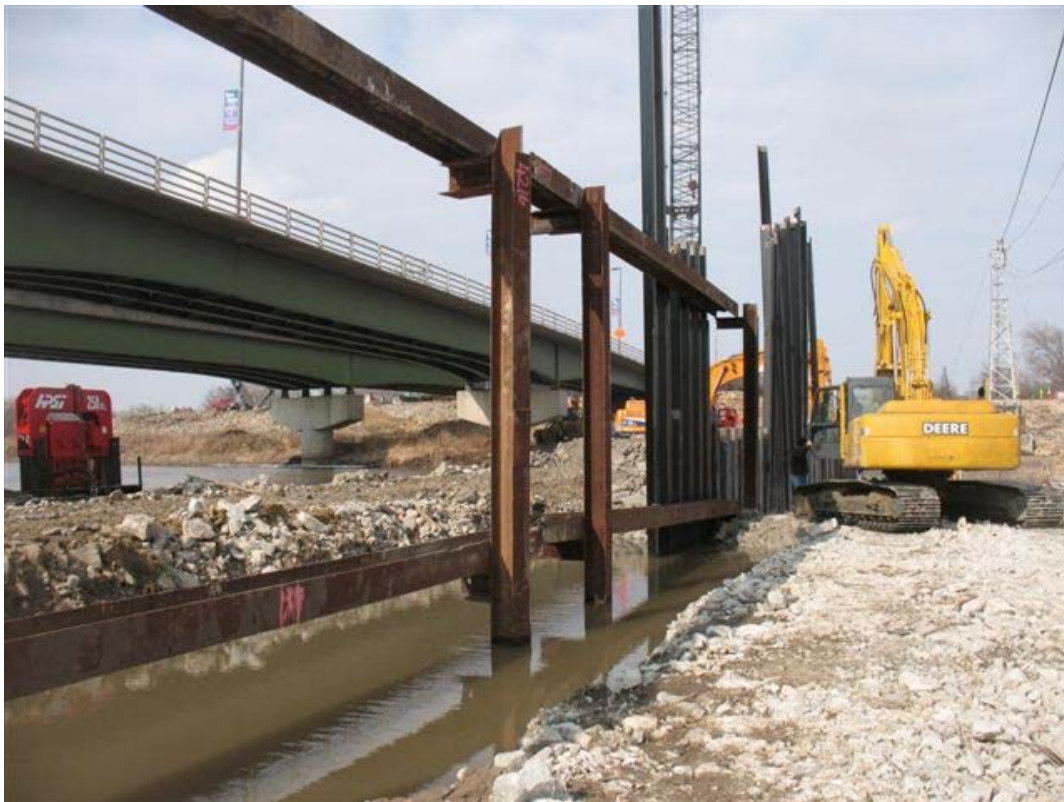
Template used to align sheet pile
