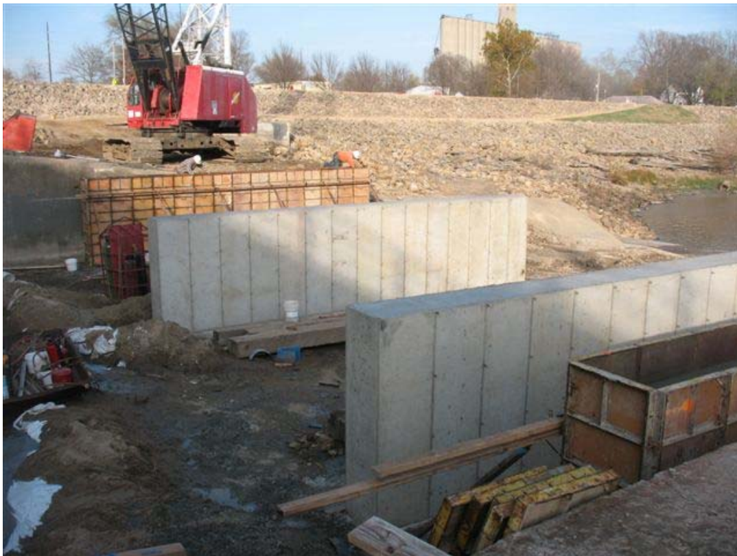
Middle bents of the temporary bridge spanning the spillway.
