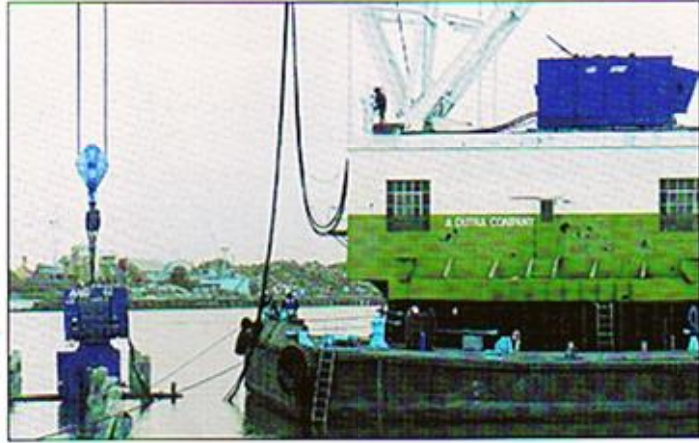
Model 450 Extracting 24" Concrete Pile
