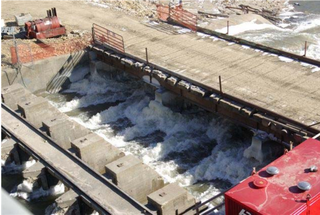
Completed temporary bridge across spillway
