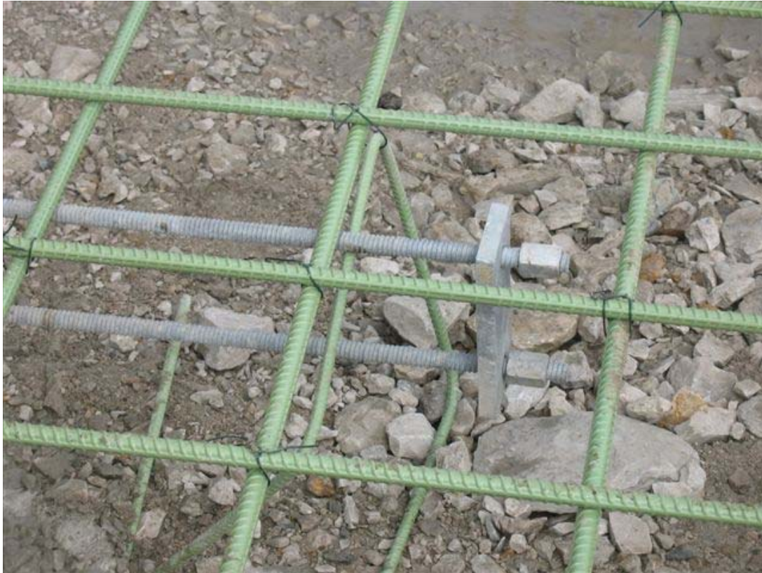
Sheet Pile Anchor – free end
