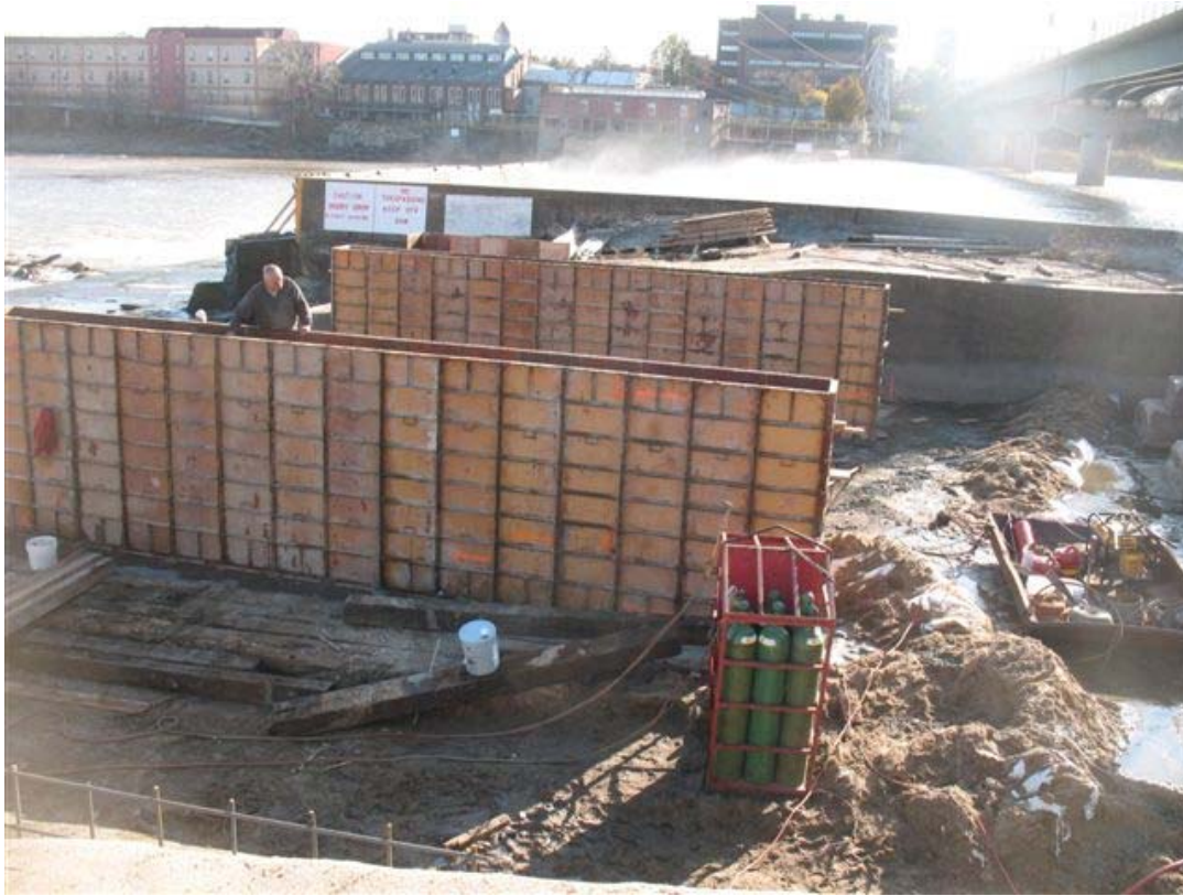
Middle bents of the temporary bridge spanning the spillway under construction.
