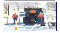
**What Is A Pothole?** While several factors contribute to the creation of potholes, they are distresses in the pavement that can create a failure of the pavement. This failure causes the pavement material to crumble and create a void in the pavement.
