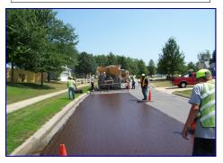
What Is Microsurfacing? Microsurfacing is a preventative street sealing technique that uses a pre-mixed slurry of rock, polymer asphalt binders, cement, and filler materials to seal the entire roadway at a depth of about 3/8th of an inch. It is applied over the top of the pavement.
