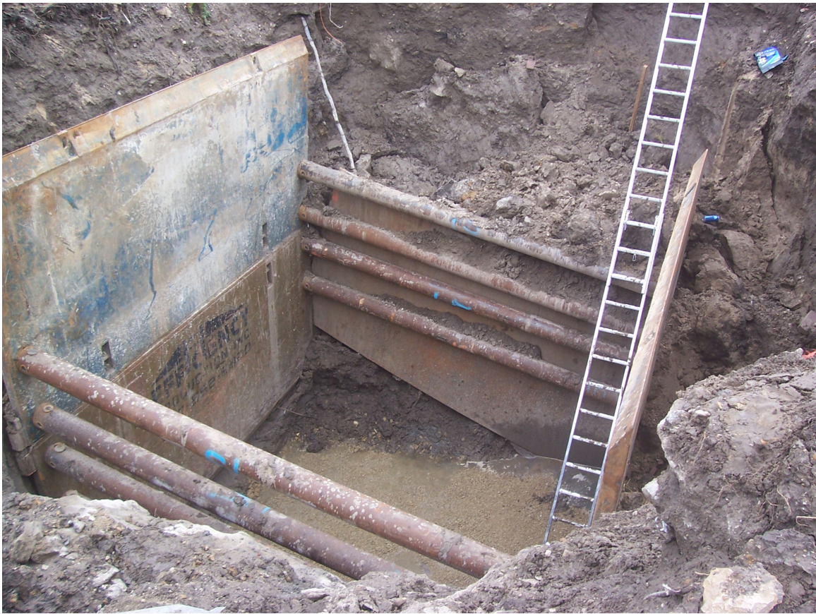
Trench box for storm sewer construction.
