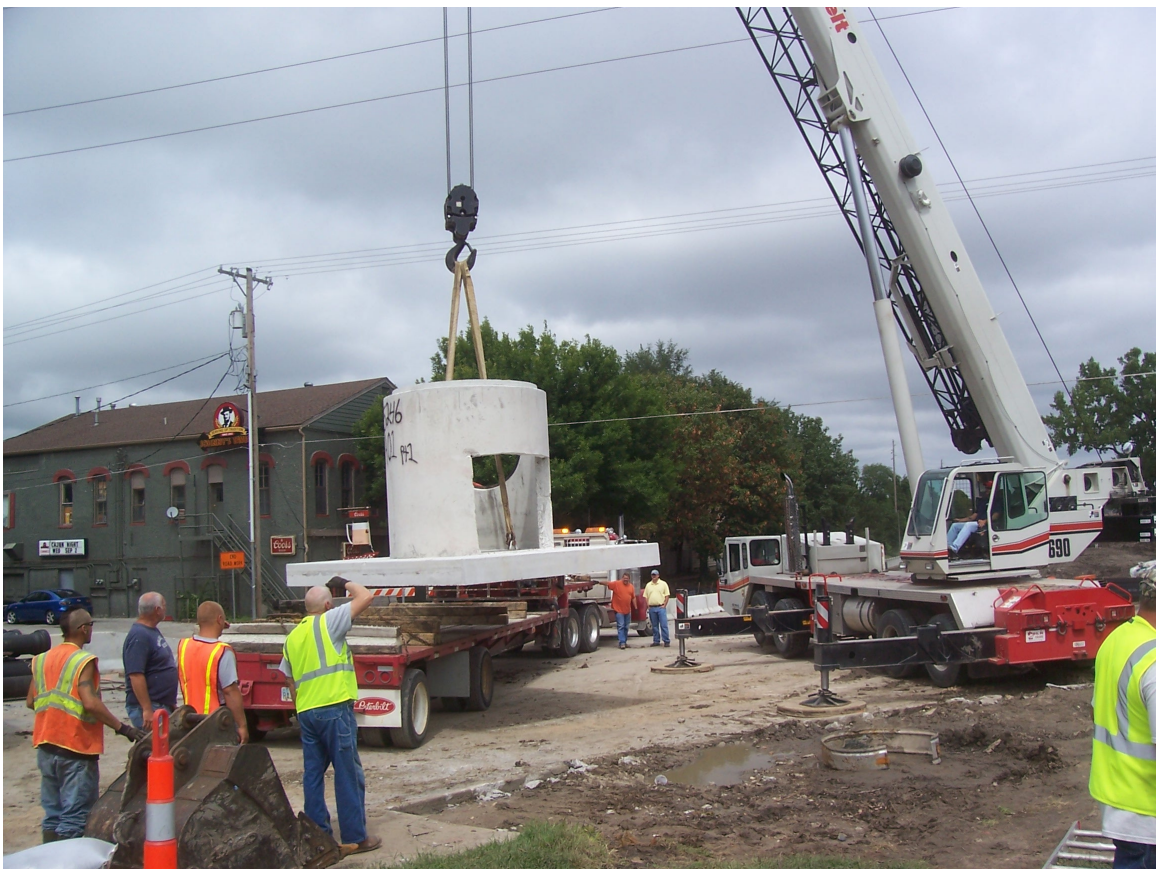
Setting 23000 lbs structure with crane
