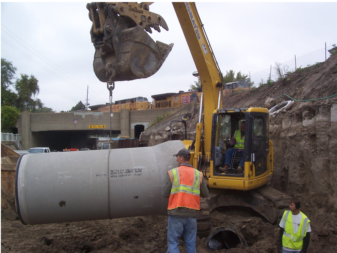
Placing pipe in trench.
