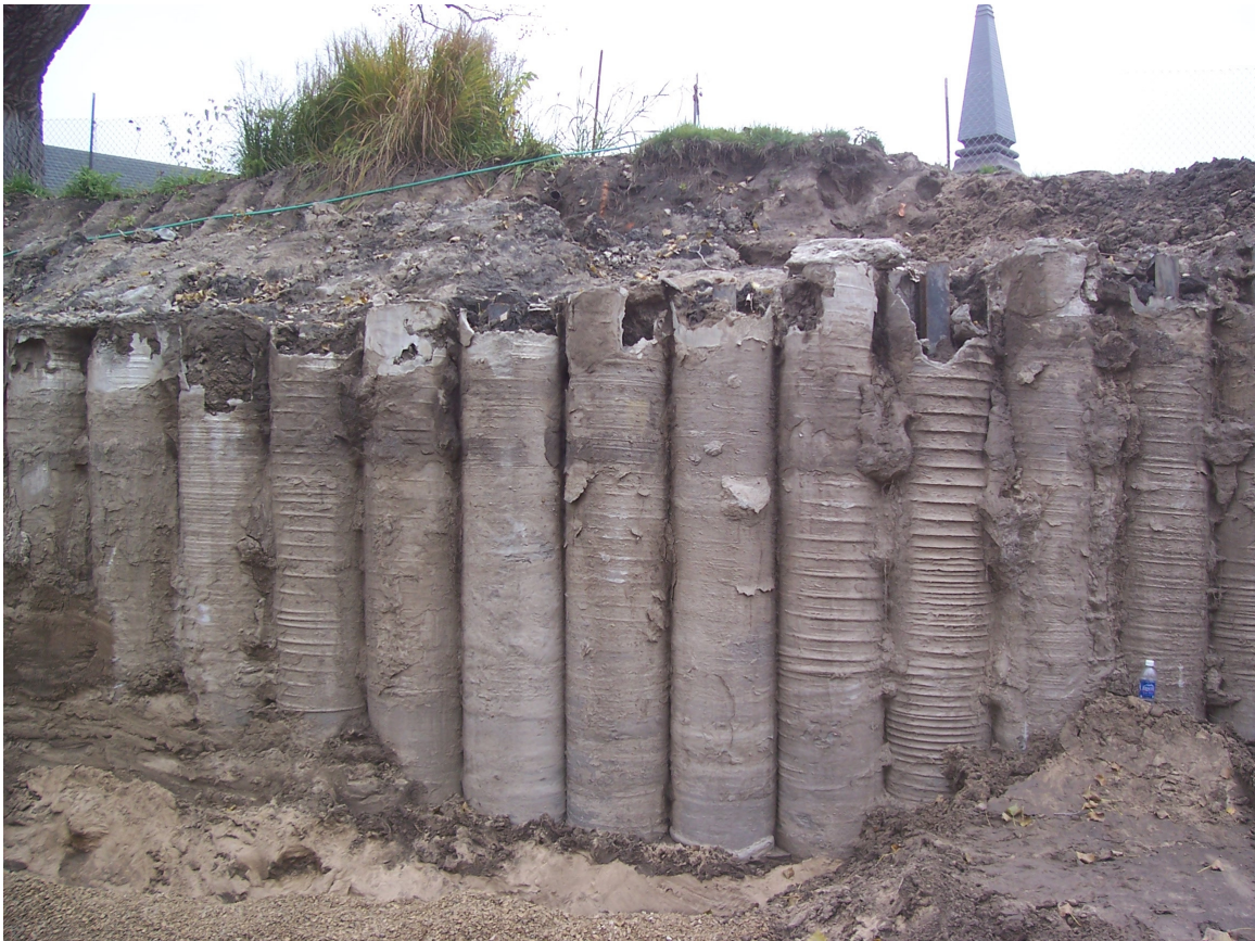
Retention wall along excavation
