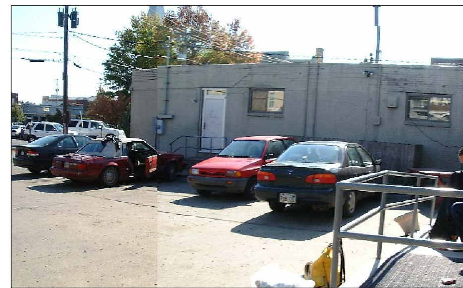
VIEW OF NORTH SIDE OF BUILDING
