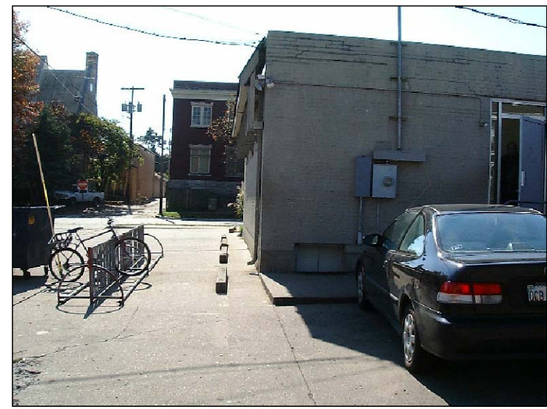
VIEW OF NORTHEAST CORNER
