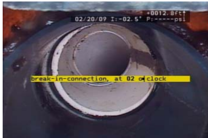
Service connection 2 feet outside of Hobbs Park Manhole
