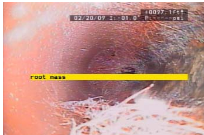
Severe Root Intrusion
