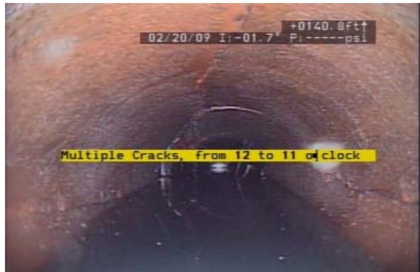
140.8 feet west of manhole/also severe sag in line
