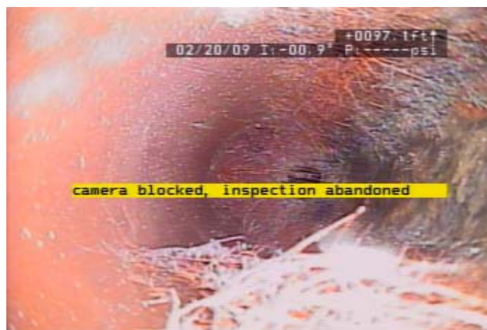
Severe Root Intrusion
