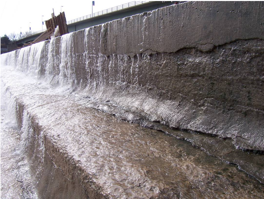
59. Sta 1+25 to south. Eroded shotcrete.
