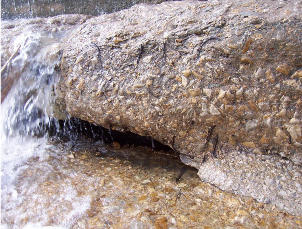
69. Sta 2+95±. Void between lower and middle steps. (See #41, 2007 Report)
