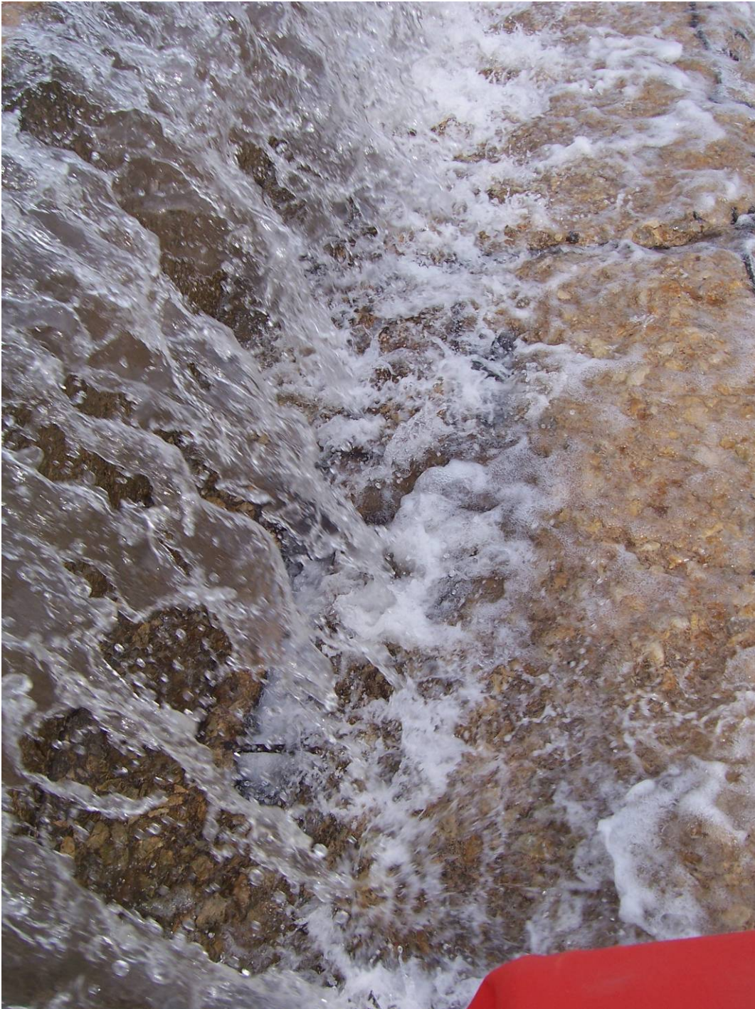
15. Sta 3+90±. Water flowing into eroded concrete with exposed wire mesh in top step. (See #55 & 99, 2007 Report.)
