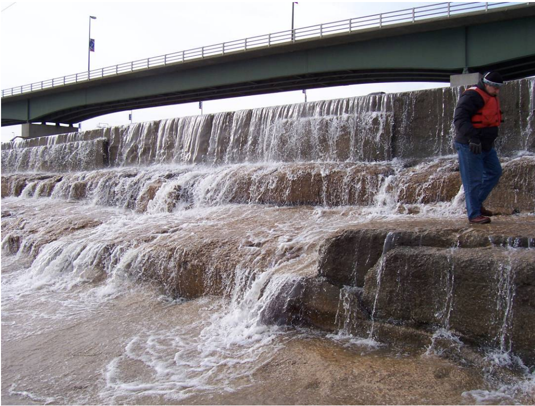
47. Sta 2+40±. Deteriorated steps and exposed joints. (See #27 and 29, 2007 Report.)
