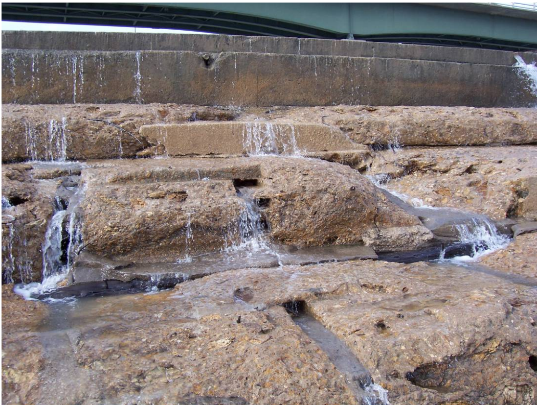
24. Sta 3+40. Eroded timber holes, exposed timber, eroded concrete. (See #45, 46, 47, 2007 Report.)
