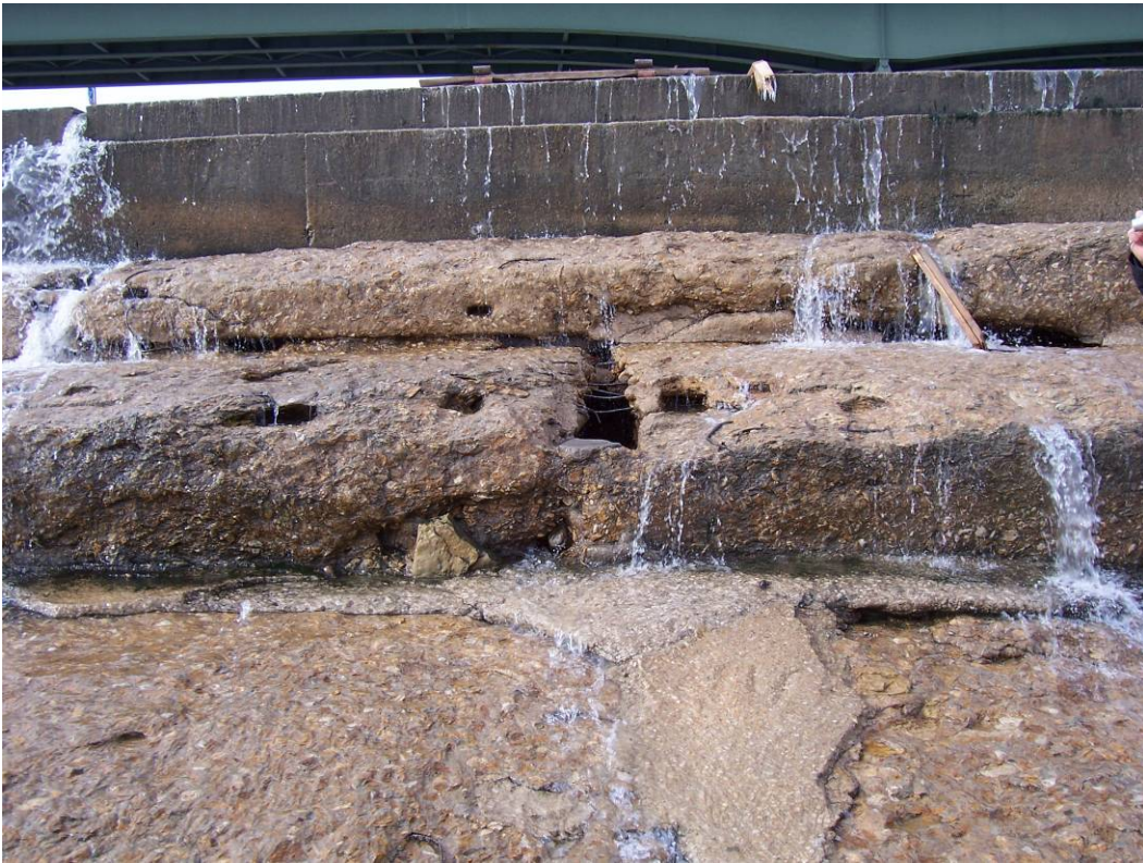
35. Sta 3+00. Exposed and eroded timber holes, exposed rebar, severely deteriorated steps. (See #39-41, 2007 Report.)
