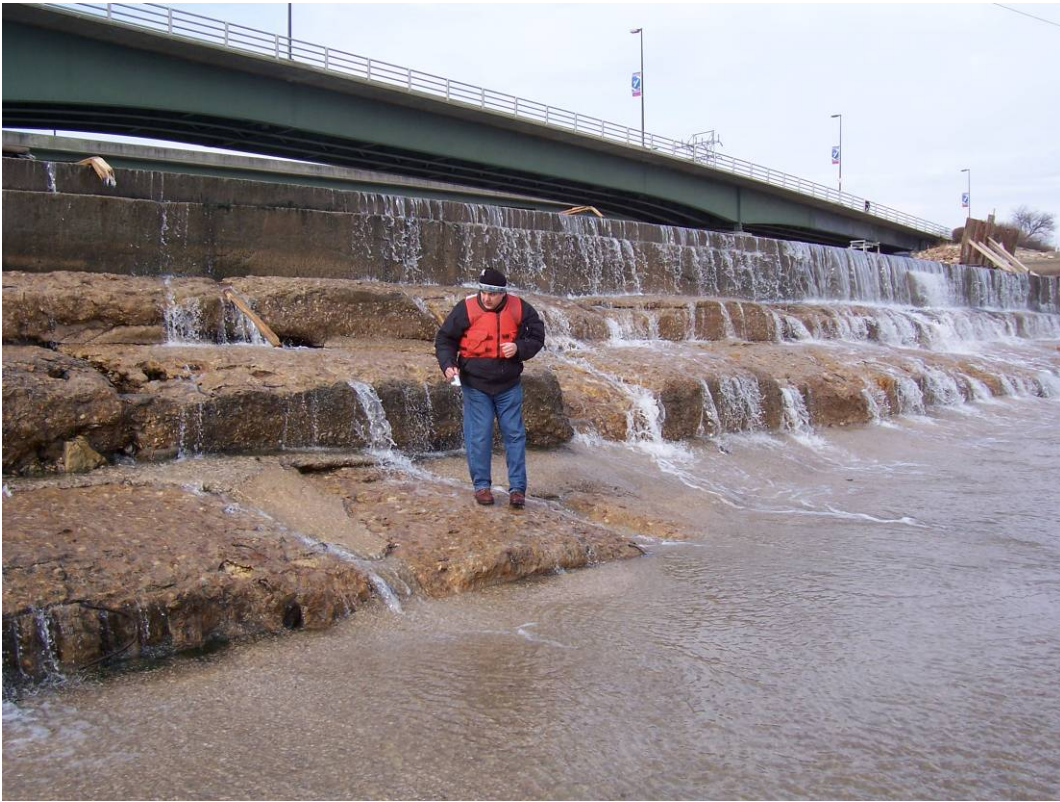
33. Sta 2+50 to Sta 3+60. Exposed and eroded timber holes, exposed rebar, severely deteriorated steps. (See #39-41, 2007 Report.)
