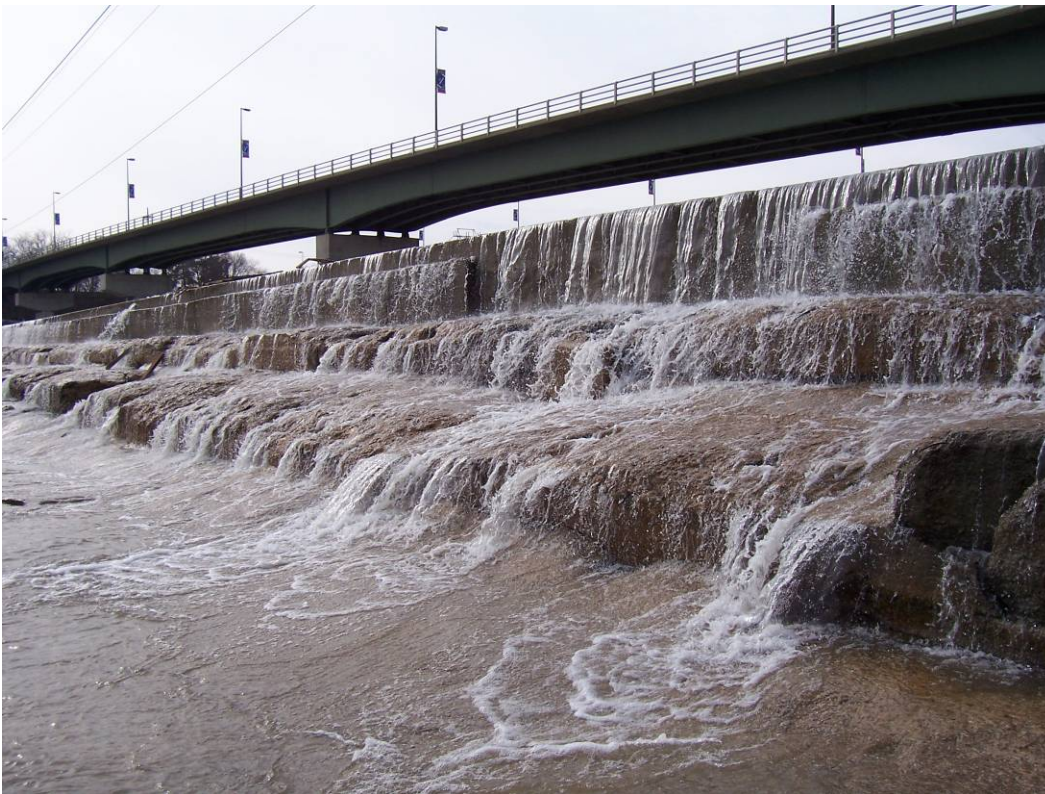
48. Sta 2+40 to 2+80±. Deteriorated steps.
