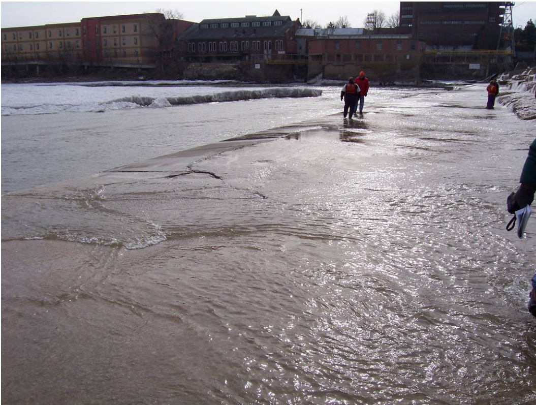
50. Sta 2+40 to Sta 3+00±. Existing crack in apron. No apparent change.
