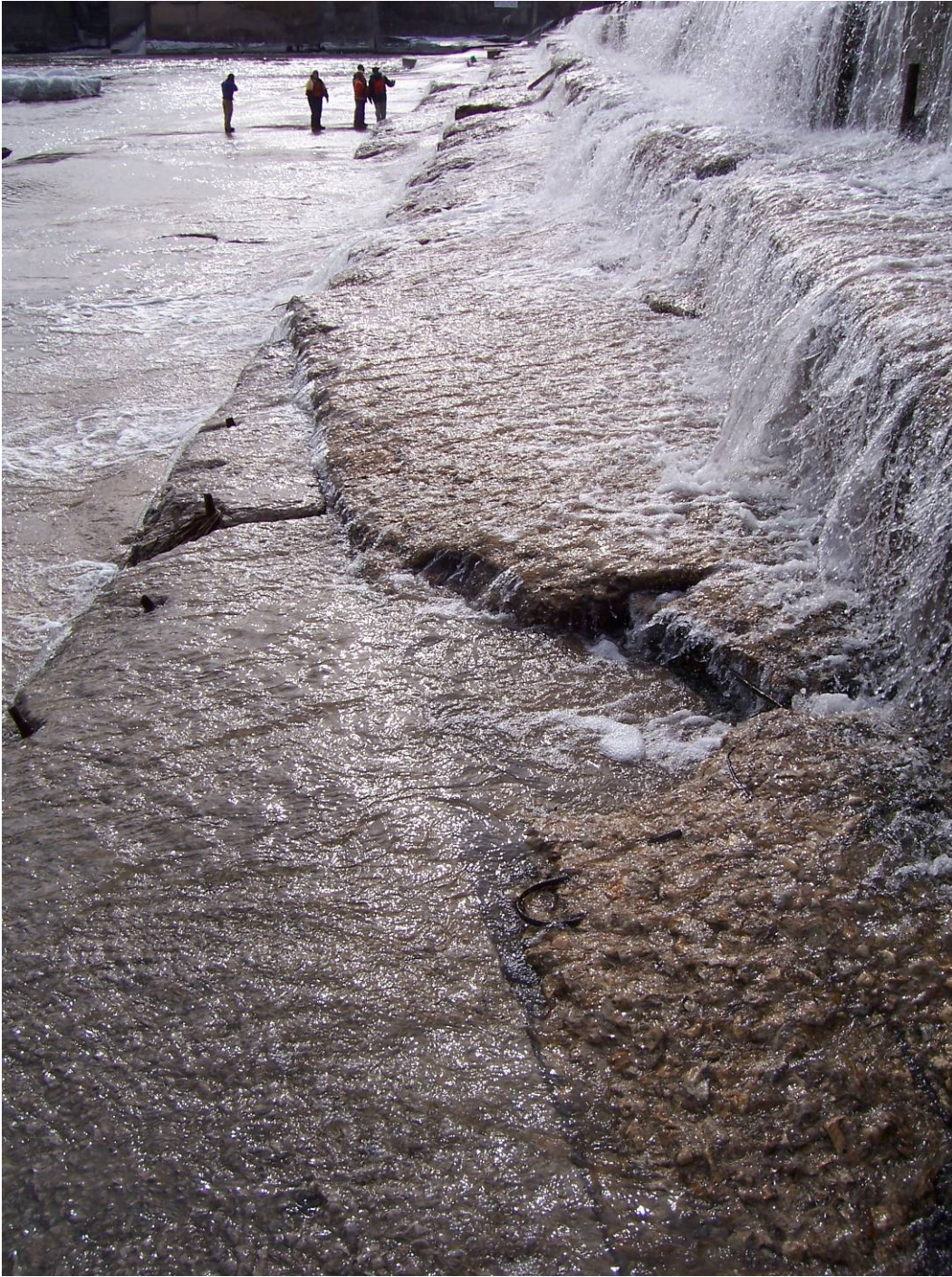
55. Sta 1+90± to south. Separated triangular section in bottom step. Eroded concrete. (See #108, 2007 Report.)
