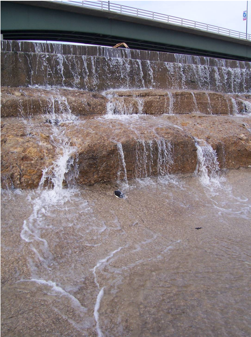
39. Sta 2+75. Exposed joint and cracked middle step crack in bottom step, weep hole. (See #36, 2007 Report.)
