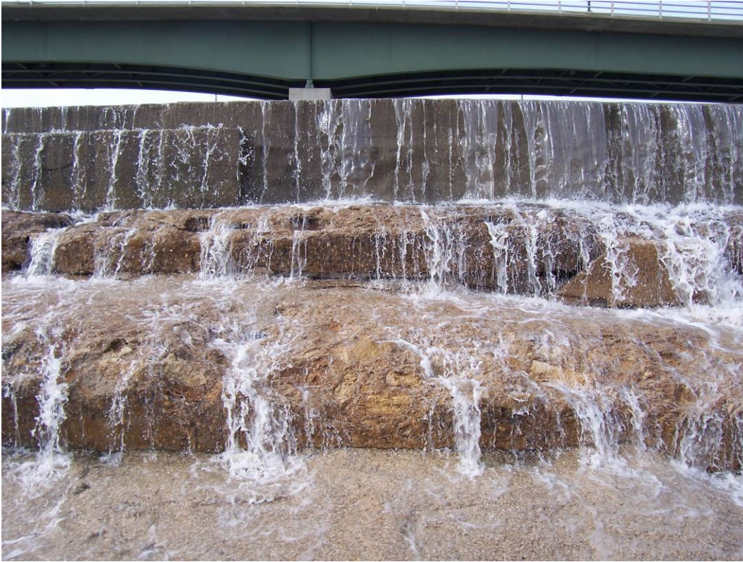
43. Sta 2+50. Exposed joints between steps eroded concrete. (See #30-32, 2007 Report.)
