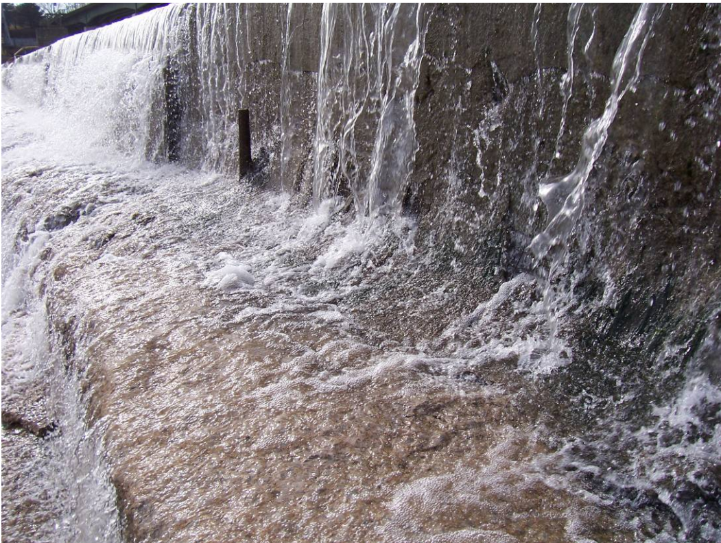
54. Sta 2+40± to south. Exposed wire fabric and eroded shotcrete. (See #29, 2007 Report.)
