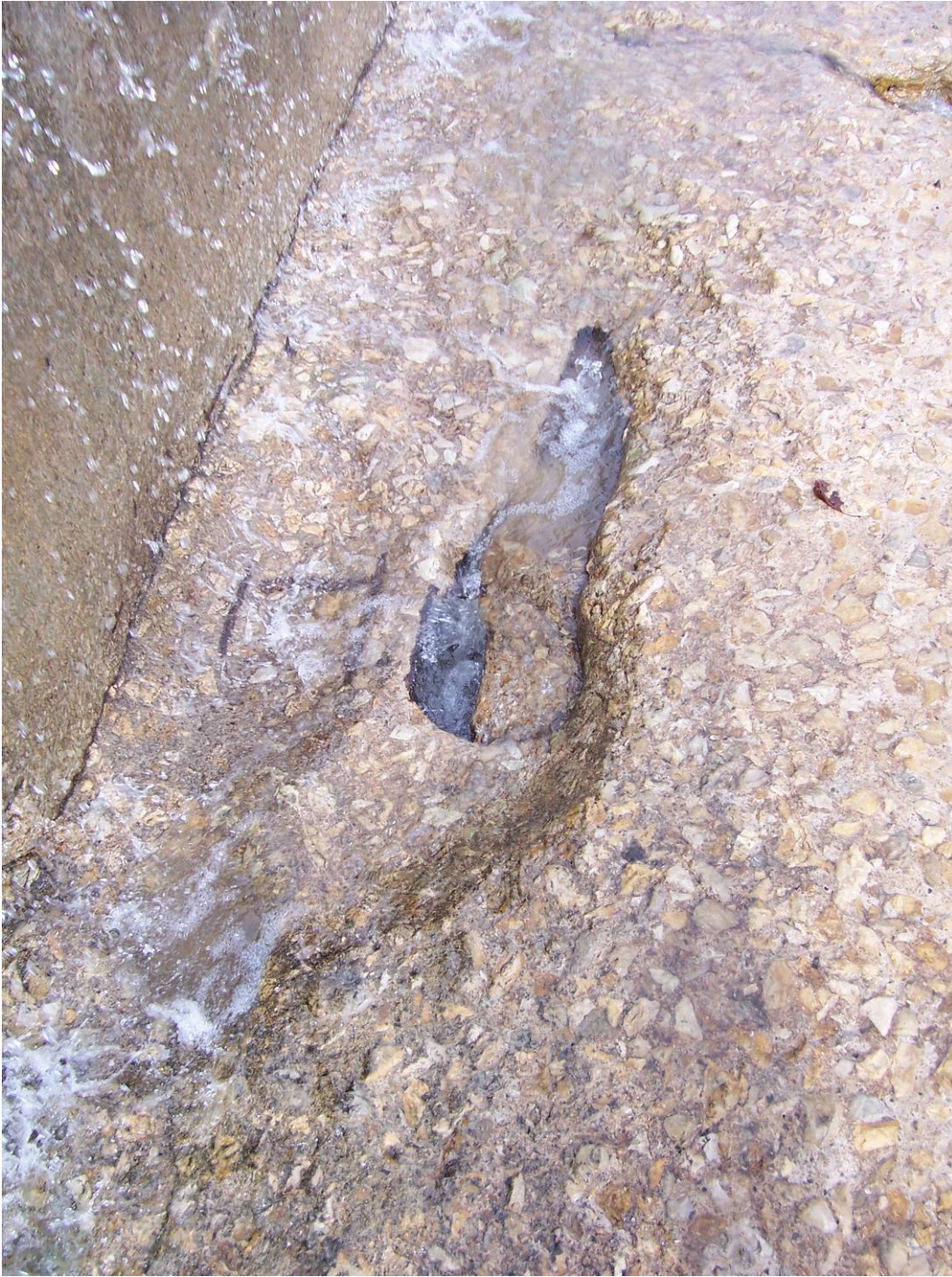
14. Sta 4+40. Water draining into eroded concrete and exposed timber hole. (See #98, 2007 Report.)
