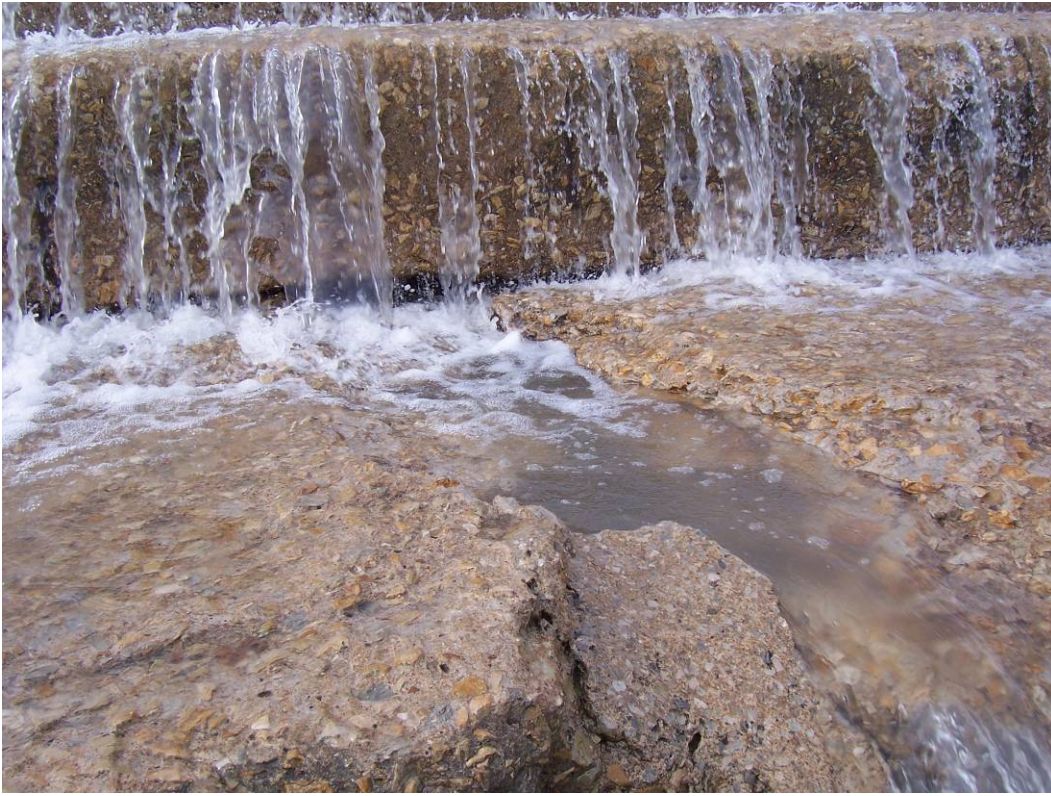
16. Sta 3+90±. Location of prior significant leak. 4 ft deep hole in second step. (See #50, 52, 53, 54, 56, 58, 100, 102 in 2007 Report.)
