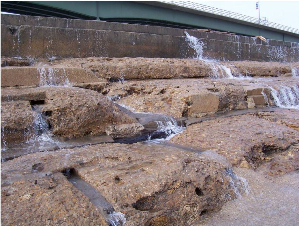
25. Sta 3+25. Eroded timber holes, exposed timber, eroded concrete. (See #46, 47, 2007 Report.)
