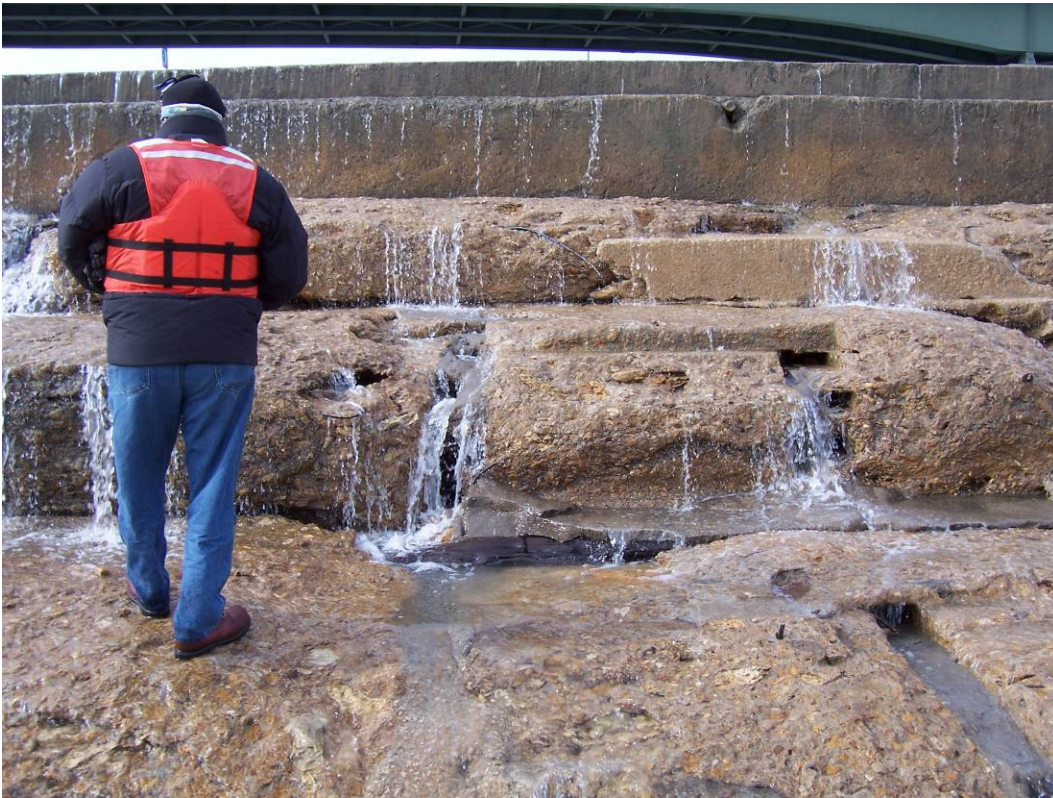
23. Sta 3+40. Eroded timber holes, exposed timber, eroded concrete. (See #45, 46, 47, 2007 Report.)
