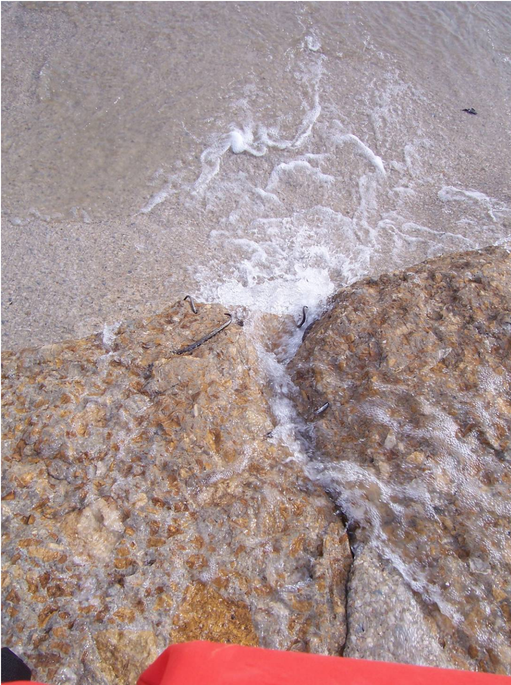
68. Sta 2+75±. Exposed, eroded reinforcing steel on first step. (See #36, 2007 Report.).
