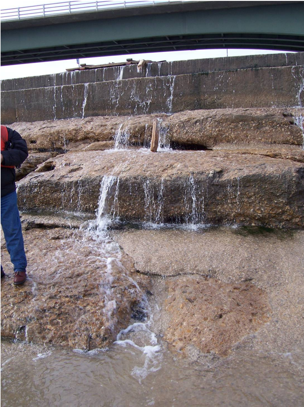
37. Sta 2+95. Exposed joint between 2 nd & 3 rd steps, severely deteriorated lower step. (See #41, 2007 Report.)
