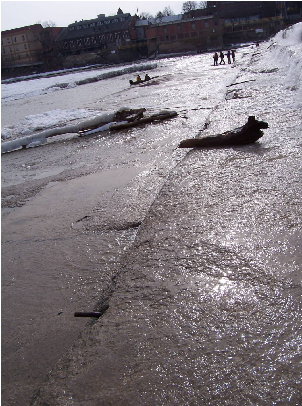
60. Sta 1+25 to south. Eroded concrete. Exposed bar. (See #17 & 19, 2007 Report.)
