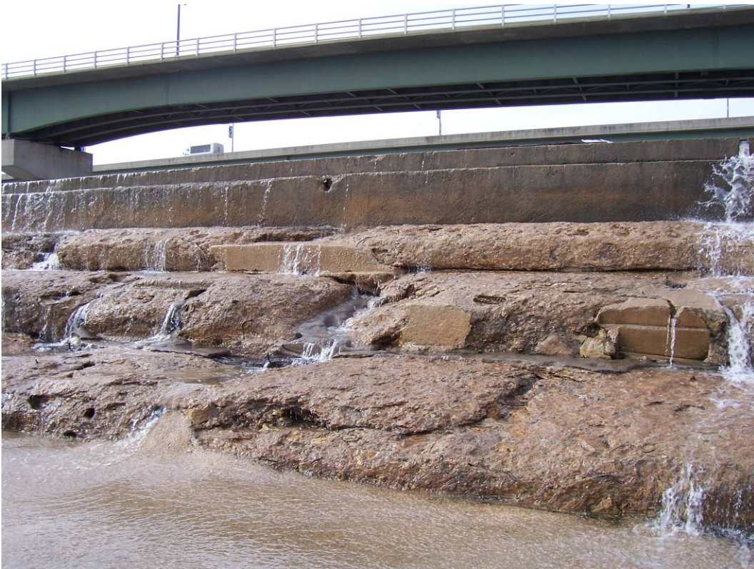
30. Sta 3+30. Severely deteriorated concrete. Eroded timber holes.
