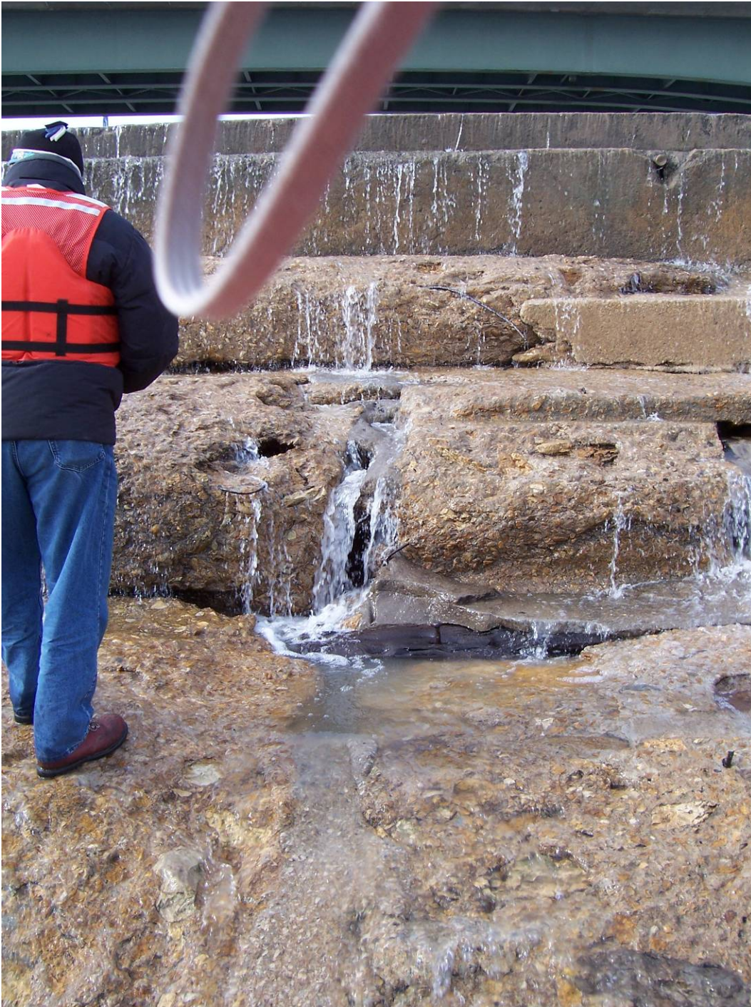
22. Sta 3+40. Eroded timber holes, exposed timber, eroded concrete. (See #46, 47, 2007 Report.)
