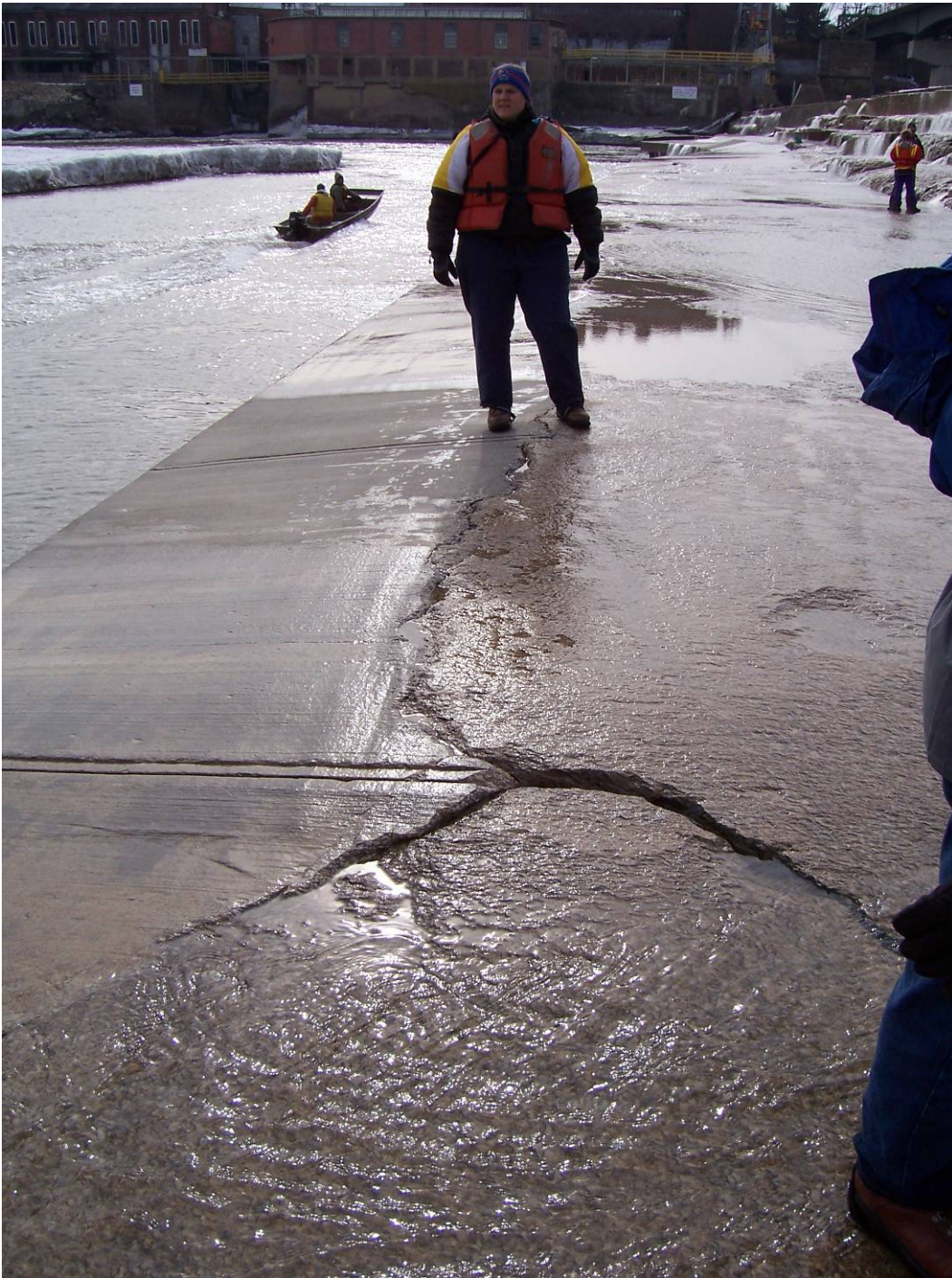
46. Sta 2+70±. Existing crack in apron to new apron interface. No apparent change.
