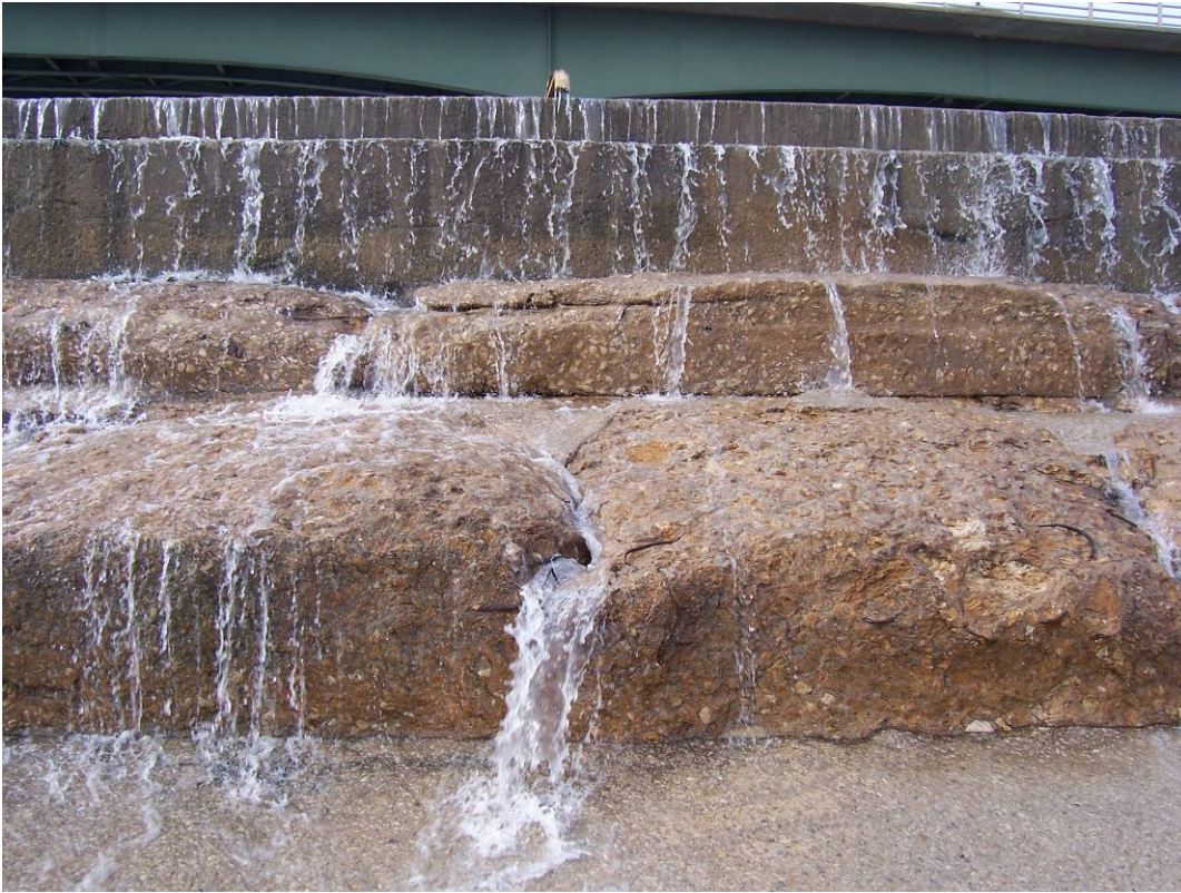
41. Sta 2+75. Exposed joint and cracked middle step crack in bottom step, weep hole. Additional erosion since 2006. (See #36, 2007 Report.)
