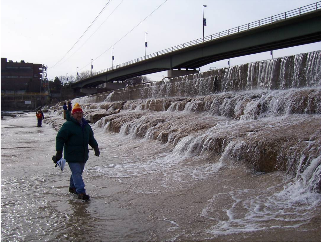
49. Sta 2+50 to Sta 3+00±. Deteriorated steps.
