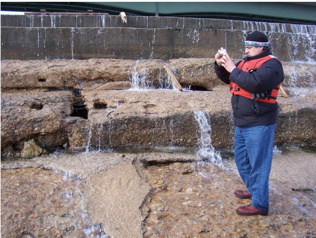
36. Sta 3+00. Exposed and eroded timber holes, exposed rebar, severely deteriorated steps. (See #39-41, 2007 Report.)
