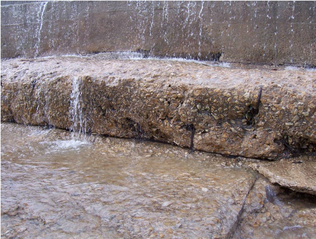
18. Sta 4+25. Deteriorated joint & exposed rebar at top of bottom step. (See #57 in 2007 Report.)
