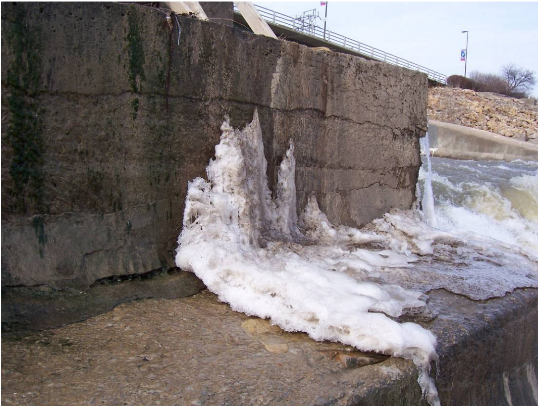
58. Sta 1+25 to northwest. Eroded shotcrete. (See #18, 2007 Report.)
