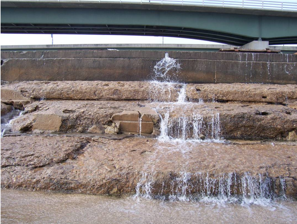
31. Sta 3+25. Severely deteriorated steps. (See #42, 2007 Report.)
