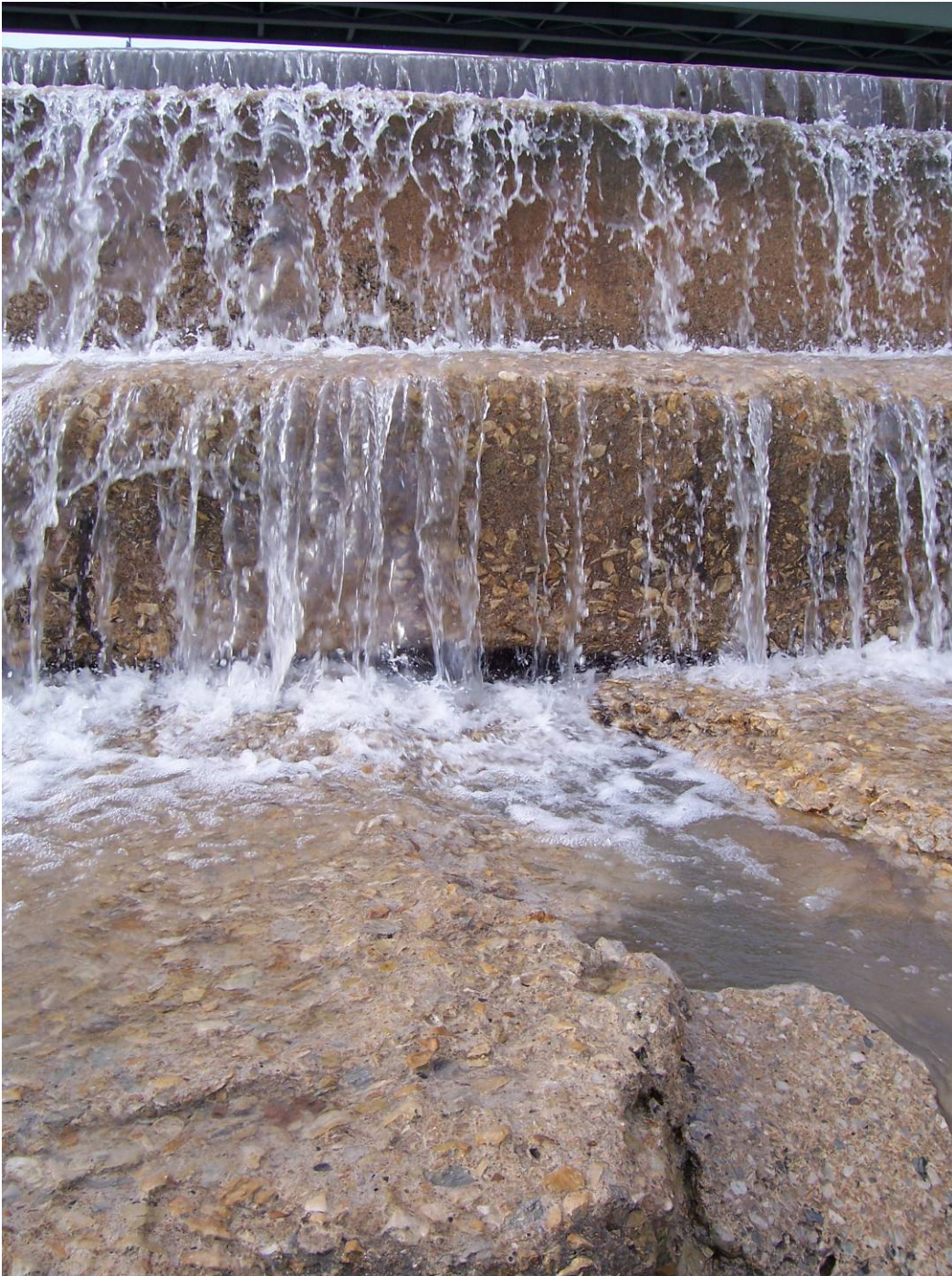
17. Sta 3+90±. Location of prior significant leak. 4 ft deep hole in second step. (See #50, 52, 53, 54, 56, 58, 100, 102 in 2007 Report.)
