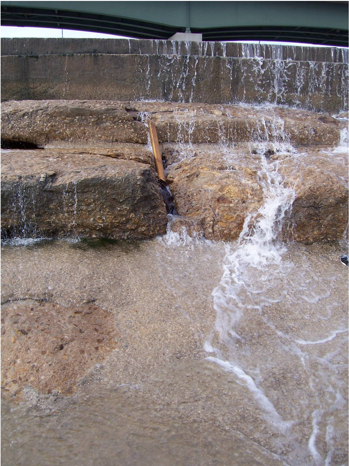
38. Sta 2+80. Exposed timber and eroded concrete. Crack in bottom step. (See #37 and 38, 2007 Report.)
