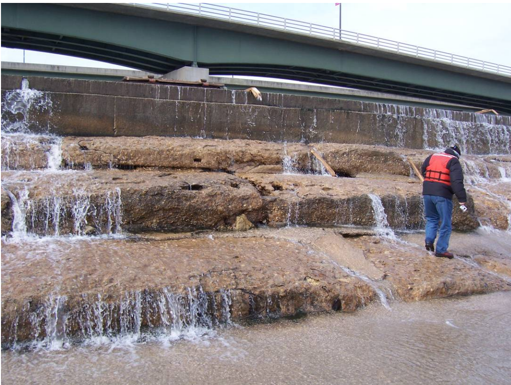
32. Sta 3+00 to Sta 3+20. Exposed and eroded timber holes, exposed rebar, severely deteriorated steps. (See #39-41, 2007 Report.)
