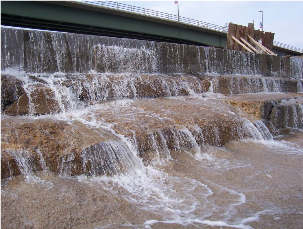
45. Sta 2+40. Deteriorated concrete steps. Exposed joints. (See #29, 2007 Report.)
