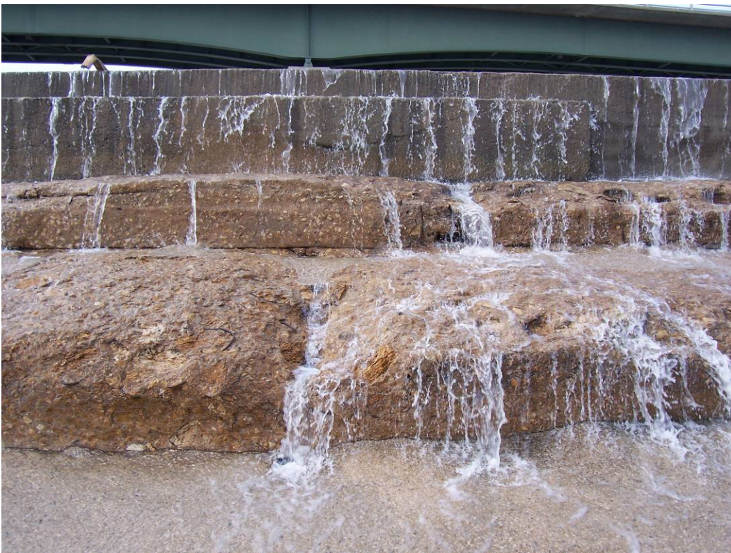
42. Sta 2+65. Eroded concrete and exposed timber hole. Additional erosion since 2006. (See #31, 33, 34 & 35, 2007 Report.)
