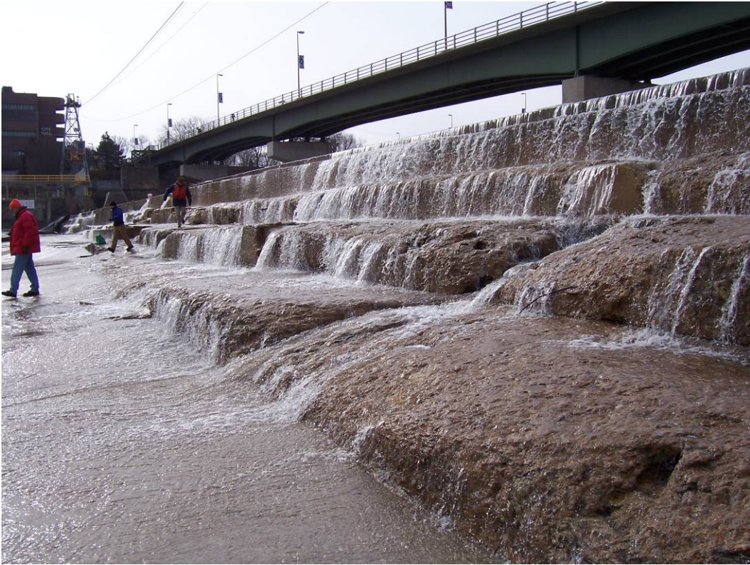
29. Sta 3+60 to Sta 4+00. Severely deteriorated concrete. Eroded timber holes.
