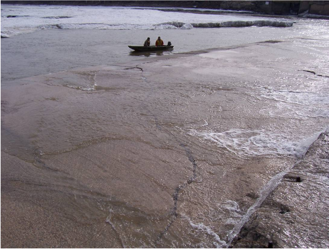
51. Sta 2+40 to Sta 2+80. Existing crack in apron. No apparent change.
