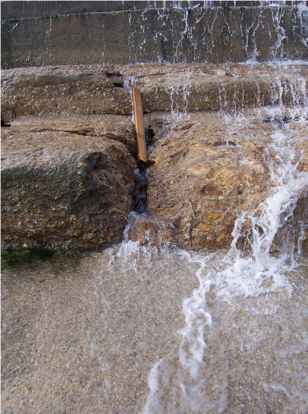
40. Sta 2+80. Exposed timber and eroded concrete. Crack in bottom step. (See #37 and 38, 2007 Report.)
