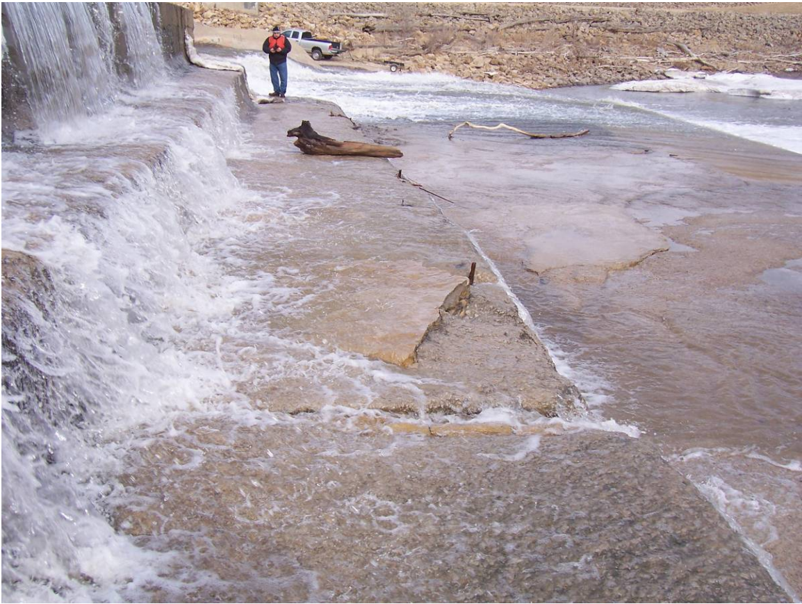
56. Sta 1+80± to north. Eroded concrete step.
