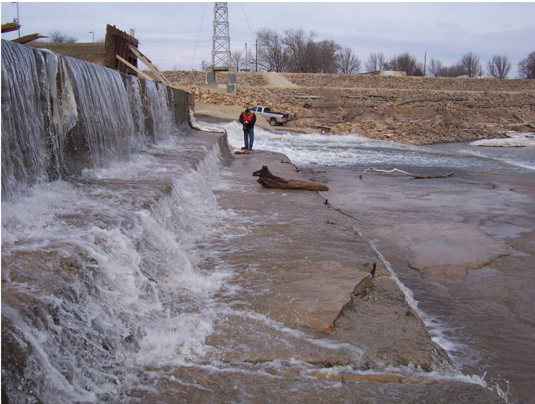
57. Sta 1+80± to north. Eroded concrete step.
