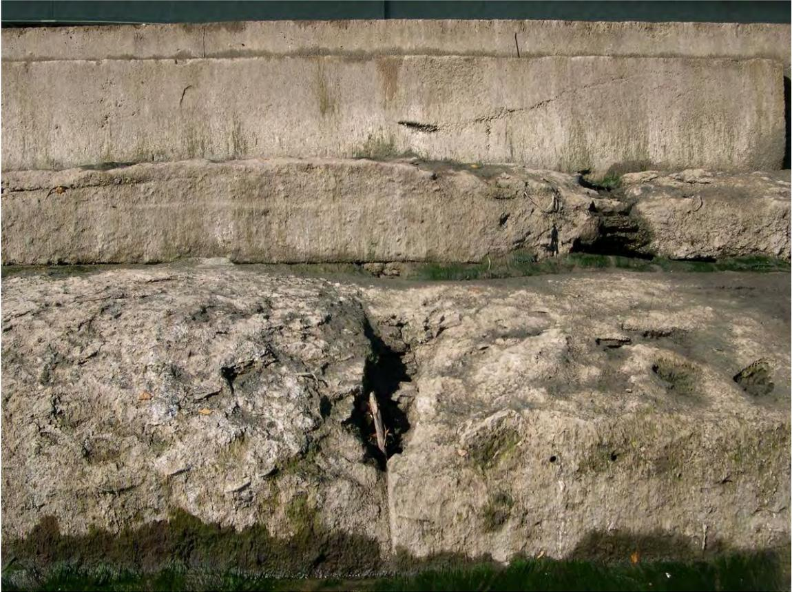
130. Sta 2+65. Exposed timber holes and rebar. Eroded concrete. Exposed joint between steps.
