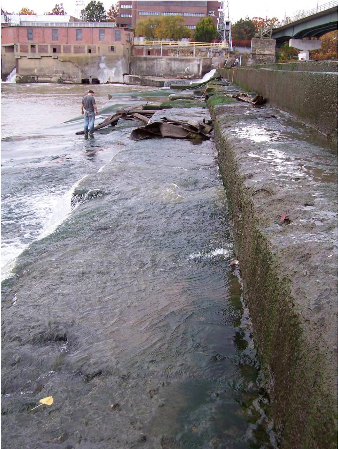
54. Sta 3+90. Looking south. Main flow point through dam. 4 ft deep hole at flow point.
