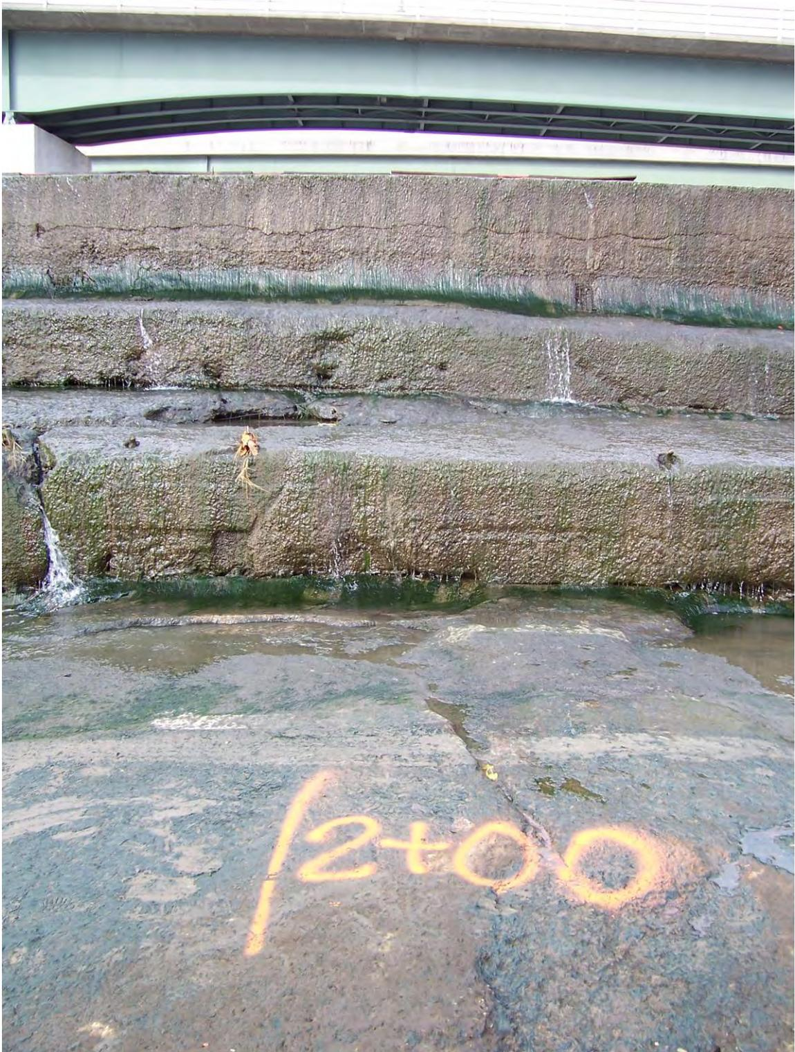
24. Sta 2+00. Eroded concrete on top of bottom step. Exposed joints at bottom of steps. Beginning of separated triangular section in bottom step.
