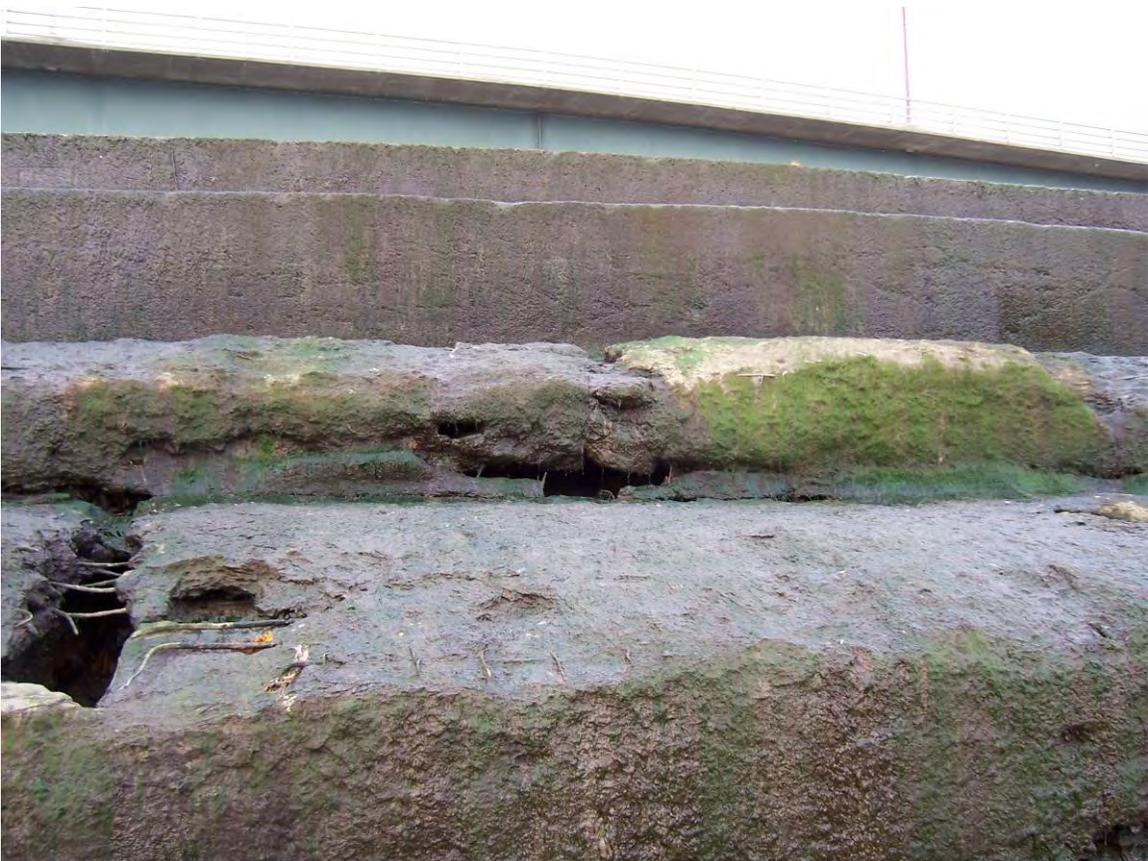
41. Sta 3+00. Eroded timber hole with exposed rebar. Exposed joint between steps.
