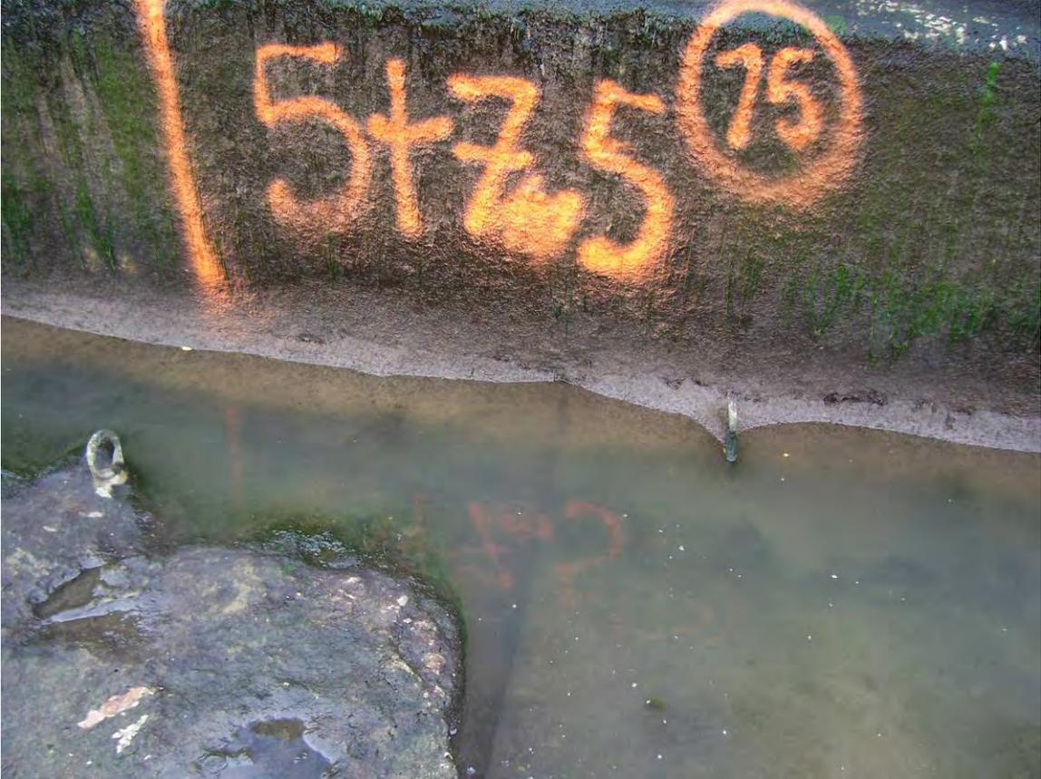
73. Sta 5+75. Eroded shotcrete. Depression with exposed spikes and tie-rings.
