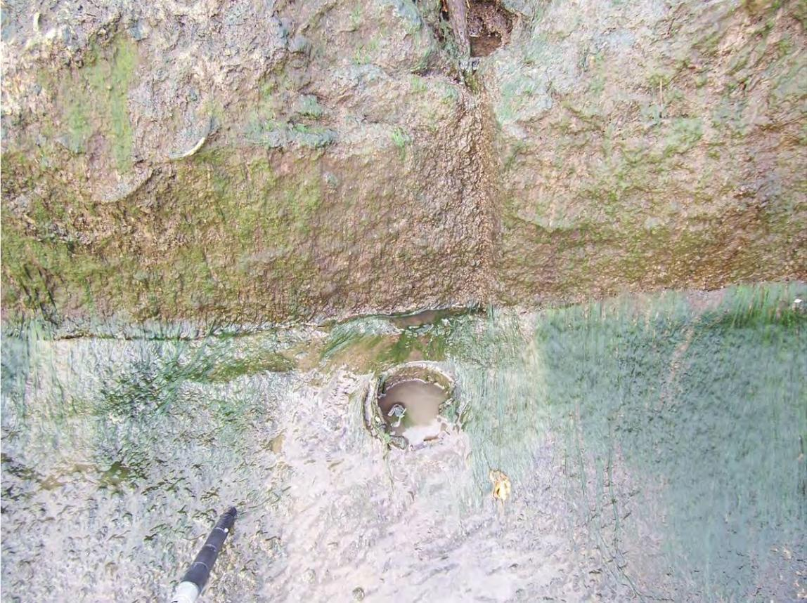
34. Sta 2+65±. Exposed eroded timber at top of bottom step. Cast-In-Place weep hole at bottom of bottom step.
