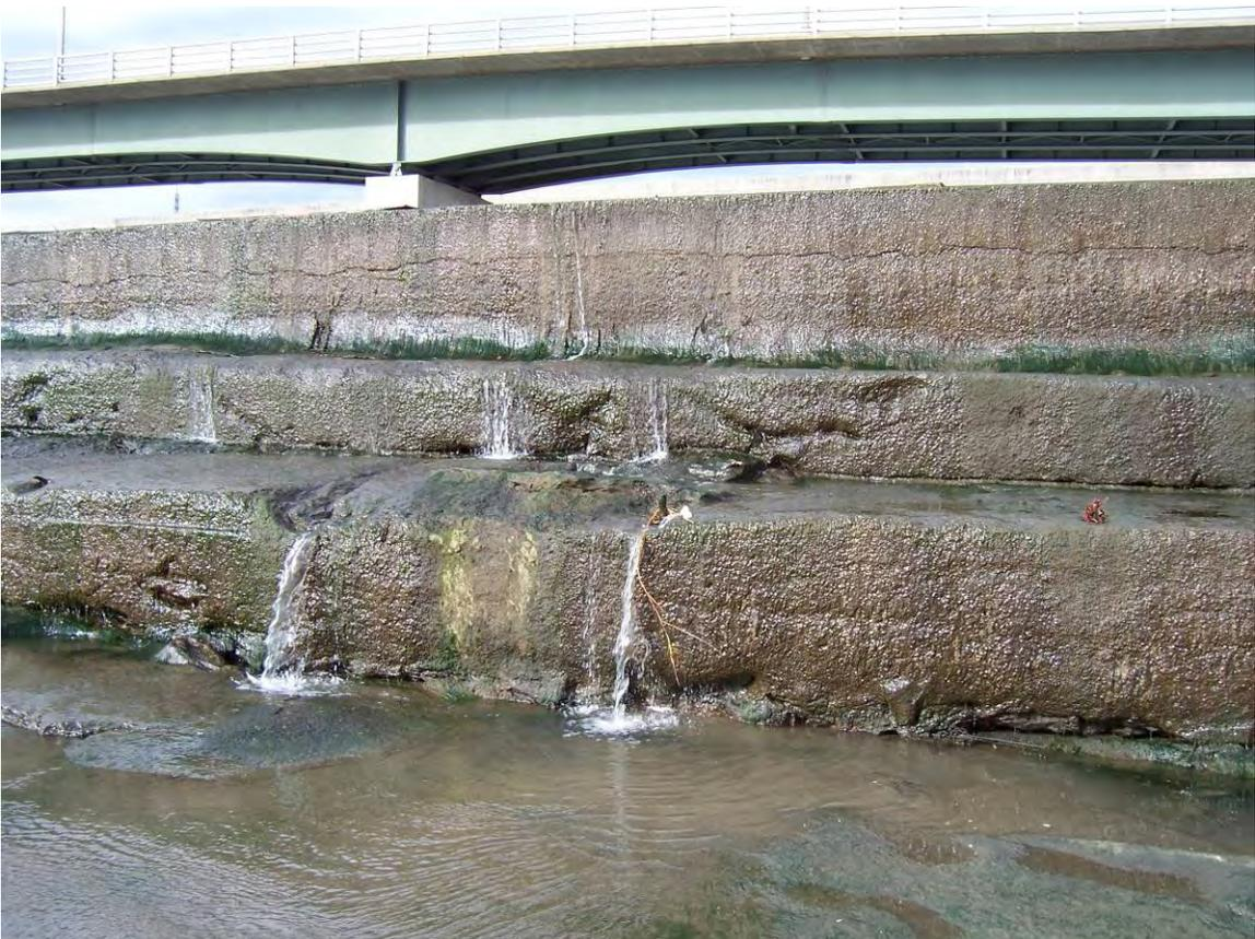
22. Sta 1+80. Eroded bottom step. Depression with 2 ft deep hole at bottom step. Eroded shotcrete.
