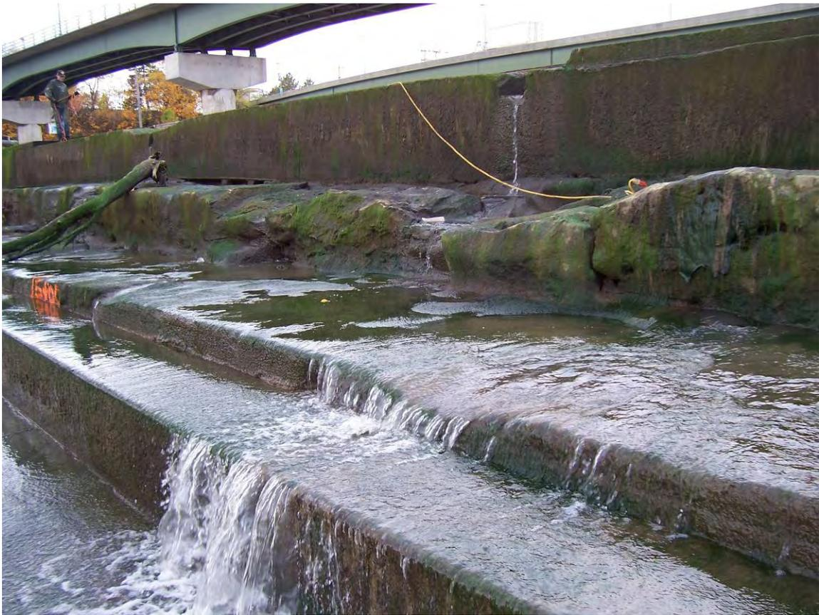
63. Sta 4+75 to 5+00. Severely eroded top step with flow through joint in step.
