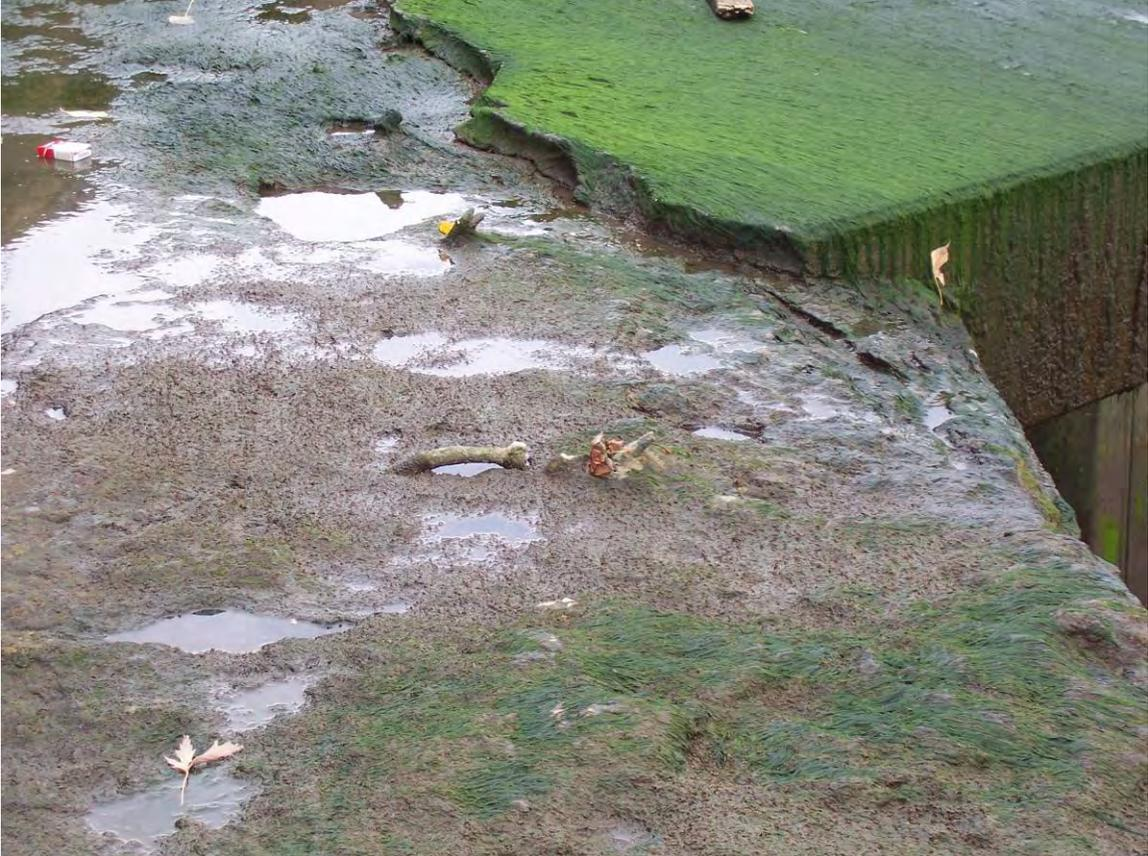
76. Sta 5+75 to 5+60 North. Eroded portion of new apron. Exposed spike in old apron.
