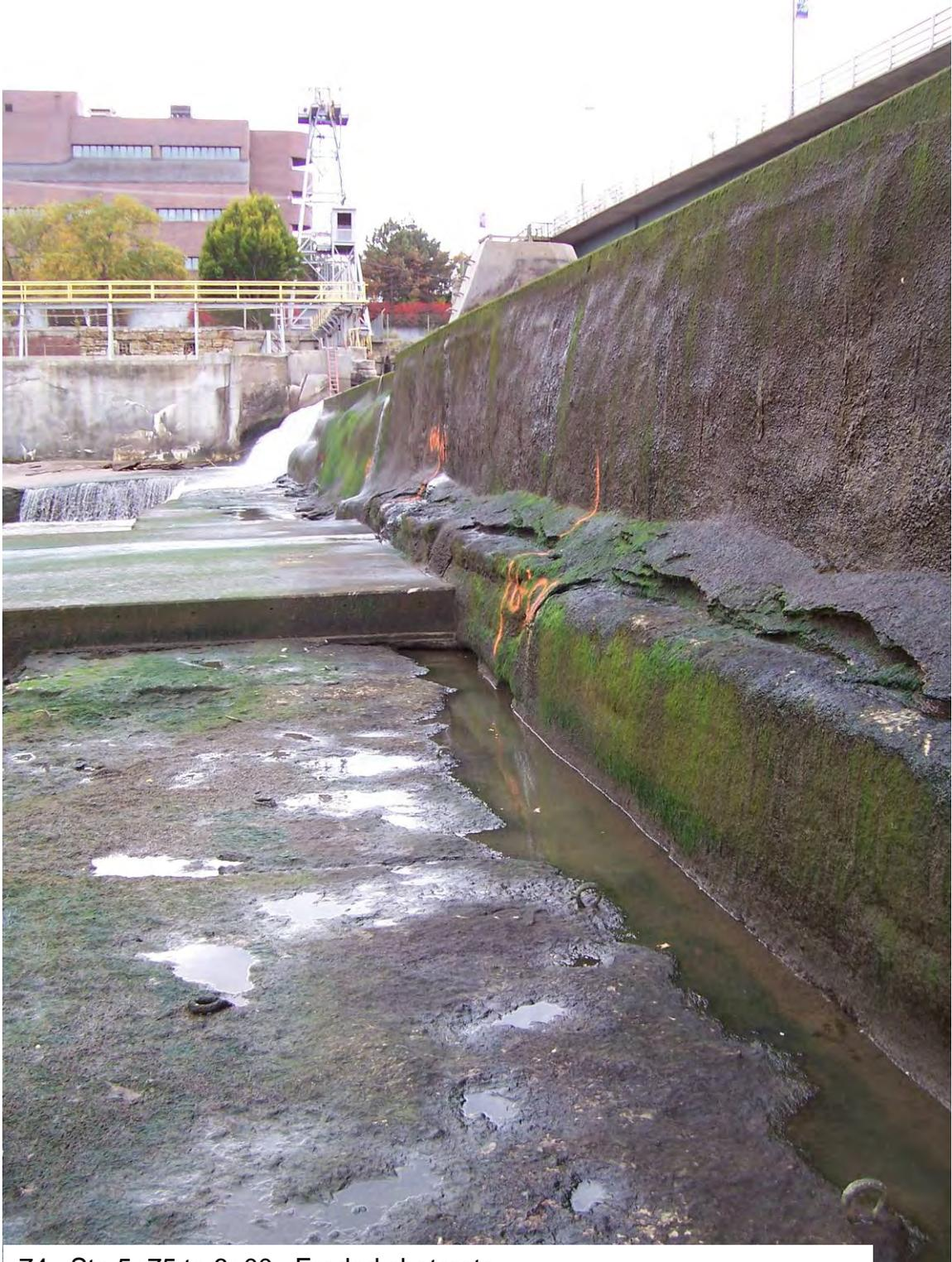
74. Sta 5+75 to 6+00. Eroded shotcrete.
