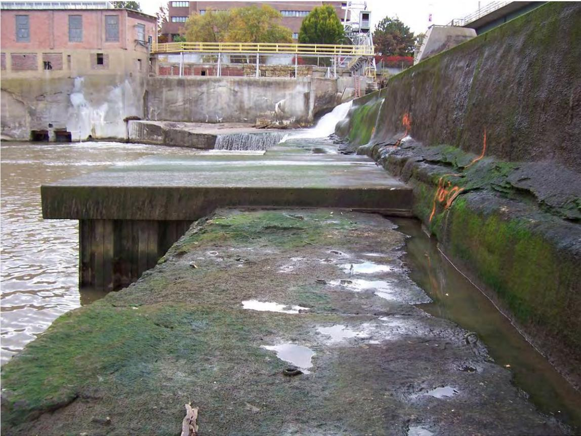
75. Sta 5+75 to Sta 6+00 South. Eroded shotcrete. Short section of piling and new apron.
