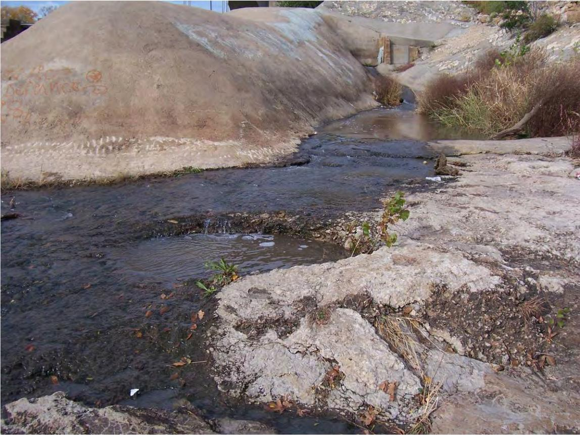
6. Sta 0+25±. Storm drainage flume north of spillway, eroded concrete
