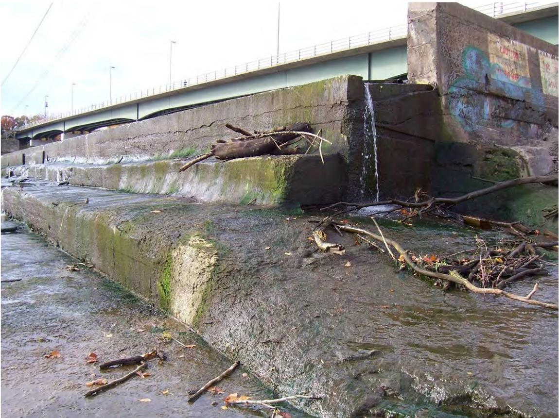
17. Sta 1+25. Eroded concrete at north end of dam.
