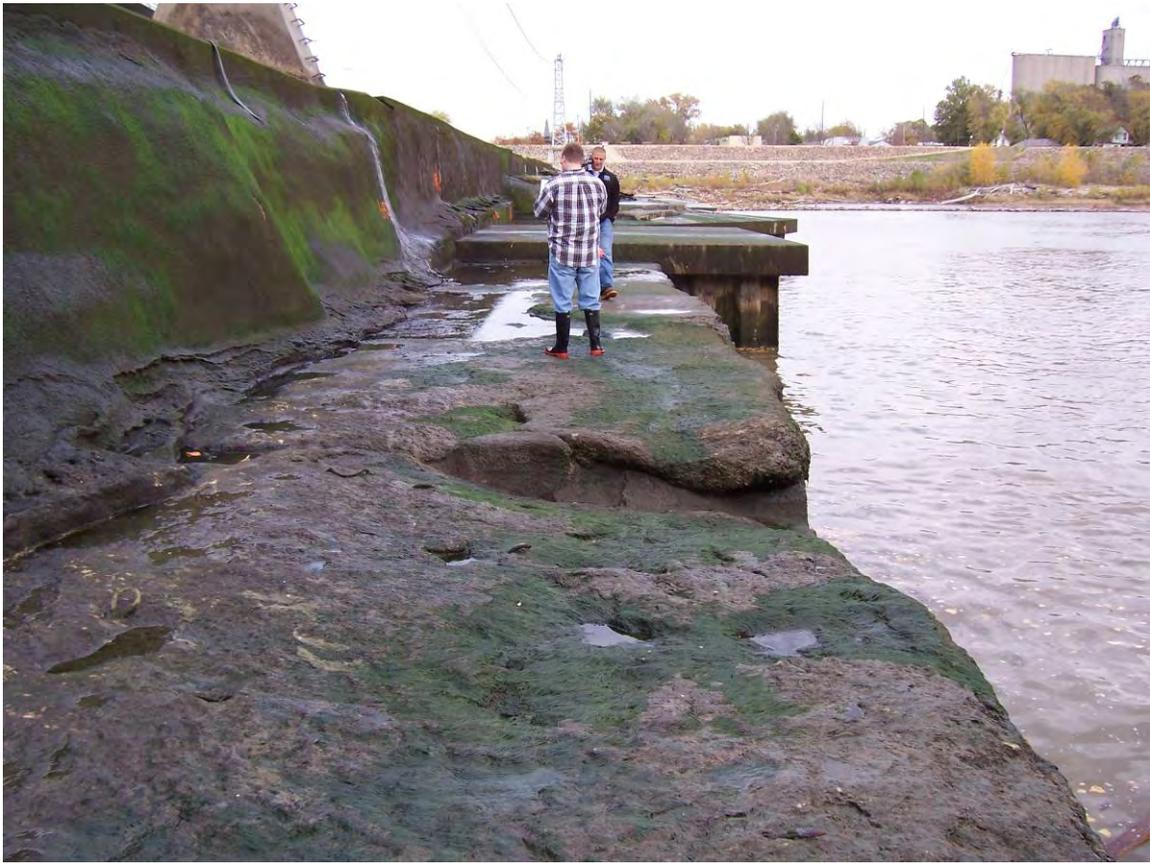
88. Sta 6+80 to north. Severely eroded apron and shotcrete.
