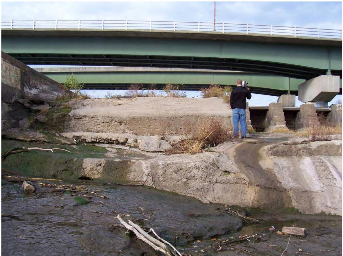
15. Sta 0+00. Eroded concrete and exposed joints in spillway.
