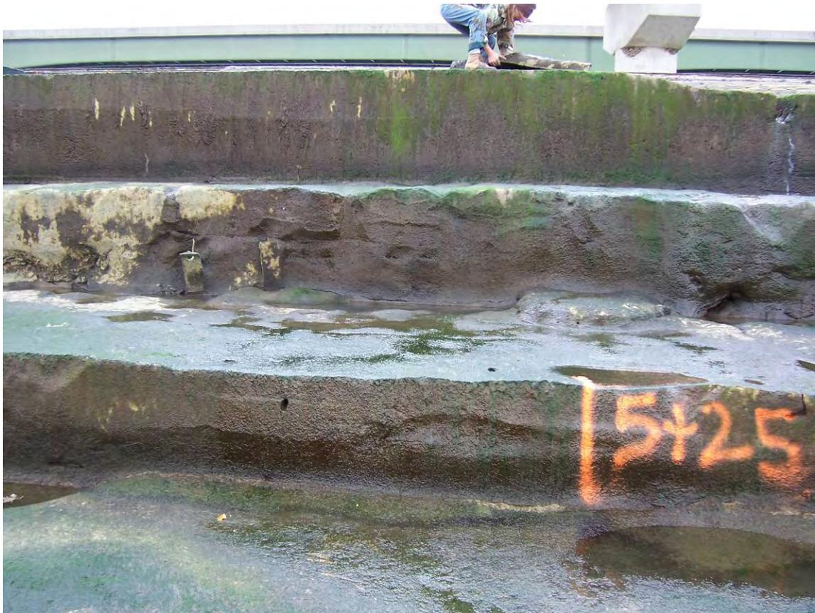
67. Sta 5+25 to 5+35. Exposed I-beam piling at Sta 5+35. Eroded shotcrete exposed joint at step.
