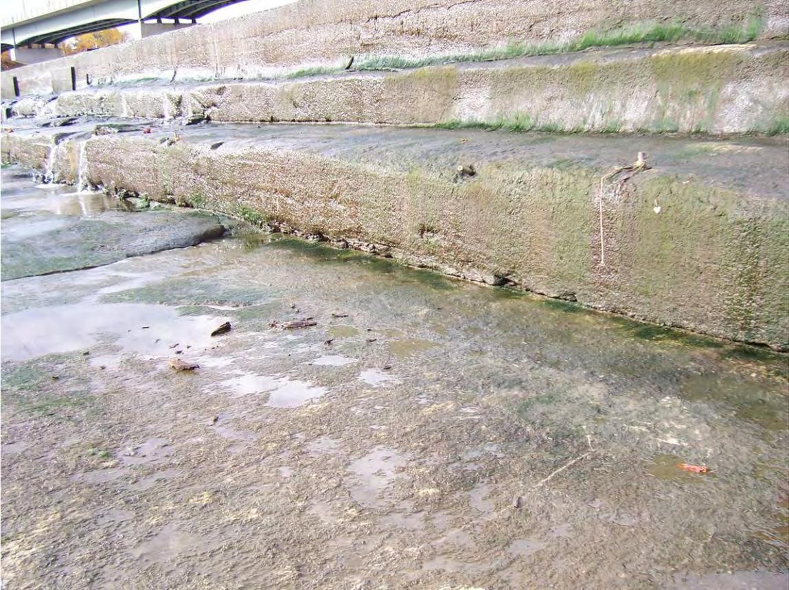
19. Sta 1+25 to 1+50. Exposed joints at bottom of dam steps. Eroded shotcrete at top step.
