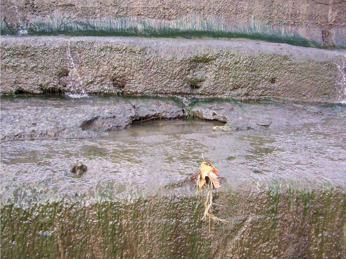
25. Sta 2+05. Top of bottom step. Eroded concrete with exposed reinforcing mesh. Exposed joint between 2<sup>nd</sup> and 1<sup>st</sup> step. Eroded shotcrete with exposed mesh on top step.
