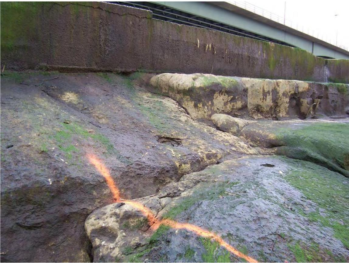
71. Sta 5+50. South end of steps. Eroded concrete exposed joints.
