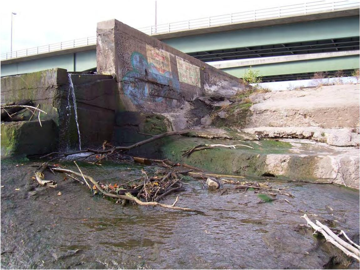
16. Sta 1+10. North wall of dam. Eroded concrete and exposed joints in spillway.
