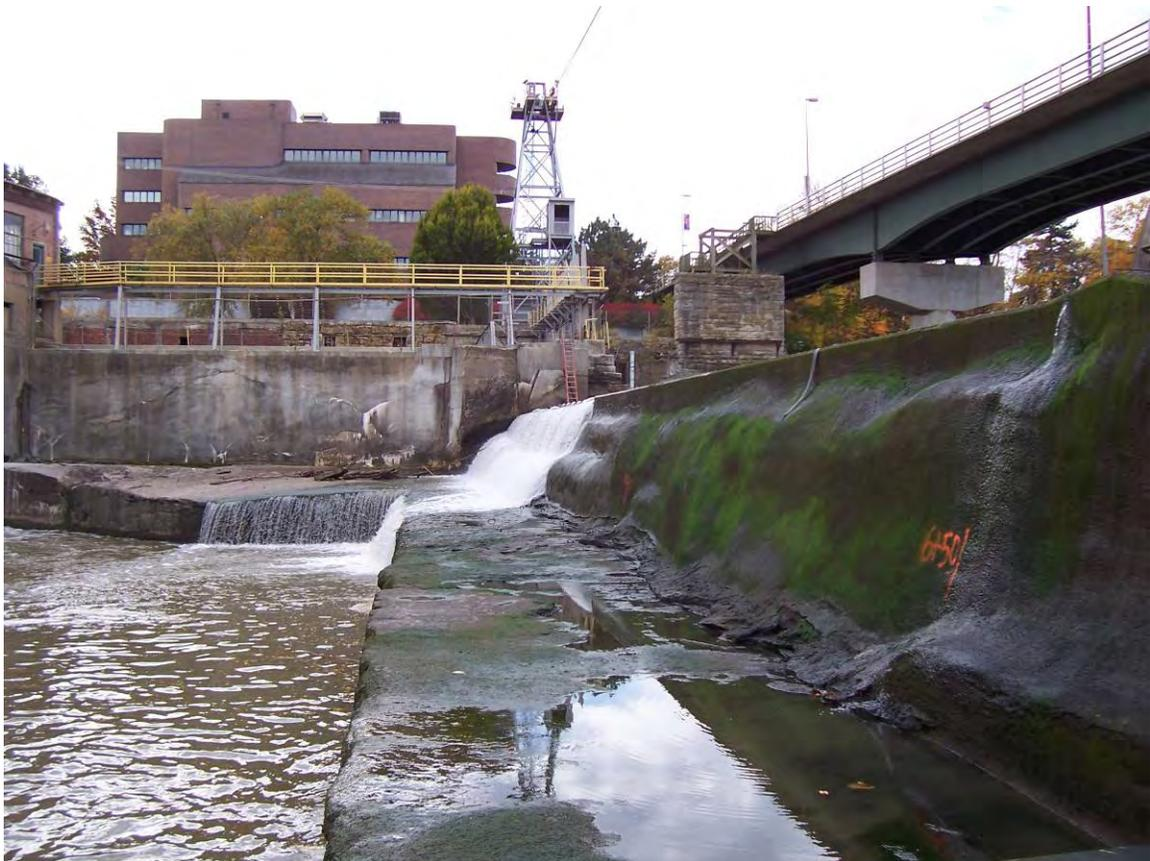
83. Sta 6+50 to south pneumatic flashboards. Eroded shotcrete.
