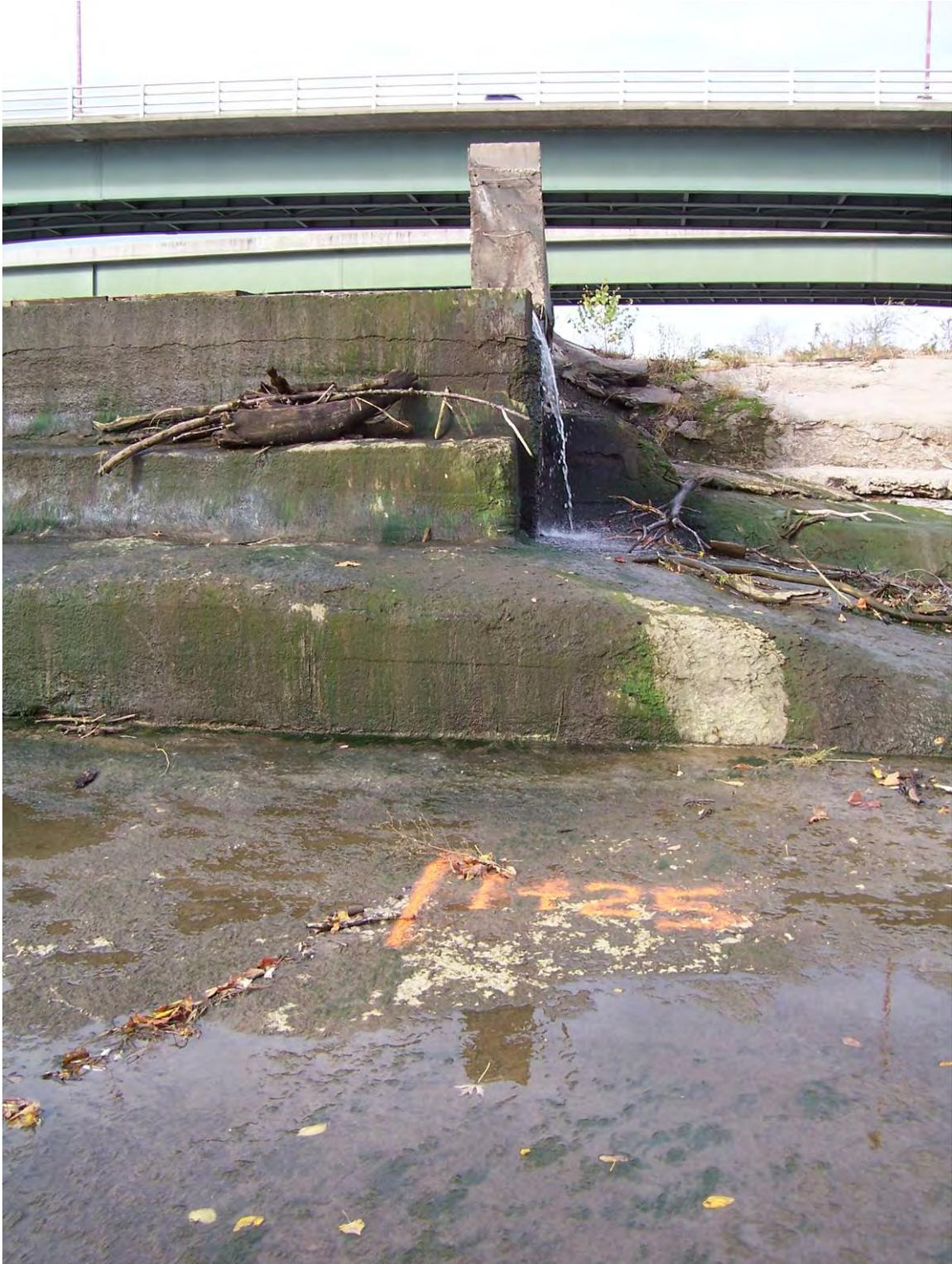
18. Sta 1+25. Eroded concrete at north end of dam. Exposed joints at bottom of dam steps. Eroded shotcrete near top of dam.
