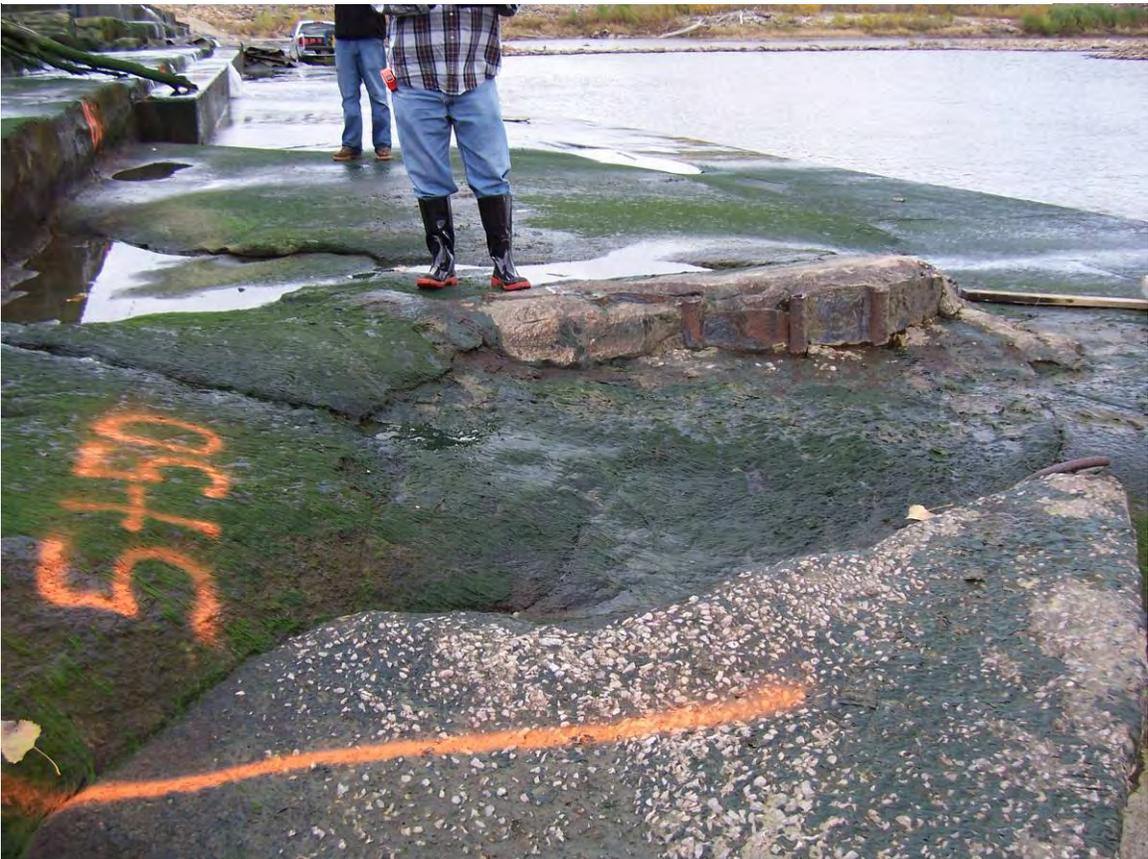
70. Sta 5+50. South end of steps. Exposed old sheet piling encased in apron. Eroded concrete with numerous exposed joints.
