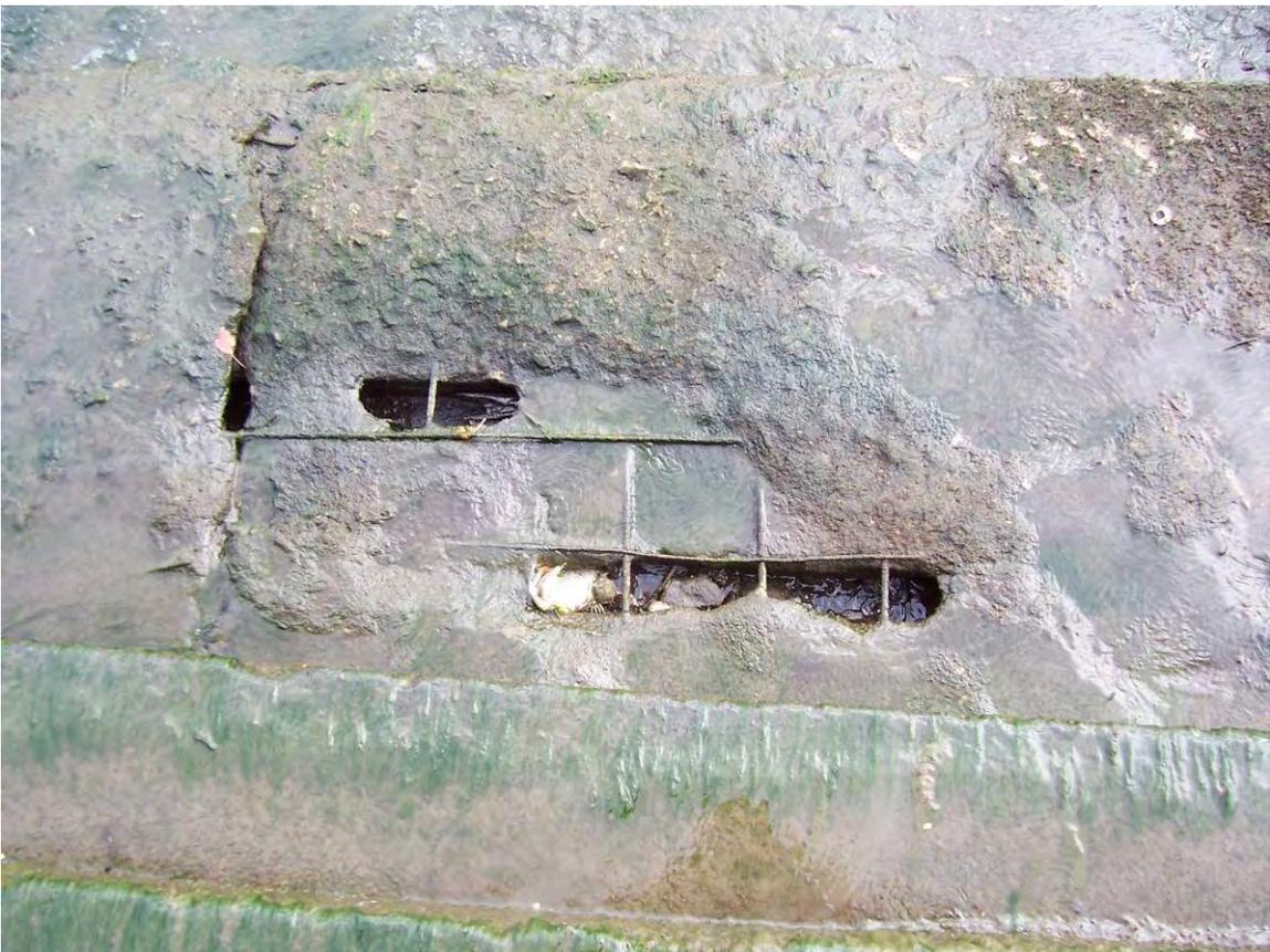
99. Sta 3+90±. Eroded concrete with exposed wire mesh in top step.
