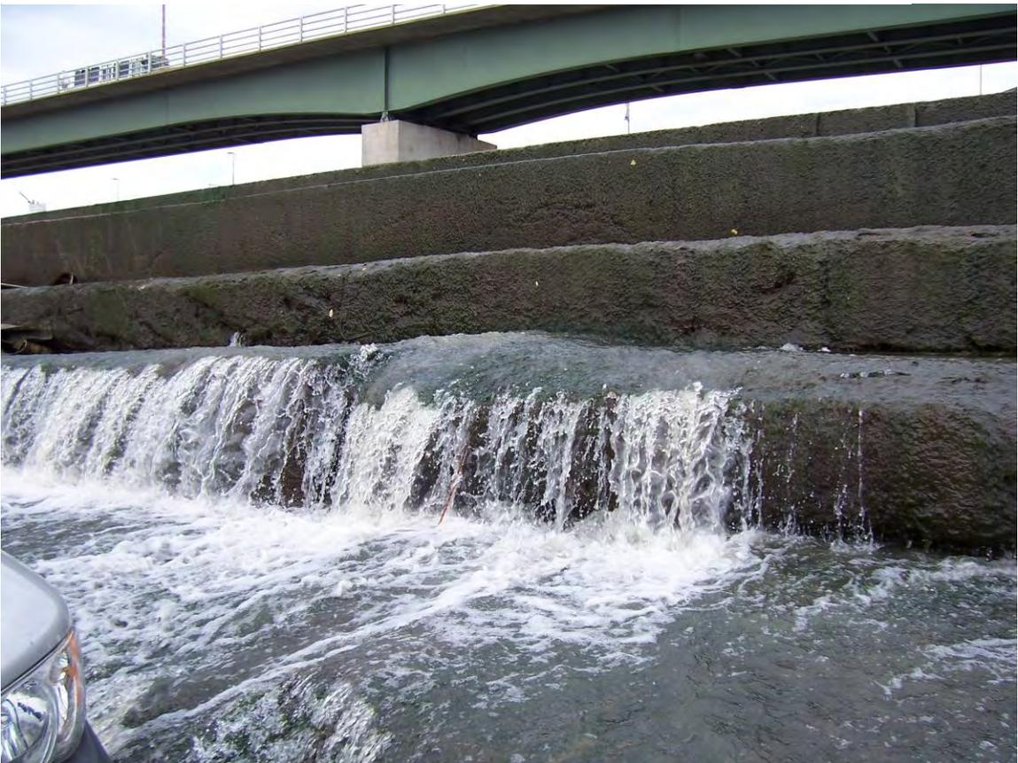
53. Sta 3+80±. Significant flow through Dam in numerous locations.
