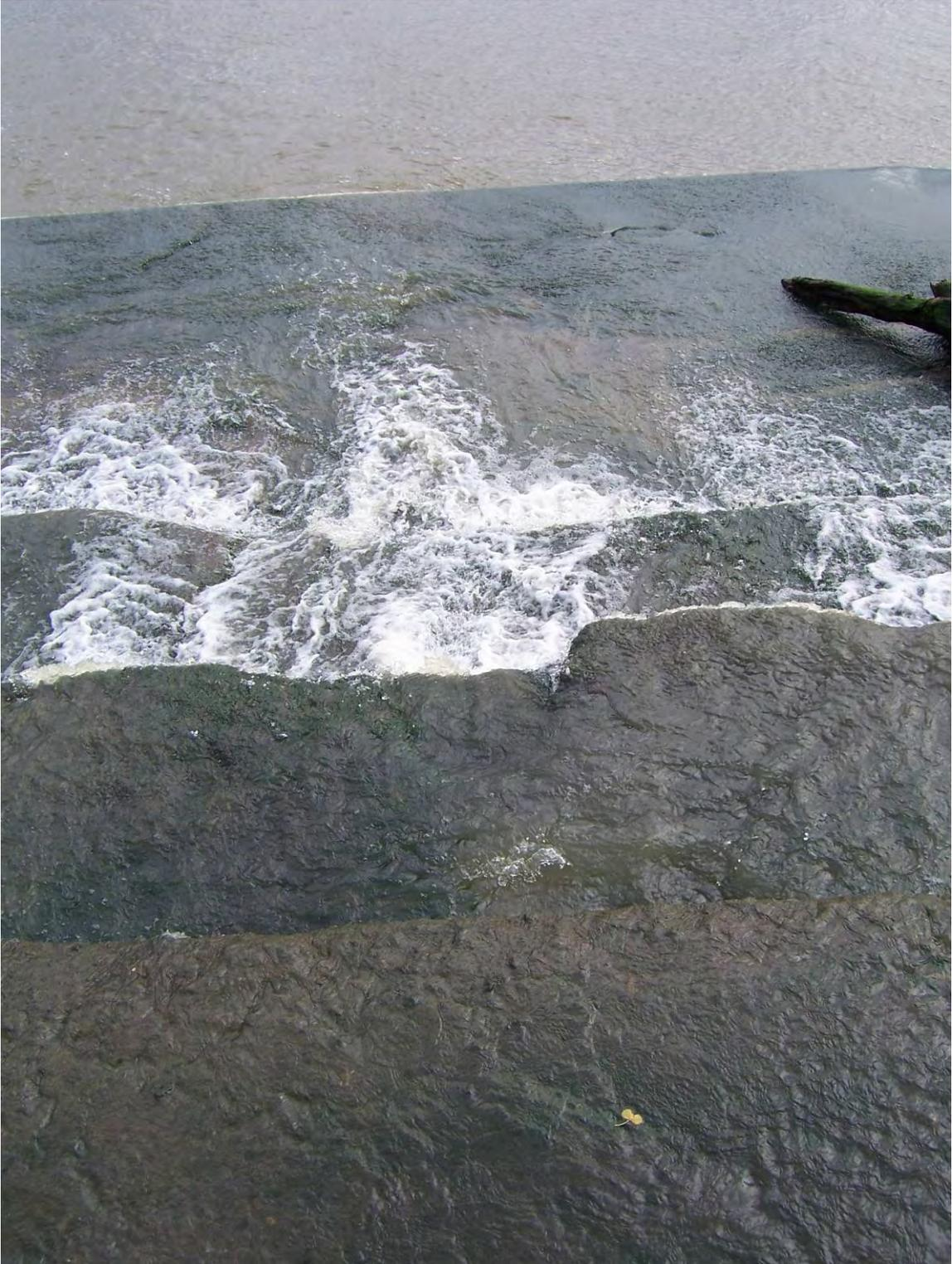
100. Sta 3+80± from top. Severe flow through dam.
