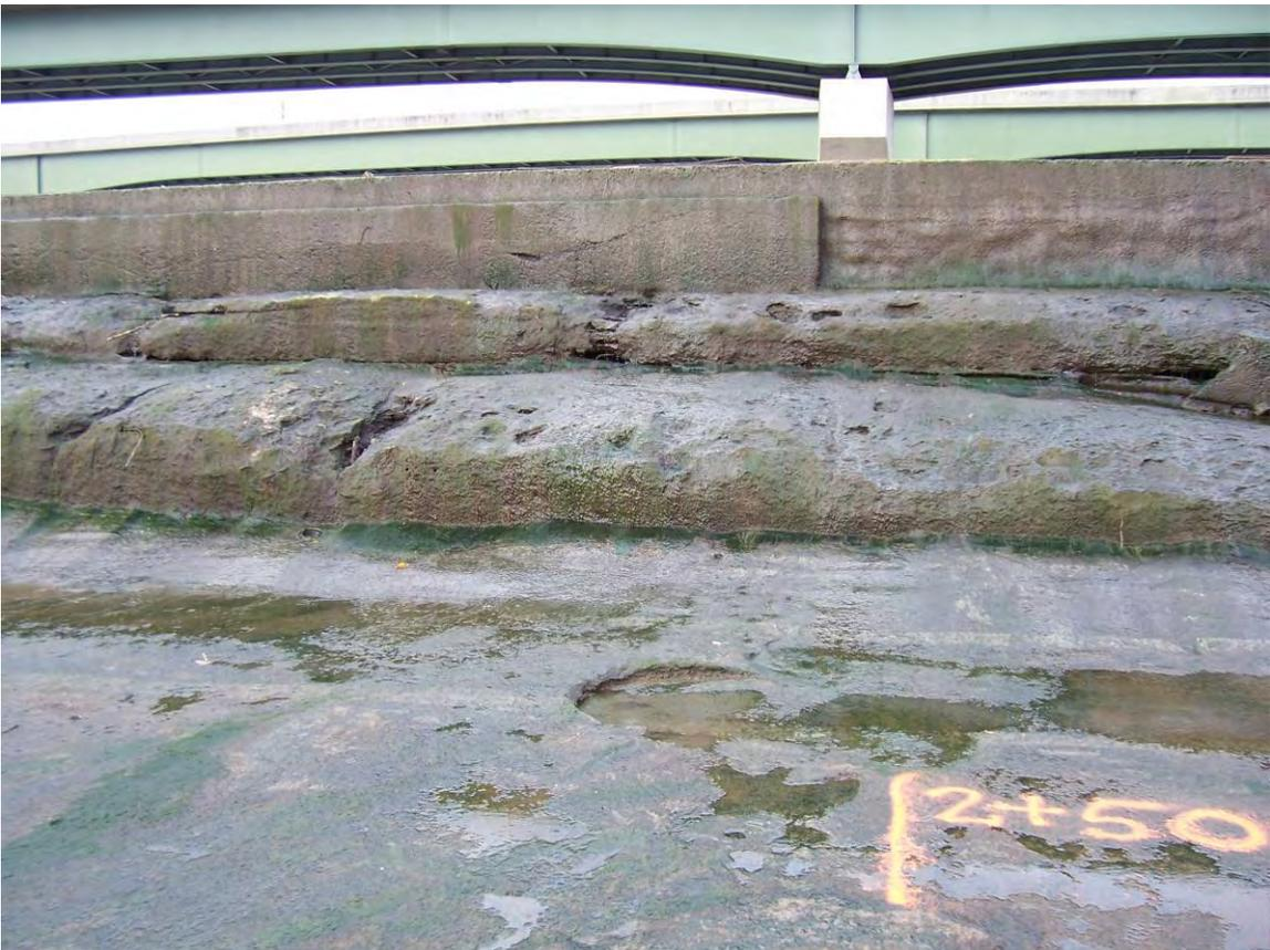
31. Sta 2+65. Eroded, disintegrated timber holes with exposed rebar. Eroded concrete on apron.
