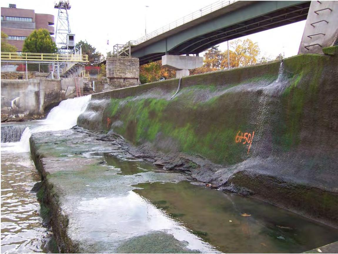
80. Sta6+50 to sour pneumatic flashboards. Eroded Shotcrete
