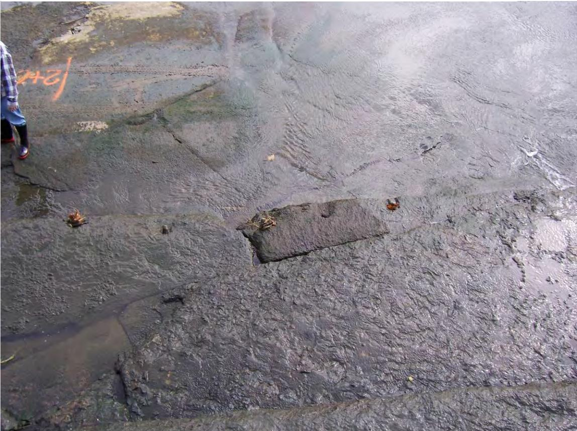
107. Sta 2+10 from top. Separated triangular section in bottom step.
