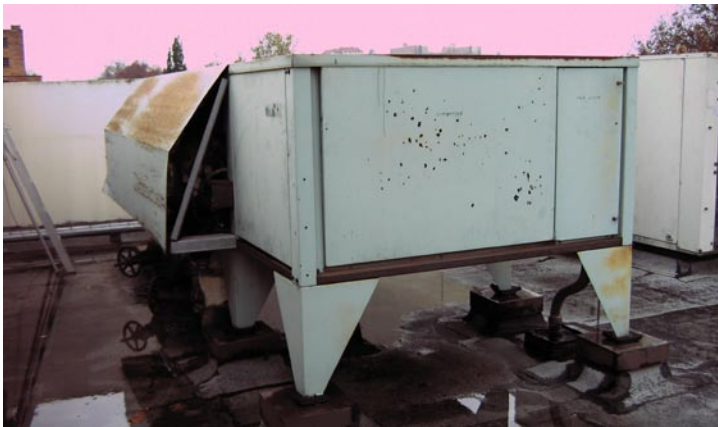
The existing 1972 chiller and its related pump that need to be replaced for improved efficiency and because of age and condition.
