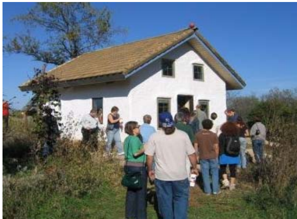
(on left) Tour guests wait their turn to walk through the O'Brien cottage, a smaller structure on the tour, featuring timber frame construction, straw bale and straw light clay walls and adobe floors.
