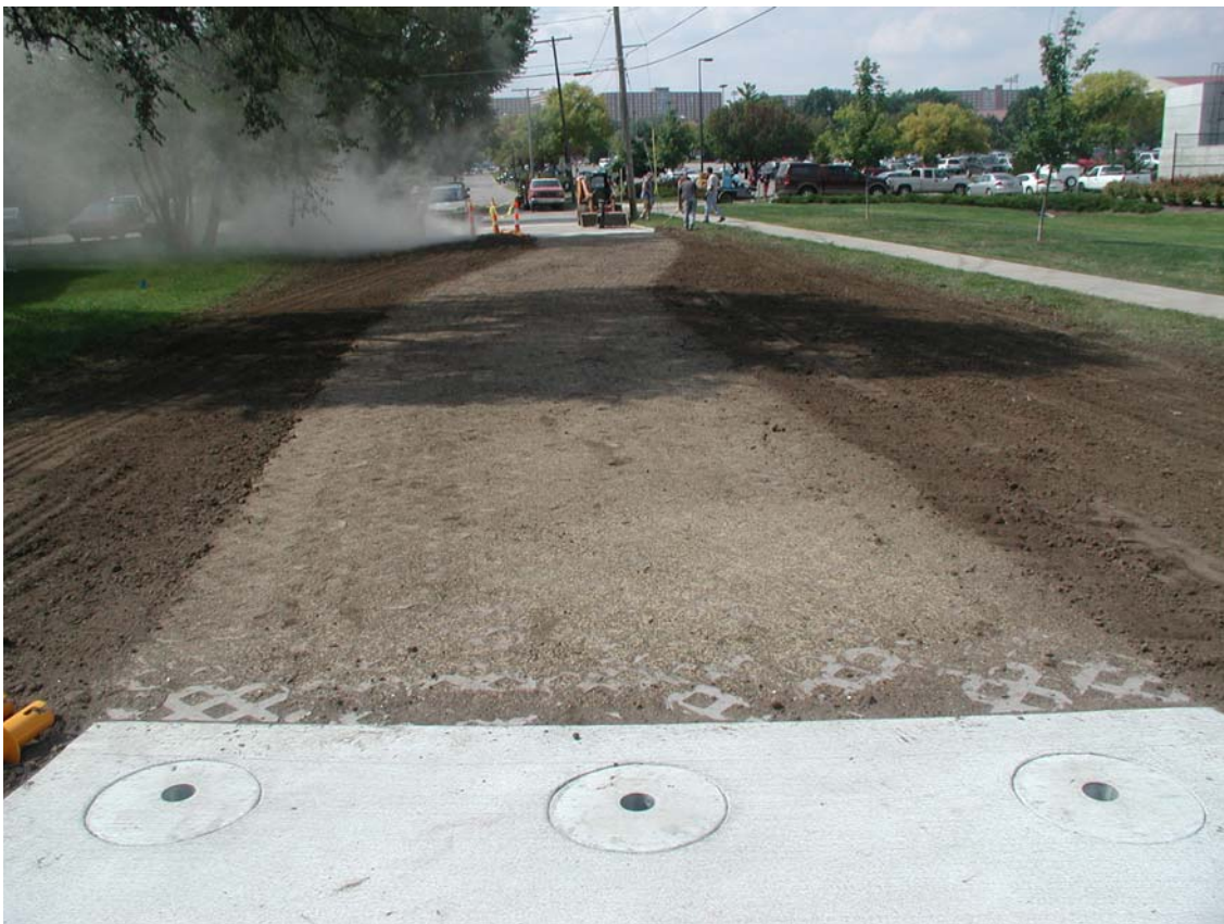
A look at the path of grass pavers before seeding (looking west).
