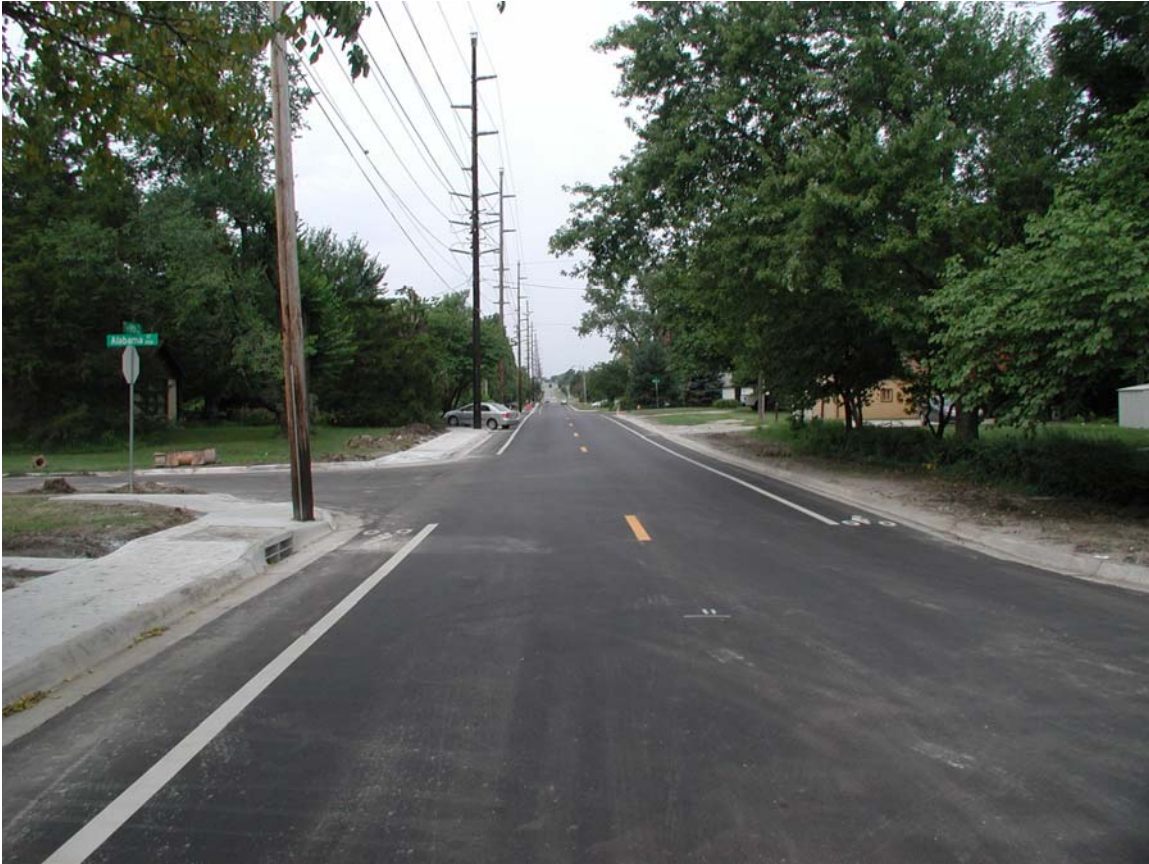
19 th & Alabama St. – Mill and overlay section with new curb and gutter and bike lanes (looking west).
